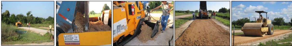
Figure 2.6. Placement of Base Material at Riverside Campus.
