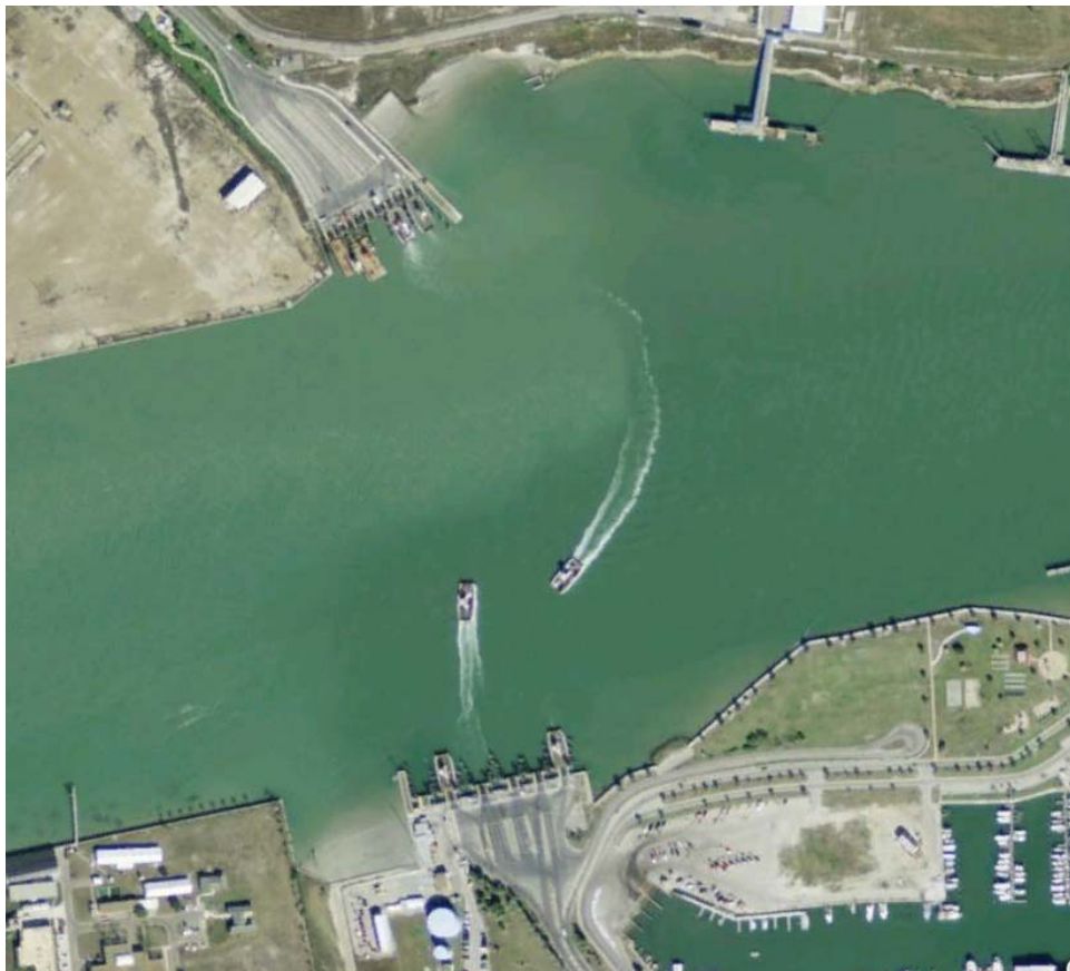
Figure 4. Port Aransas Ferry/SH 361 at Corpus Christi Channel.
