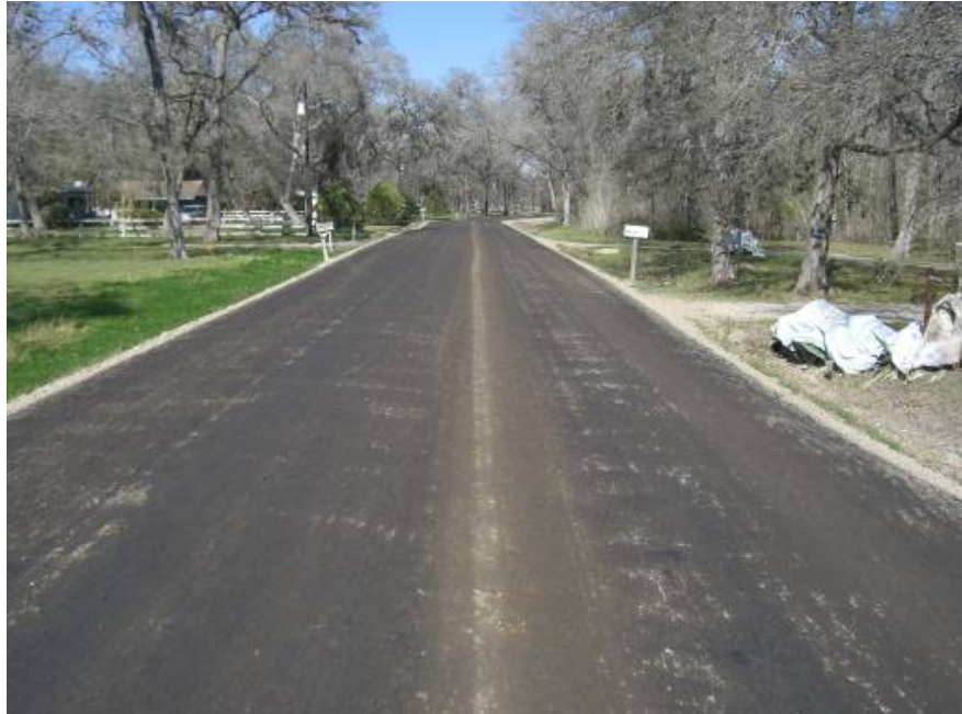
Figure 94. Greenbriar County Road, Primed with MC-30 (1).
