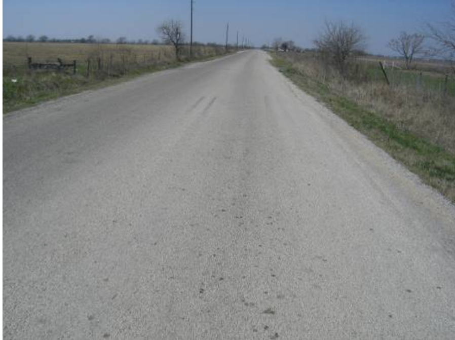
Figure 96. County Road to Saltwater Disposal Facility (1).
