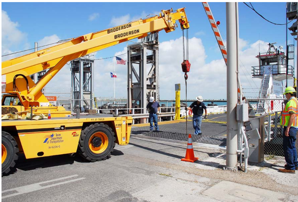
Figure 31. Photograph of Deck Panel Being Removed at End of Ramp.
