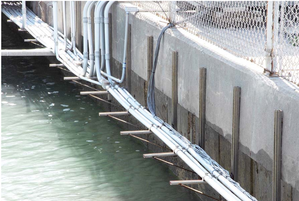
Figure 39. Photograph Showing Cable Bundle Entering Out-Building.
