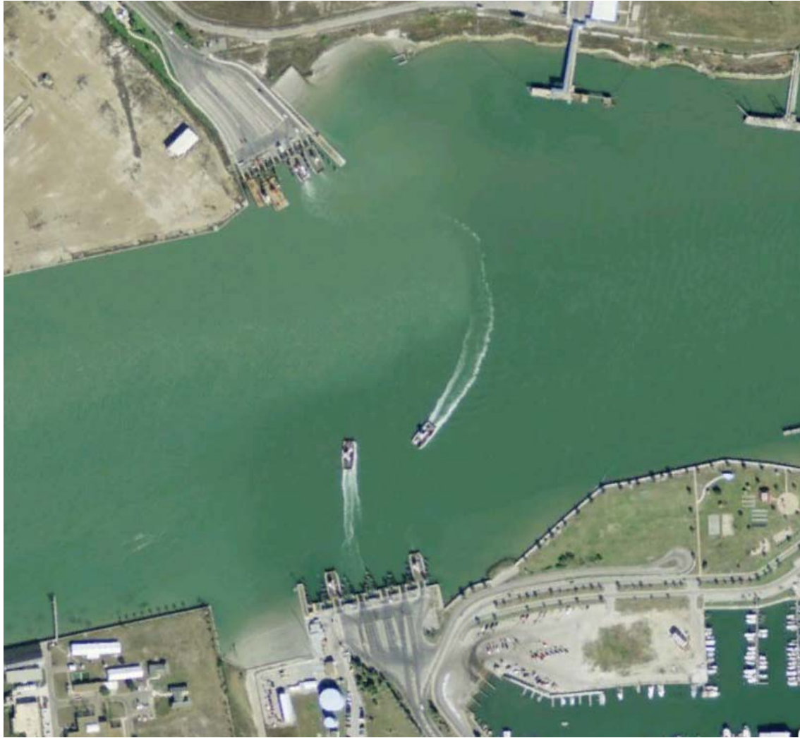
Figure 54. Port Aransas Ferry/SH 361 at Corpus Christi Channel. (Source: Google™ Earth; accessed 8/19/2010)
