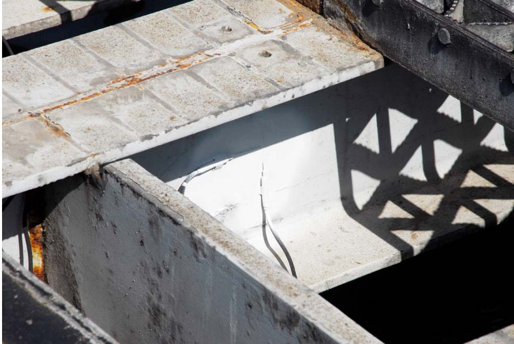
Figure 36. Photograph of Sensor Installation after Priming and Painting.
