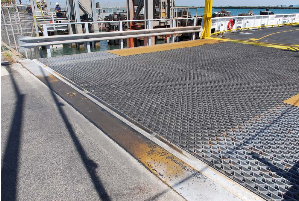
Figure 42. Photograph of Ramp at Completion of Sensor Installation.
