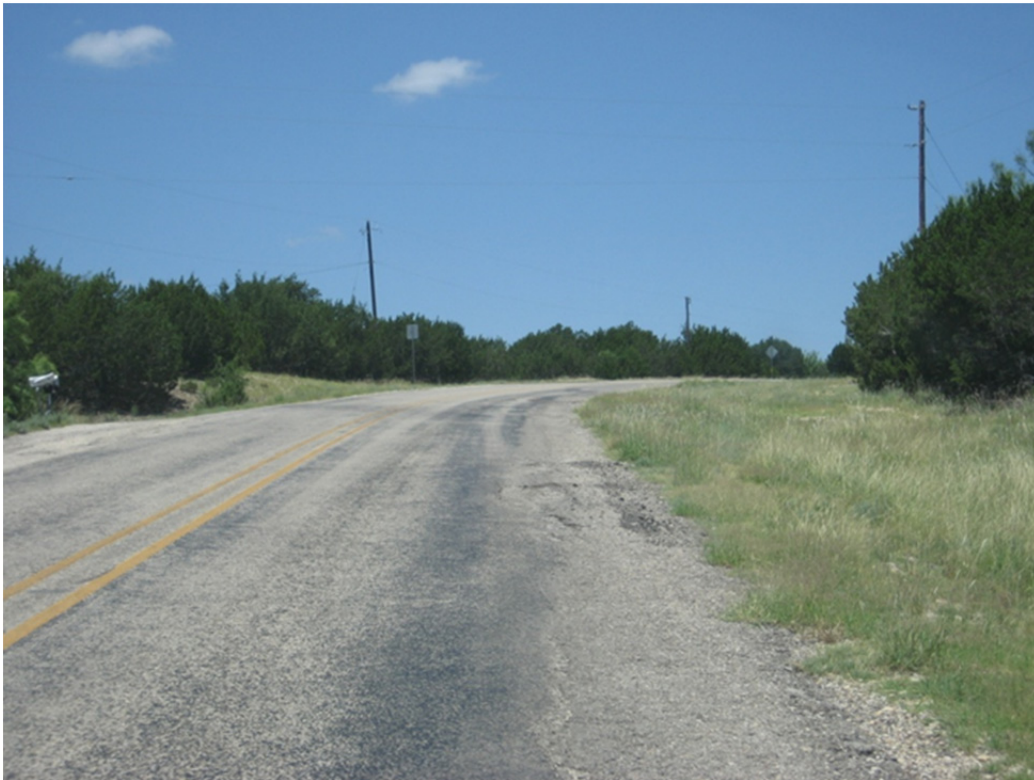
Figure 27. Edge Repairs (FM 89, Abilene District).
