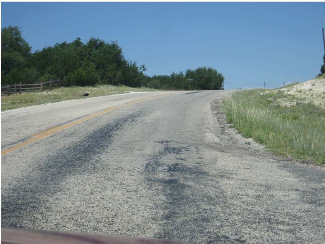
Figure 29. Patching and Flushing (FM 89, Abilene District).
