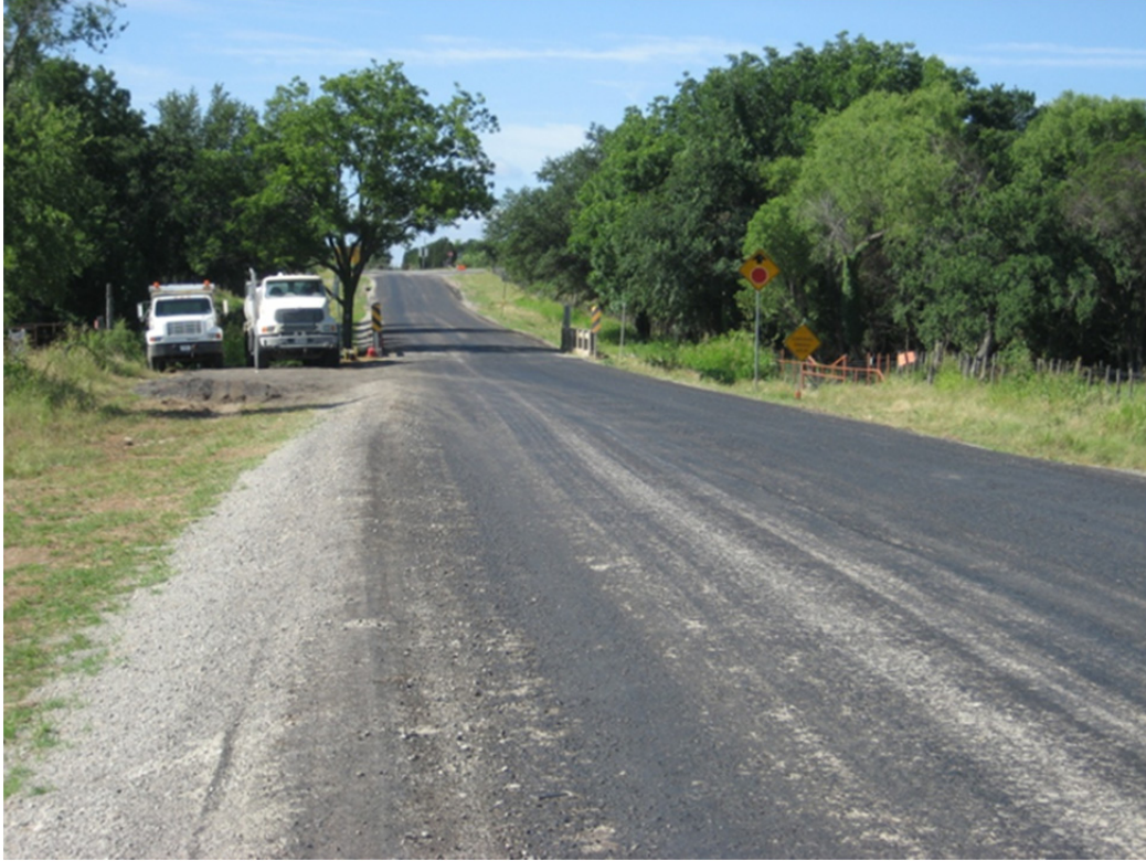
Figure 38. Full-Depth Reclamation (FM 52, Fort Worth District).
