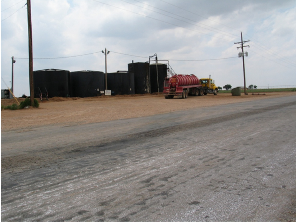
Figure 20. Well Fluid Station (FM 1585, Lubbock District).
