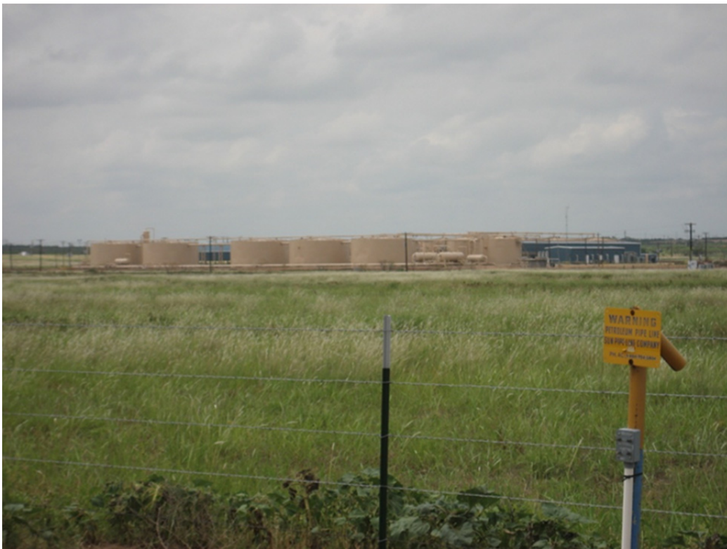
Figure 33. Gas Plant (FM 1611, Abilene District).
