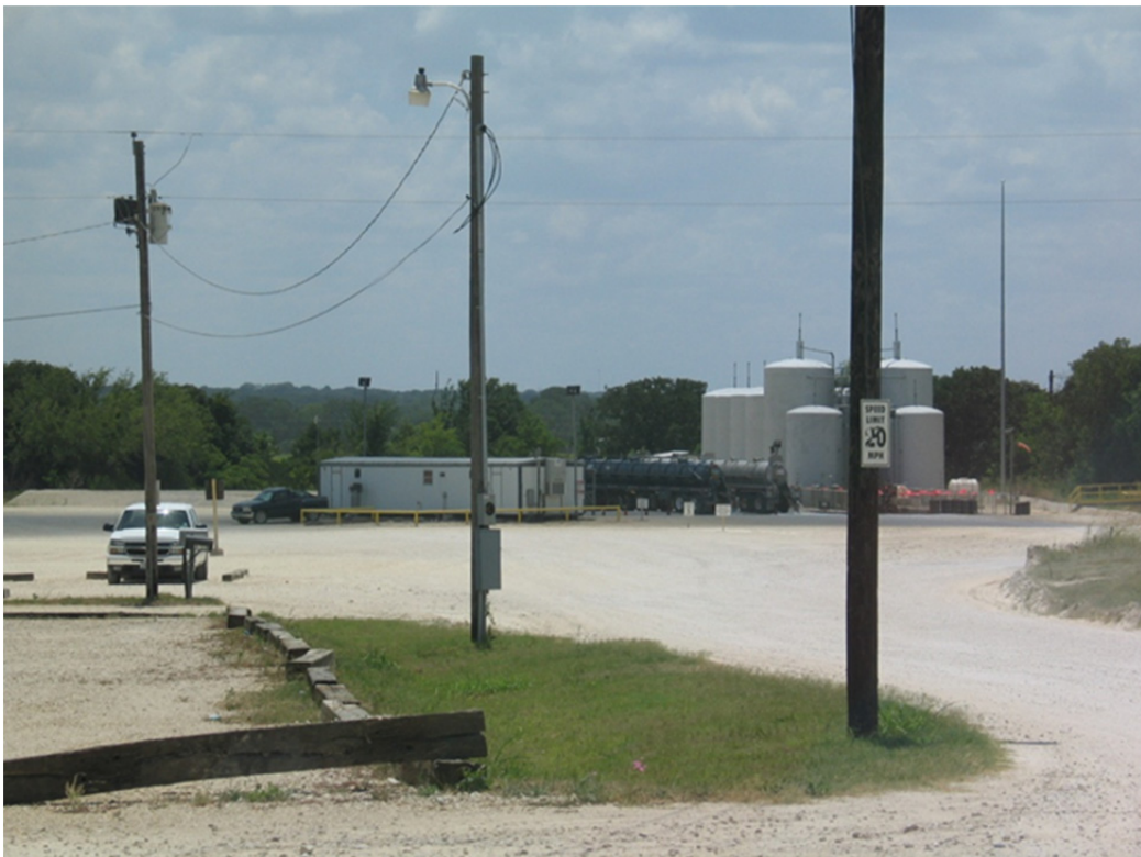
Figure 49. Saltwater Disposal Facility (IH 35W – Frontage, Fort Worth District).
