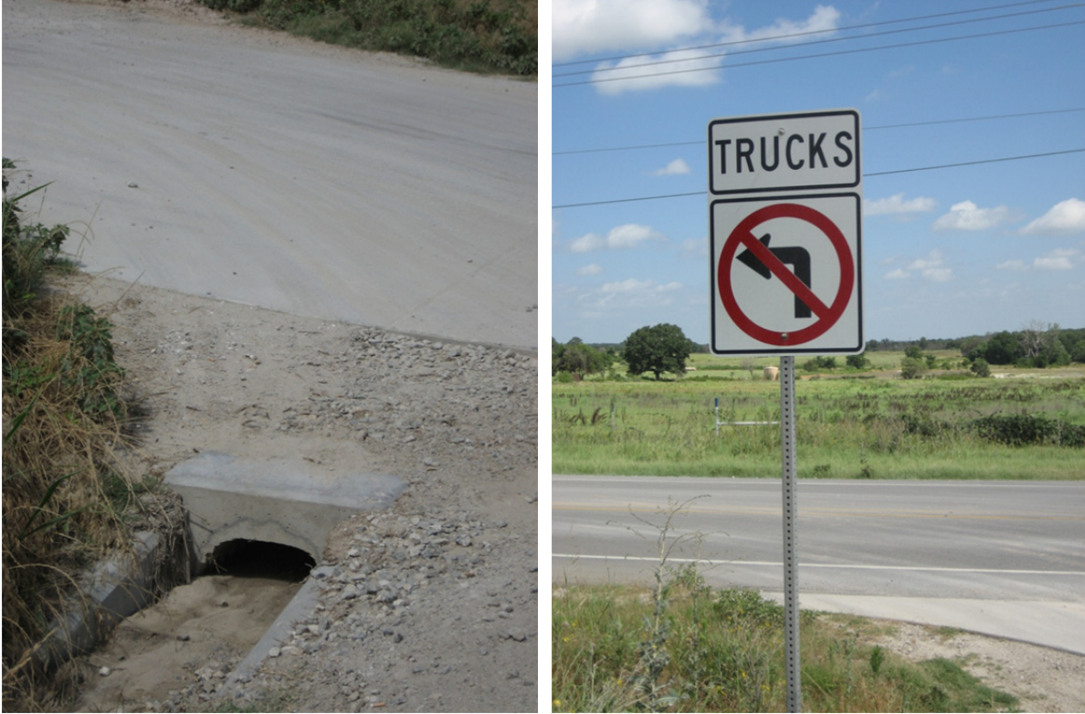
Figure 40. Saltwater Disposal Facility Exit Driveway (FM 2257, Fort Worth District).
