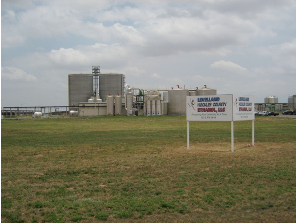
Figure 24. Ethanol Plant (FM 2646, Lubbock District).
