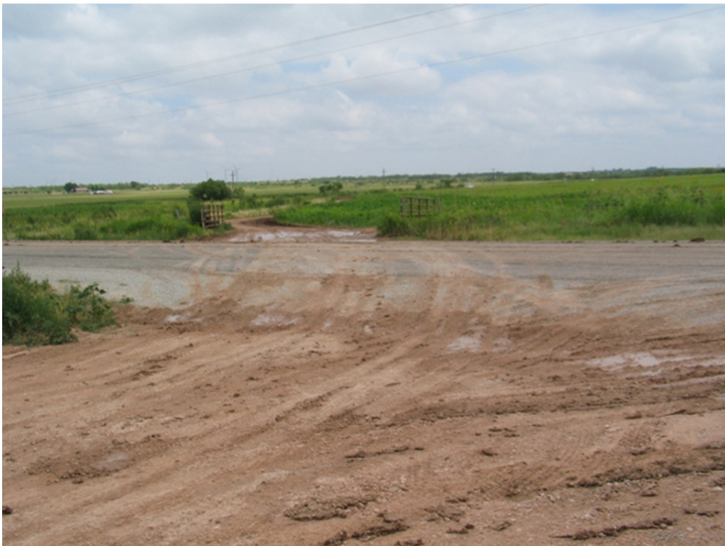
Figure 35. Mud Tracking (FM 1611, Abilene District).
