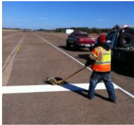
Figure 53. Stop Bar Installation.
