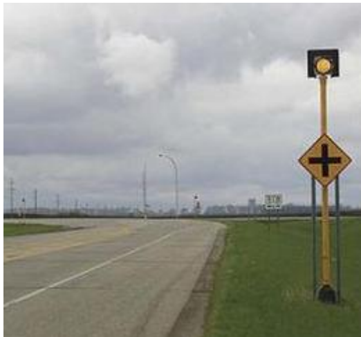
Figure 14. Examples of Replacement Beacons for Overhead Flashing Beacons.
