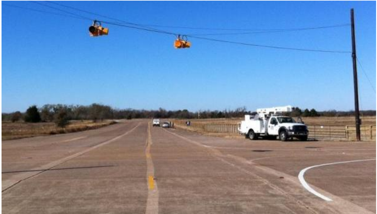
Figure 55. Overhead Beacon (Amber Beacons) Viewed from Taxiway 7 (Facing West).
