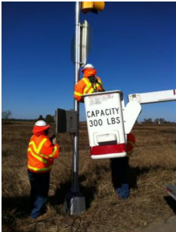
Figure 56. Installation of Stop and Warning Signs with Flashing Beacon Assemblies.
