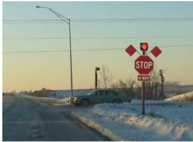
Figure 14. Examples of Replacement Beacons for Overhead Flashing Beacons.
