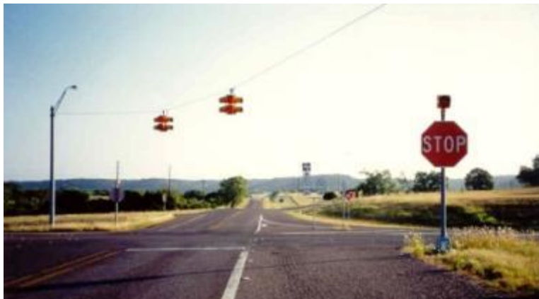
Figure 6. Use of Stop Bar at a Rural Intersection.
