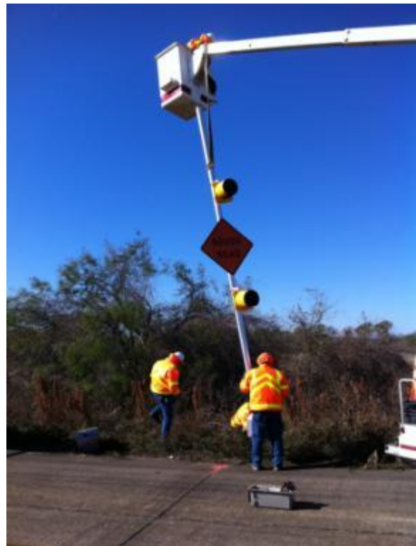
Figure 56. Installation of Stop and Warning Signs with Flashing Beacon Assemblies.
