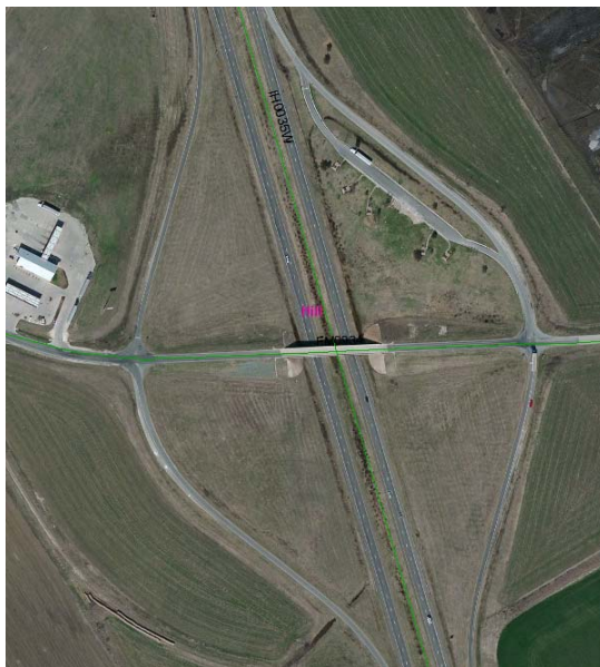
a) Bridge on IH 35W main lanes (Hill County)
