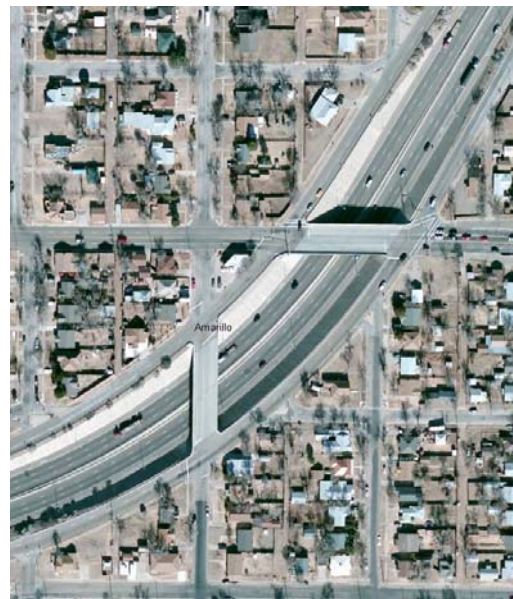
b) Bridges on IH 27 main lanes (Amarillo)
