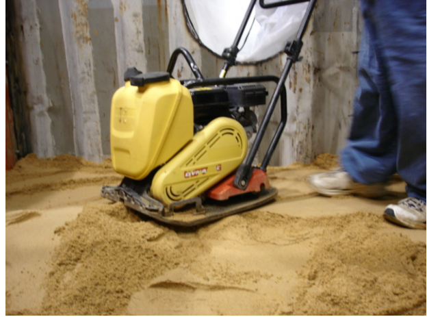
Step 2. Compact sand lift.
