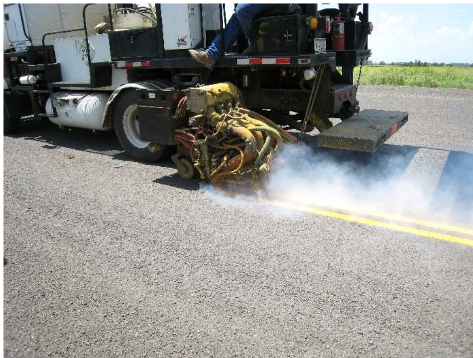
Figure 24. SH 21 Lead-Free Thermoplastic Installation.
