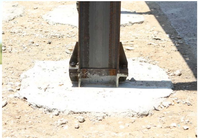
Figure 7.25. TxDOT W8×18 – 16-ft × 10-ft Large Sign Support before Test No. 463630-2.
