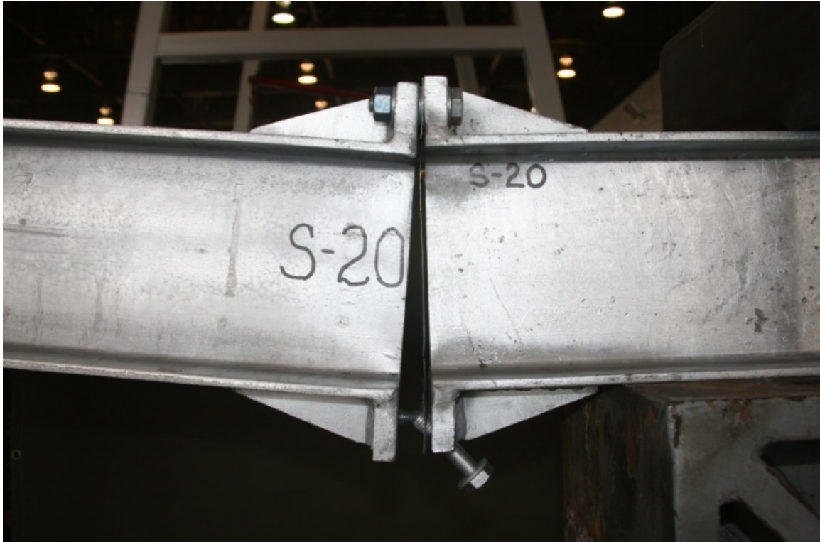
Figure C7. Test Sample S20 after Slip Bolt Failure.
