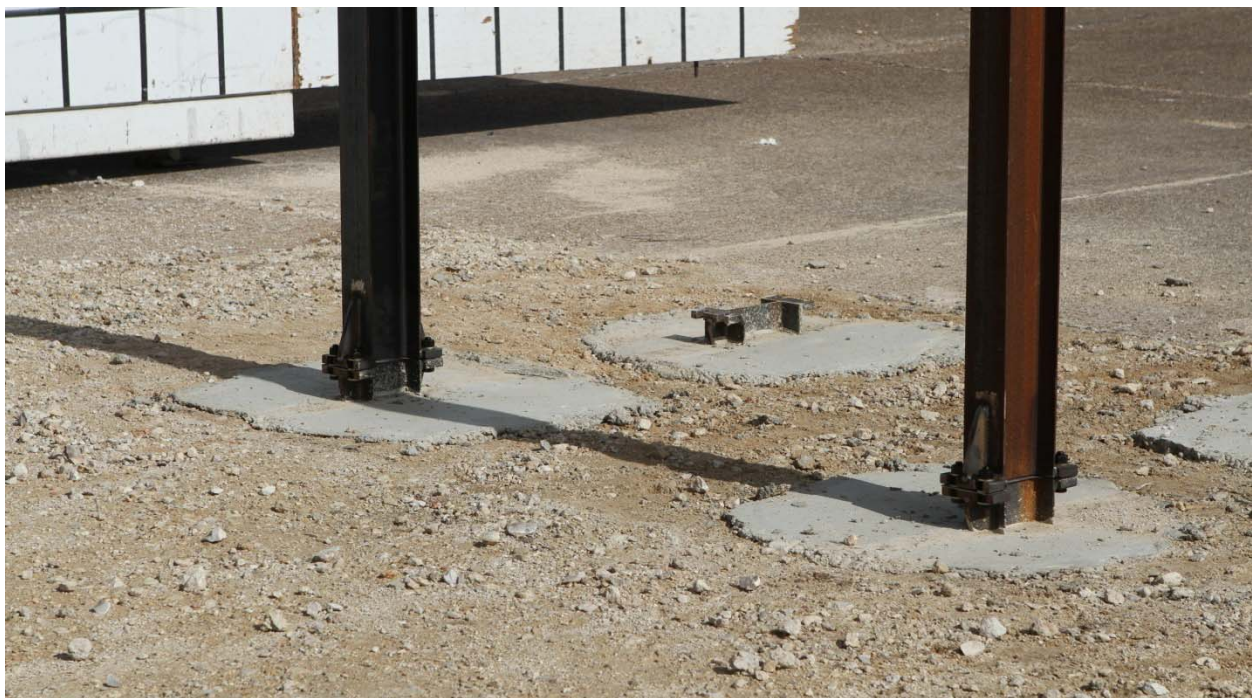
Figure 7.16. TxDOT W6×9 – 4-ft × 10-ft Large Sign Support before Test No. 463630-1.
