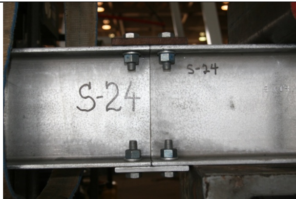
(b) Fuse Plate Connection Before Loading (No Gap)
