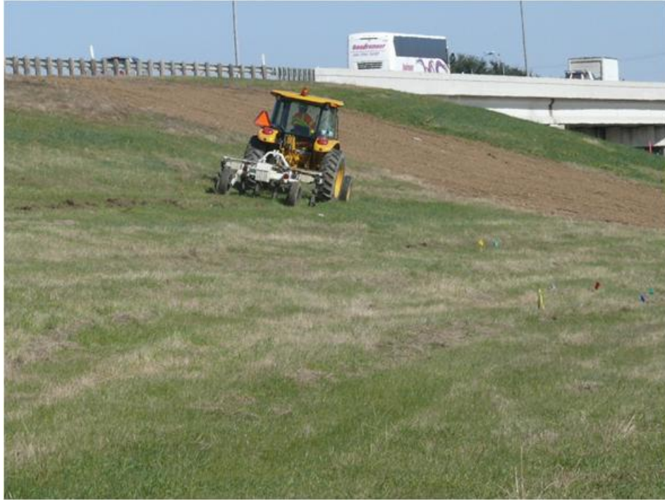
Figure 5a.11. Grapevine Site 2 Showing Embankment with Steep Slope that Prevented Collecting Soil Samples Using the Drilling Rig from Some Areas.
