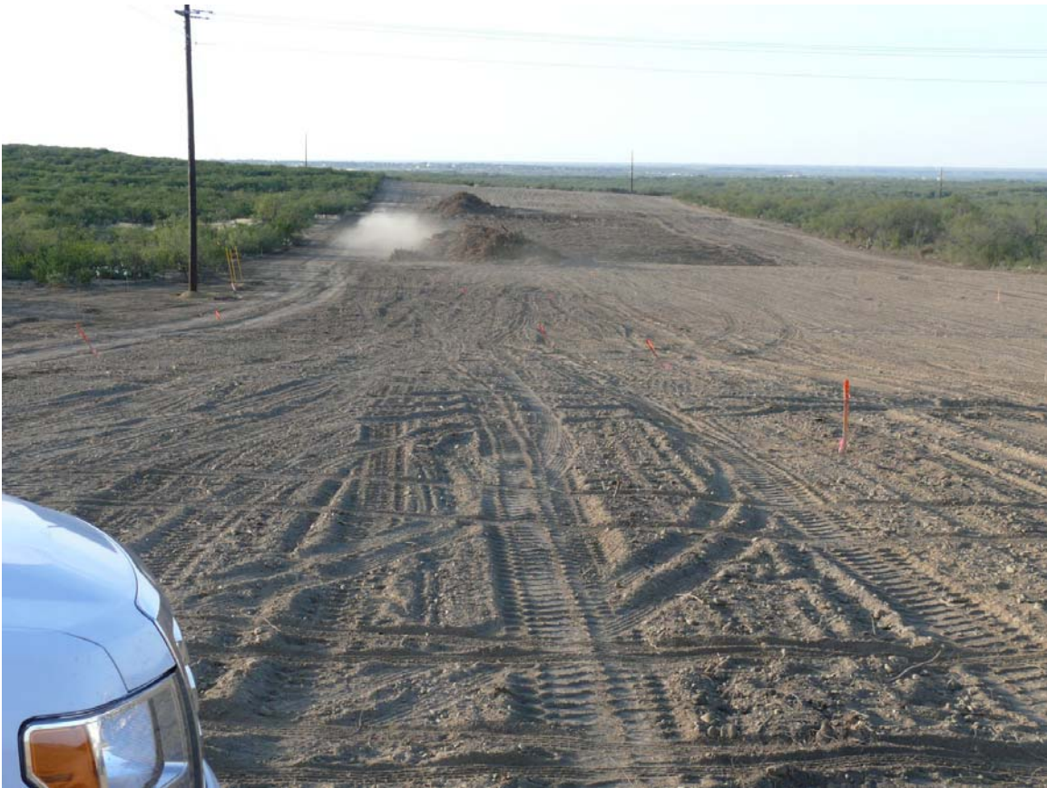
Figure 5a.3. New Construction Site in Eagle Pass, Texas, Shows Dry Conditions.
