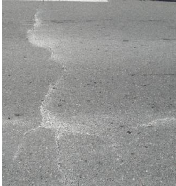
Figure 4.5. Block Cracking.
