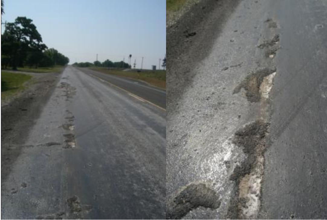
Figure 3.21. Debonded Surface Treatment (FM 2154).
