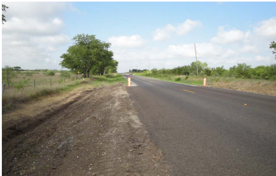
Figure 2.21. Partially Completed FM 148 Verification Testing of First 1.1 Mile.
