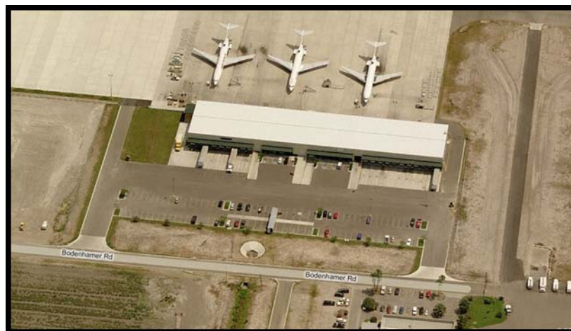
Figure 27. Freight Facility with Space for Truck Backing Maneuvers.
