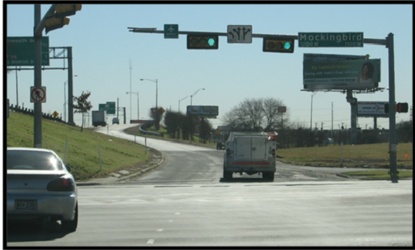
Figure 15. Placard Sign for Dallas Love Field on Southbound IH 35E Frontage Road.
