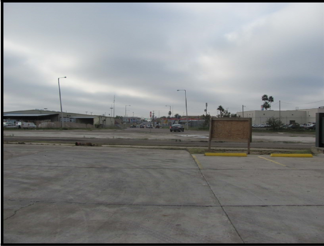
Figure 116. Laredo International Airport—Bustamante Street and Arkansas Avenue from Cargo Area.
