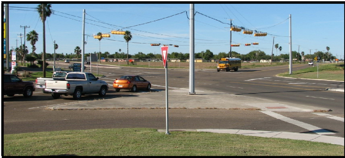
Figure 133. Skewed Intersection—SL 499 at FM 507/North 25th Street.
