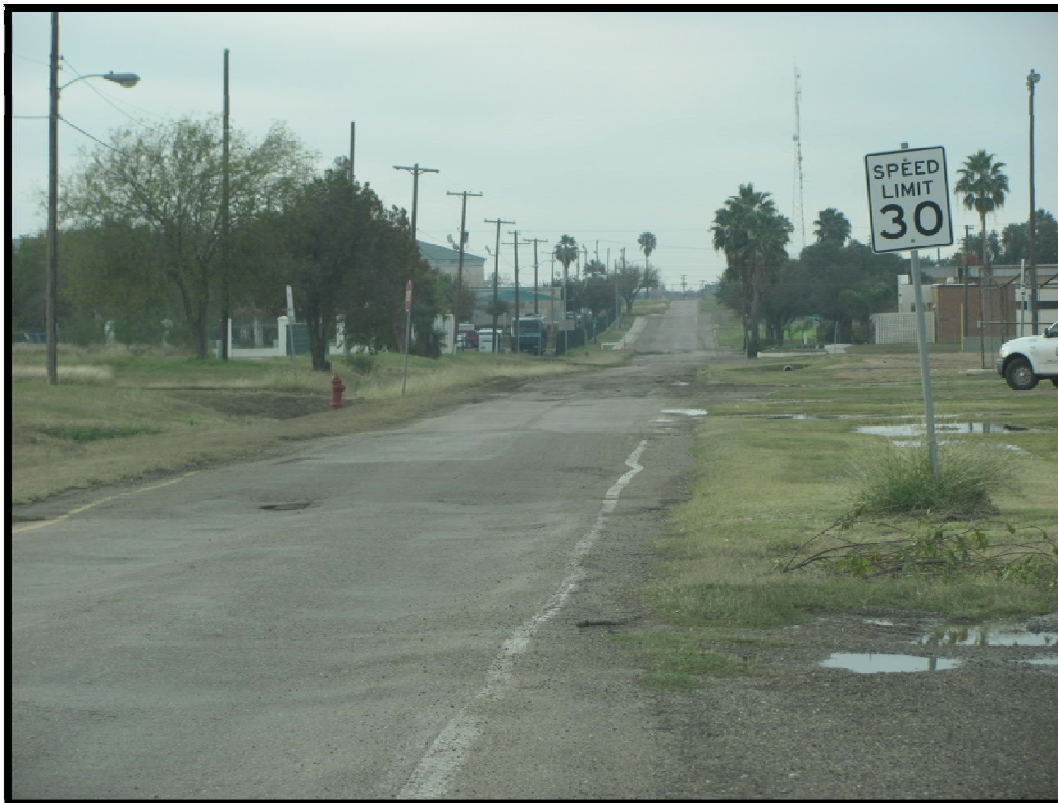
Figure 113. Laredo International Airport—Thomas Avenue.
