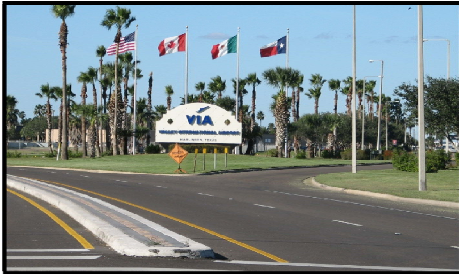
Figure 126. Gateway Entrance to Valley International Airport.
