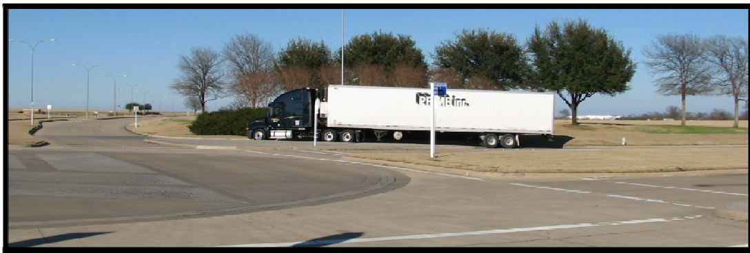
Figure 92. Turning Radius to Accommodate Large Trucks—Intersection of Alliance Boulevard at Heritage Parkway.
