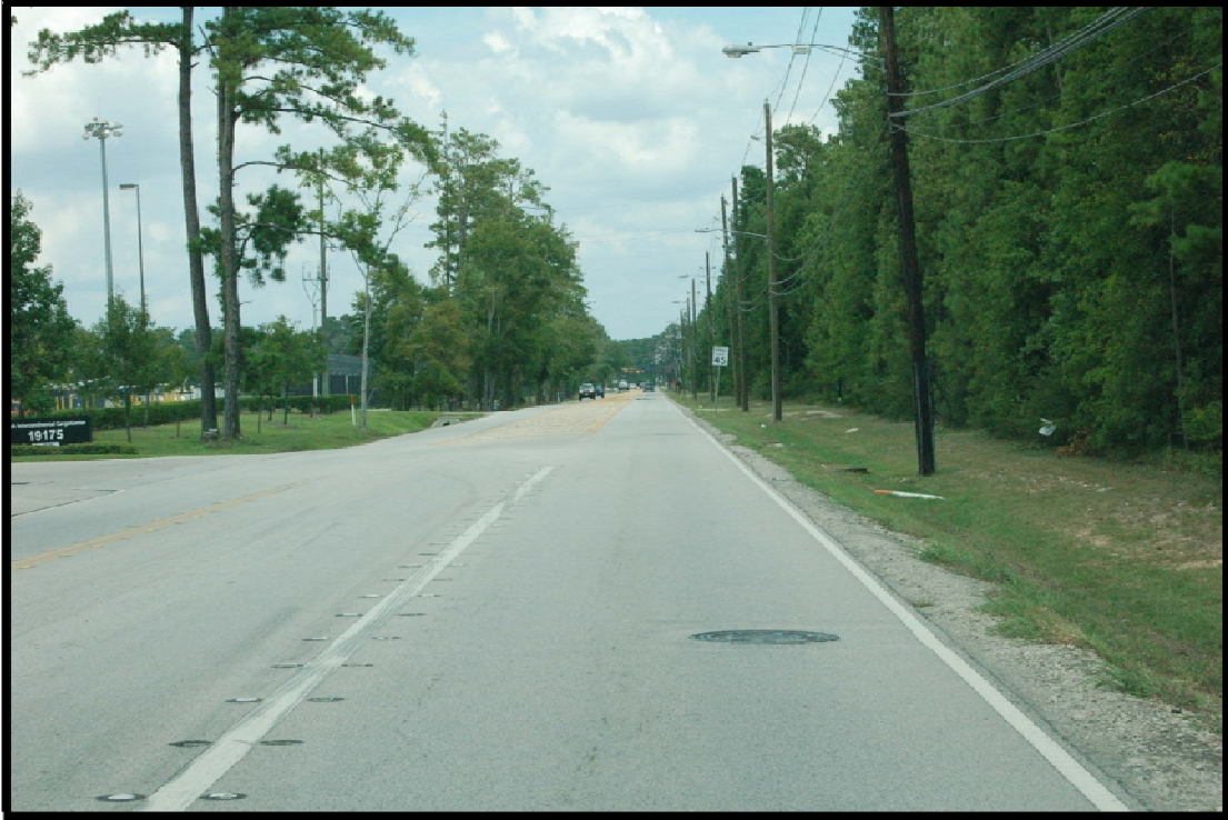
Figure 70. George Bush Intercontinental Airport—North Lee Road.
