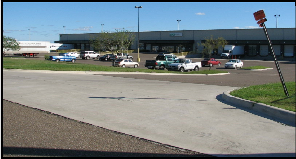
Figure 130. Freight Facility in the East Air Cargo Area at Valley International Airport.
