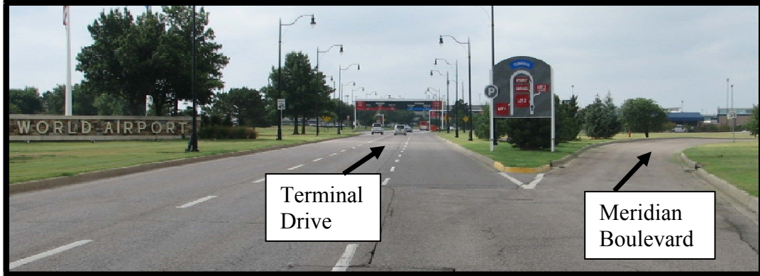
Figure 82. Southbound Airport Road Veers off from Meridian Boulevard.
