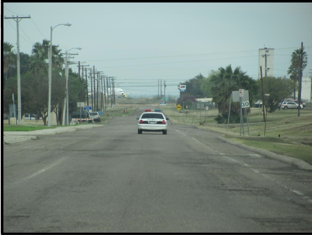
Figure 112. Laredo International Airport—Maher Avenue.
