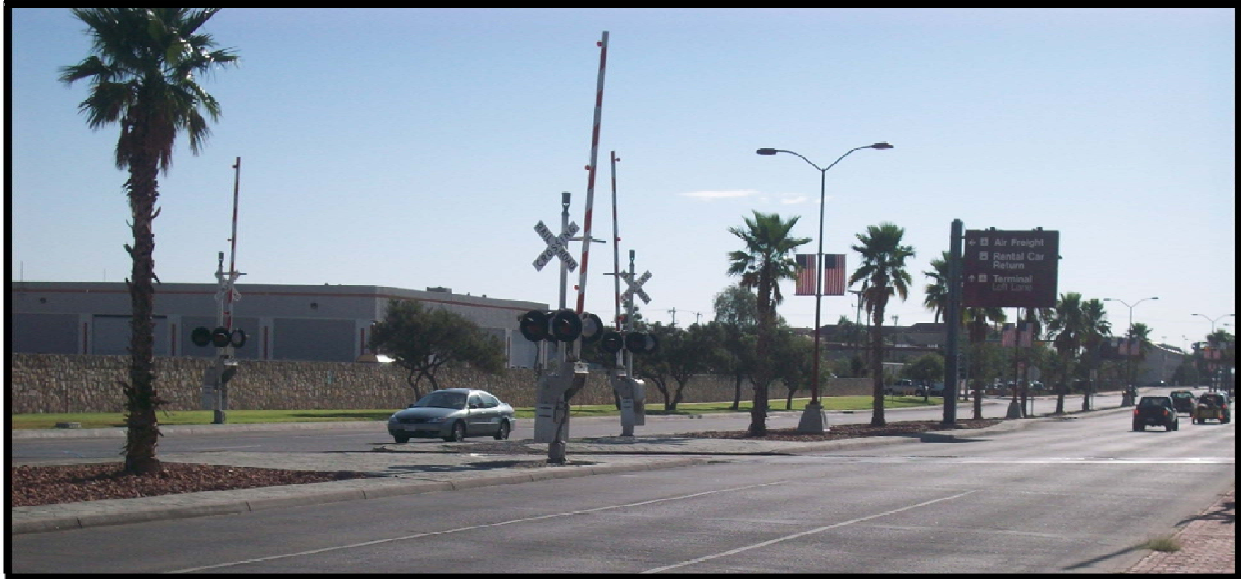
Figure 57. El Paso International Airport Air-Cargo Guide Sign—Airway Boulevard Eastbound.
