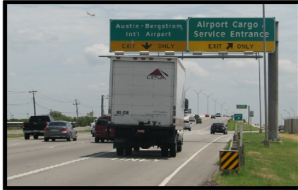
Figure 147. Separate Freight Exit at Austin-Bergstrom International Airport from SH 71.
