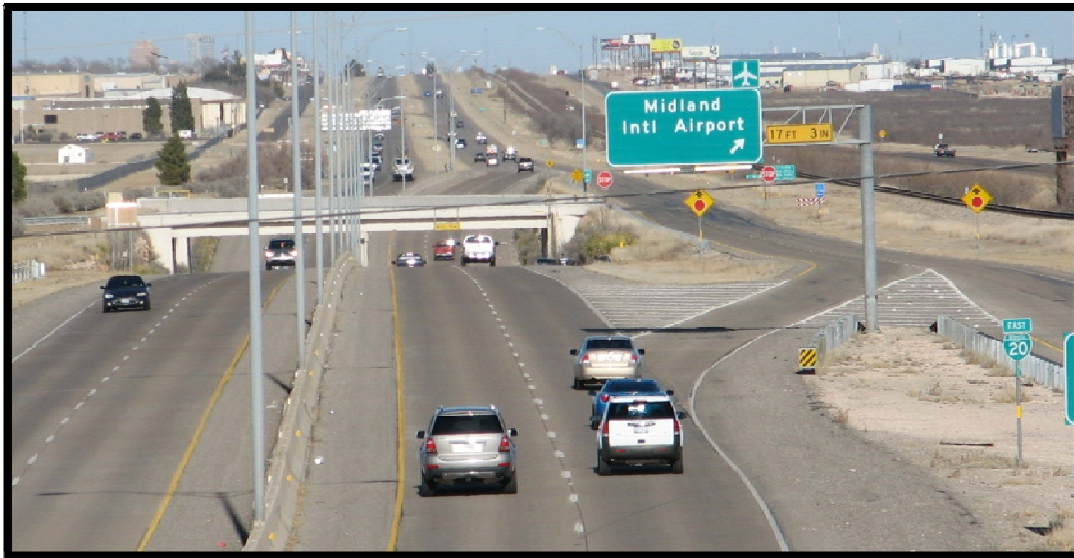
Figure 139. Exit for MAF from Eastbound BR 20.
