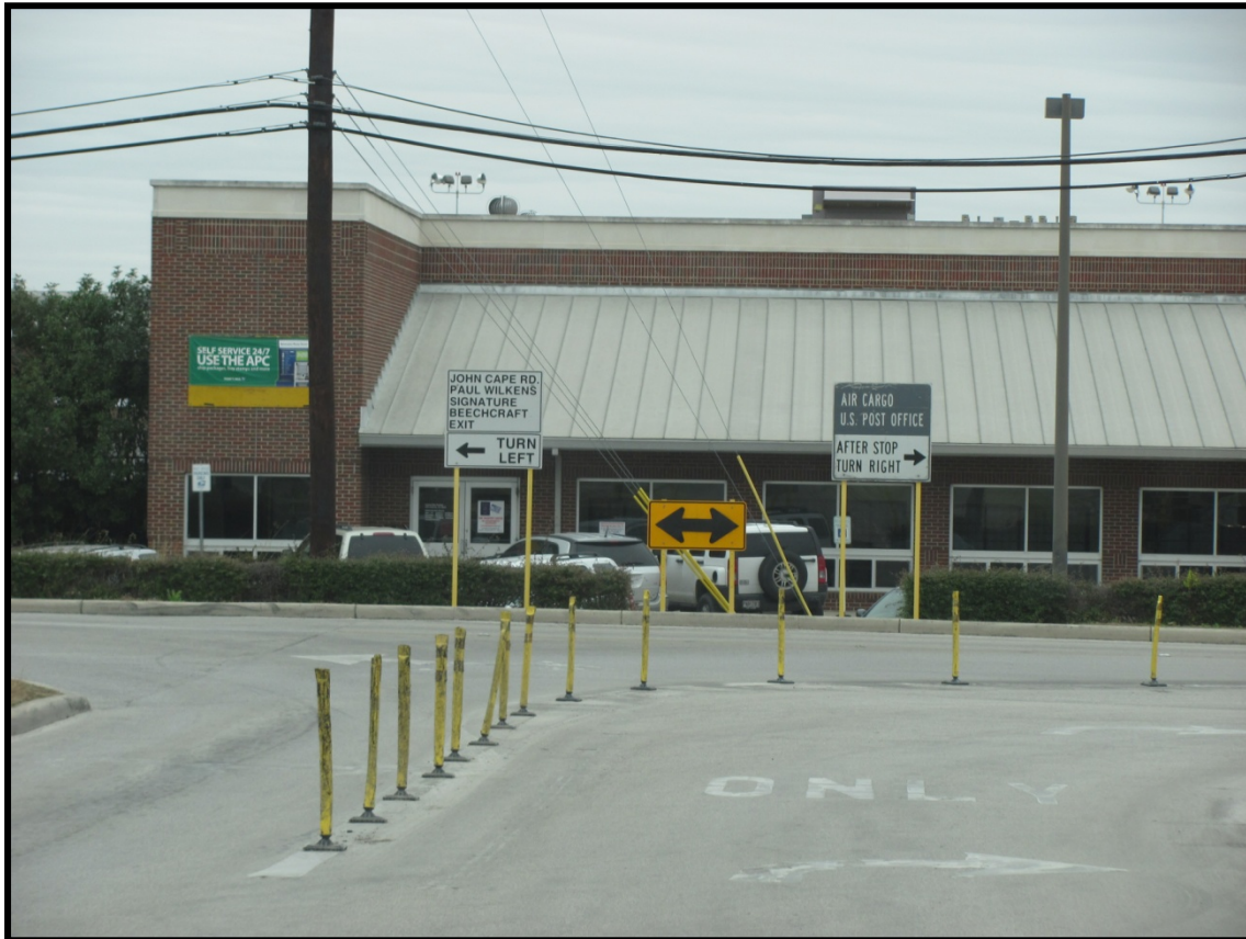
Figure 64. San Antonio International Airport—Signage/Turn Radii at Entrance to West Cargo Area.
