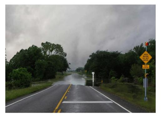
Figure 35. Illustration of How a Stop Bar Might Be Used as part of a Flood-Prone Crossing Treatment.
