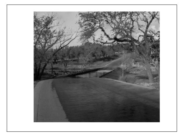
Figure 9. Roadway Scenario #2: Low-Volume Rural Road—Designed Low-Water Crossing.
