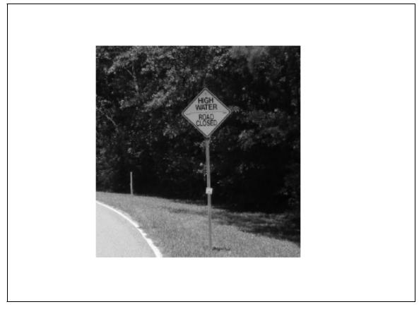
Figure 19. Example of Flip-Down Warning Sign to Alert Drivers to Flooded Roadway Conditions.
