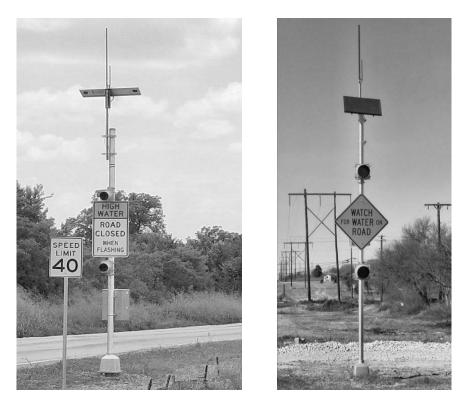
Figure 5. Example of an Advance Flood Warning System Produced by High Sierra Electronics (11).
