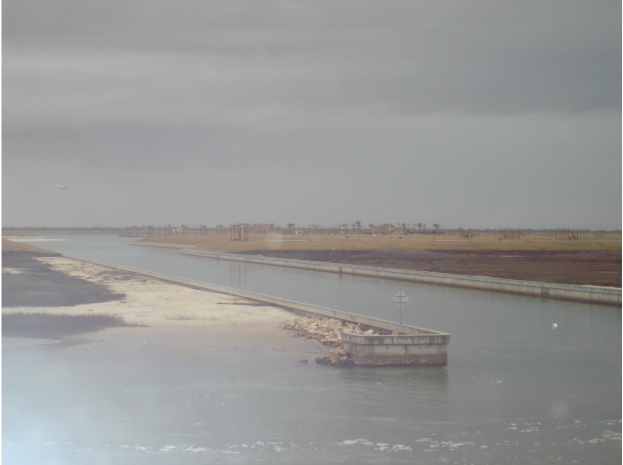
Figure 12. Canal Built into Land.
