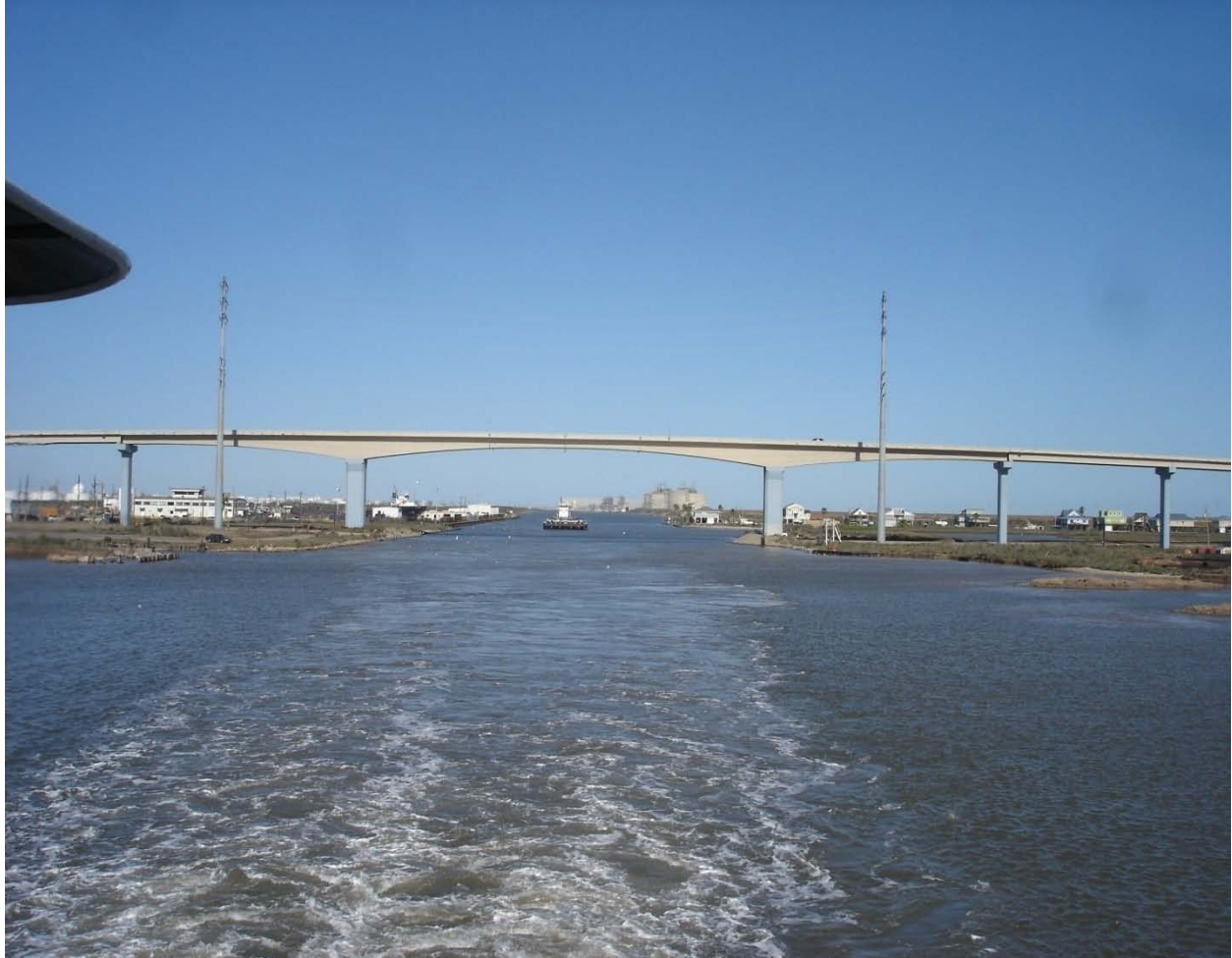
Figure 24. Bryan Beach Bridge.
