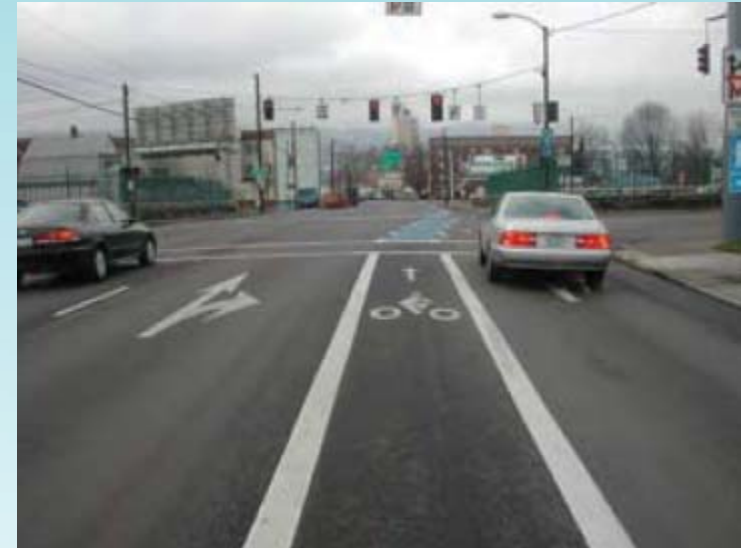
Example of blue bike lane between right turn lane and shared right-through lane (Portland, OR)
