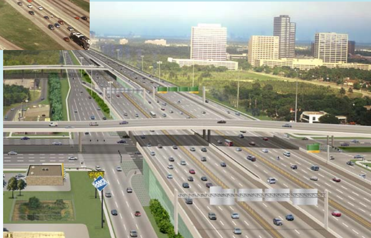
IH10 at SH 6, After Construction
