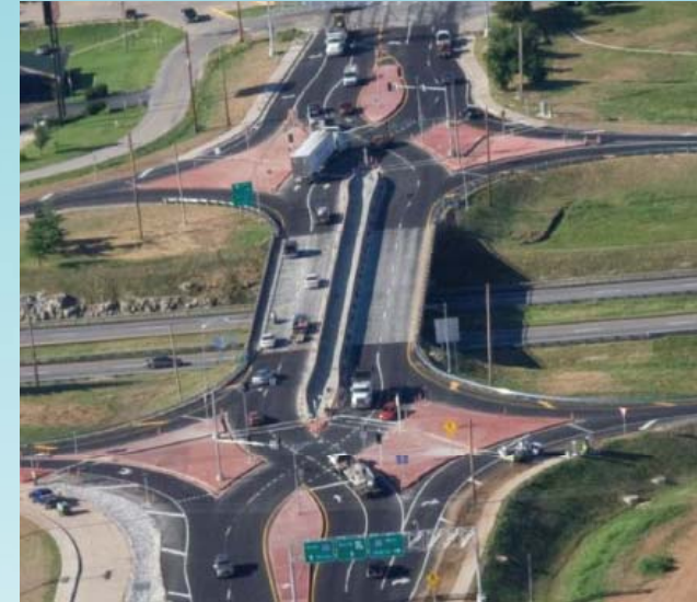
Diverging Diamond Interchange, I-40 at Hwy 13, Springfield, MO
