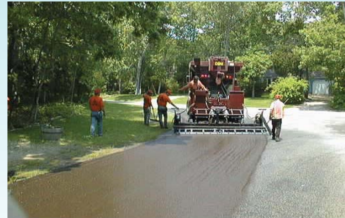
Application of skid-resistant pavement surface in curve.
