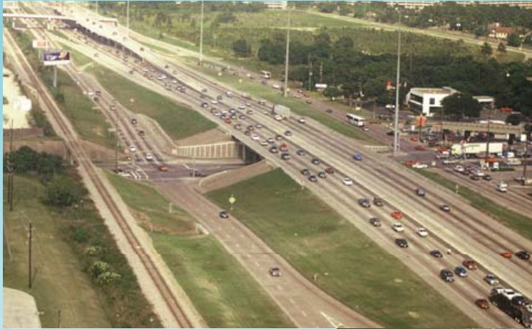
IH10 at SH 6, Before Construction
