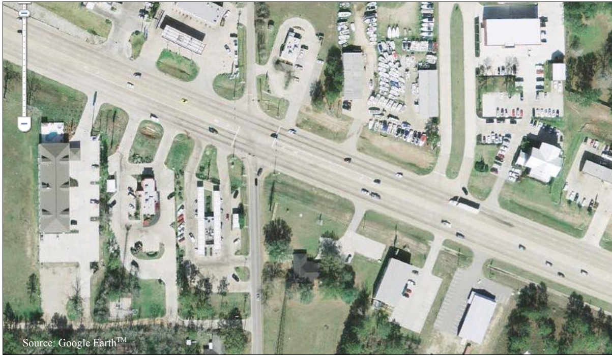
Figure 44. High Access Density on SH 105 Near McCaleb Road.
