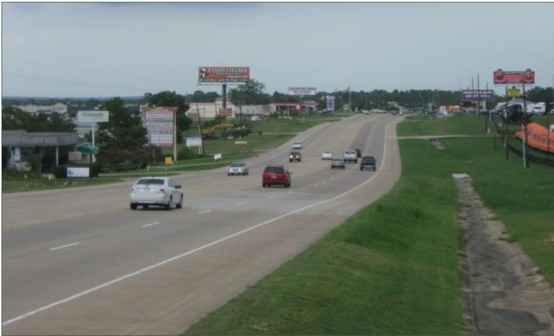
Figure 41. Existing 5-Lane Section of SH 105 on West Side of Corridor Study Area.
