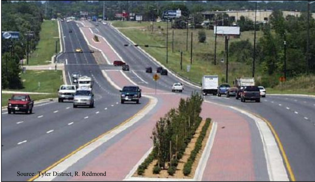
Figure 50. Loop 323 in Tyler: Example of High Speed, Multi-lane Arterial with Raised Median.
