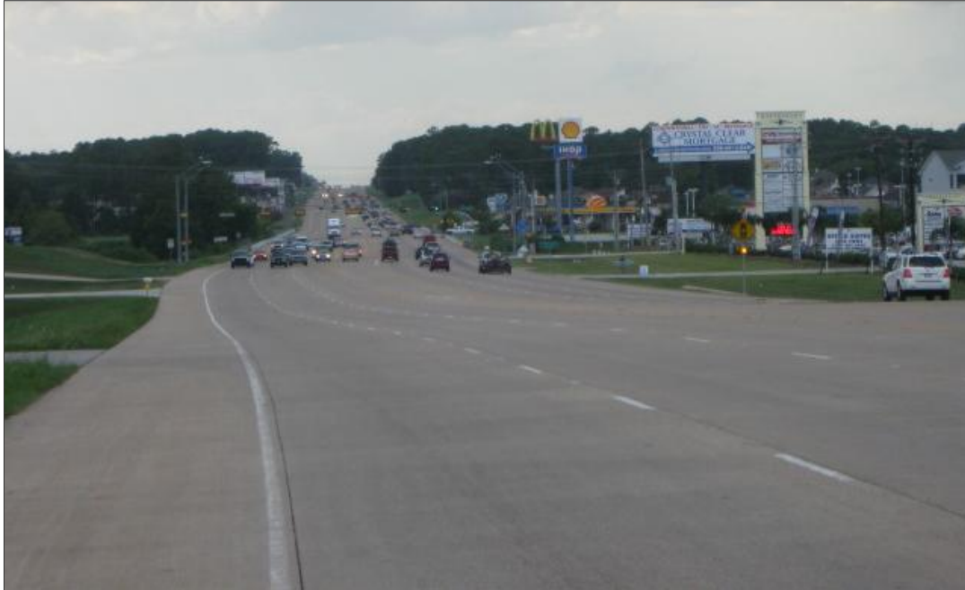
Figure 42. Existing 7-Lane Section of SH 105 on East Side of Corridor Study Area.
