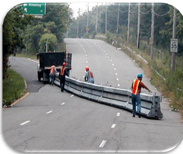
Figure 20. Example of the Deployment and Use of Steel Barrier.
