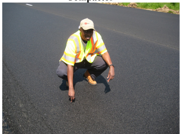
Figure E-6. Example of Finished HMA Mat.
