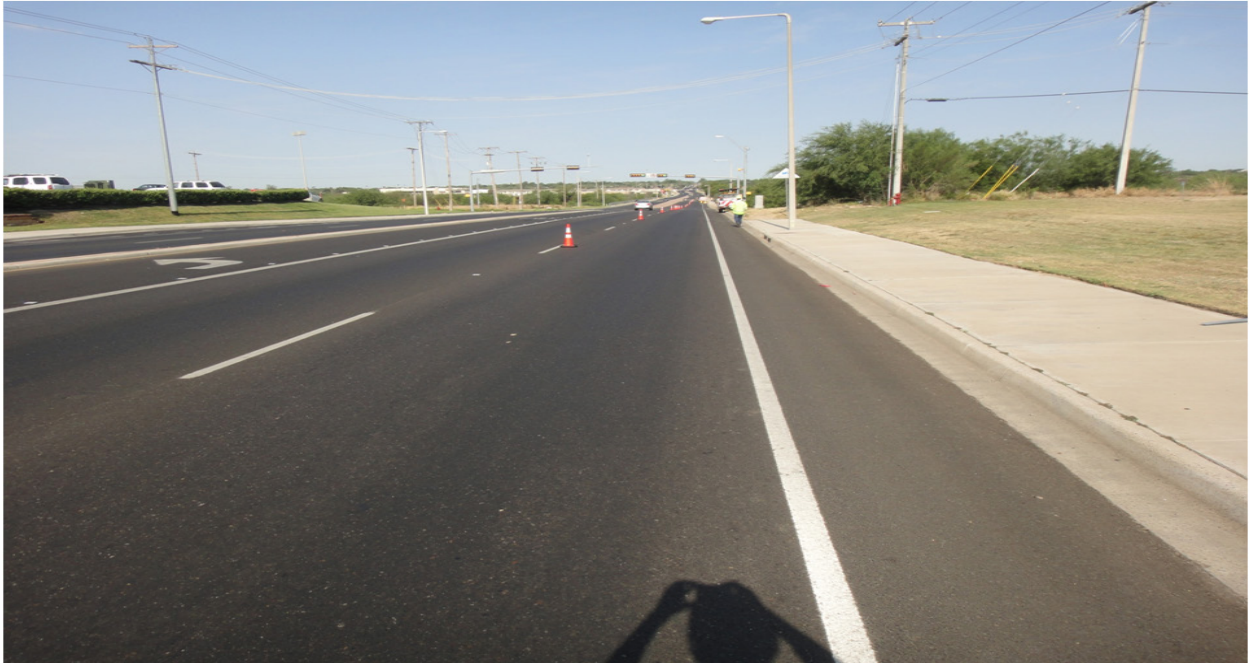
Figure G-5. Spur 400 WB Direction – No Cracking or Rutting Observed - LRD.
