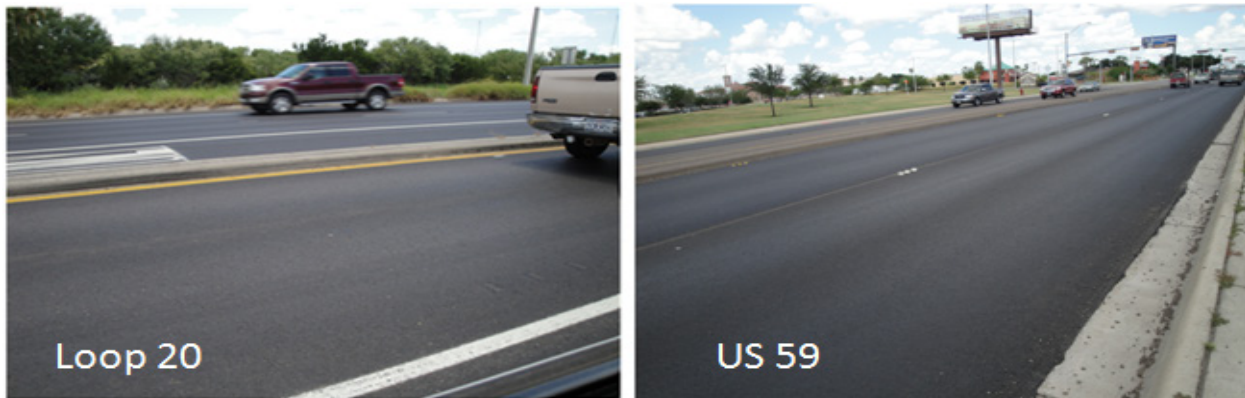
Figure 6-16. Example Completed 2 inch Thick HMA Mats on Loop 20 and US 59. (5.0%PG 64-22 + Crushed Gravel + 20% RAP + 1% Lime)
