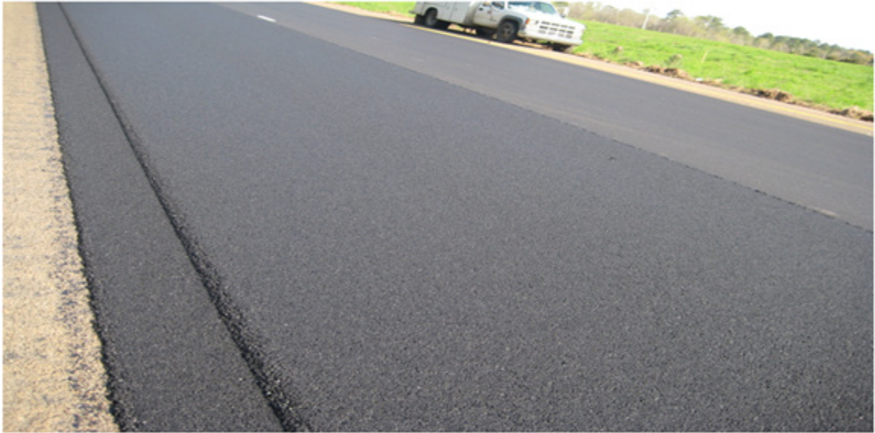
Figure 6-6. Example of Finished HMA Mat on Control Section 01 (ATL).
