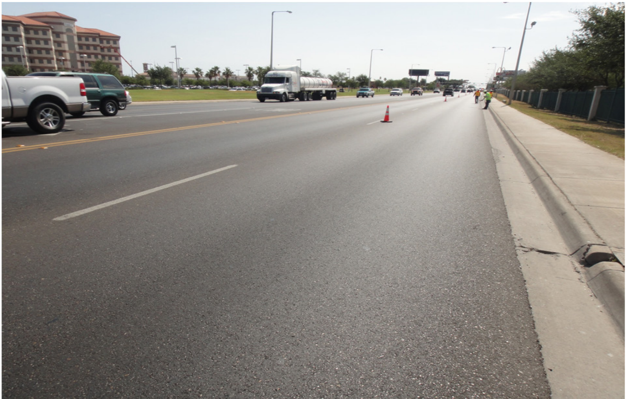
Figure G-6. US 59 EB Direction – No Cracking or Rutting Observed - LRD.
