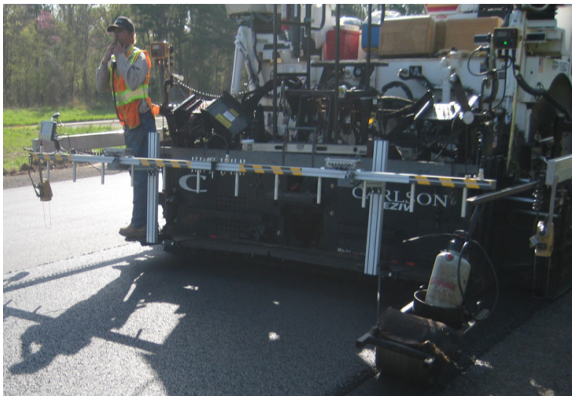
Figure E-3. IR (Temp.) Bar Setup.
