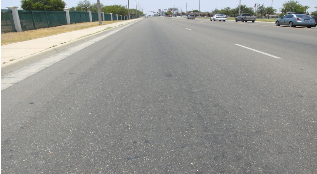
Figure 6-19. Field Performance – US 59 (Oct 2012) – No Distresses (LRD).
