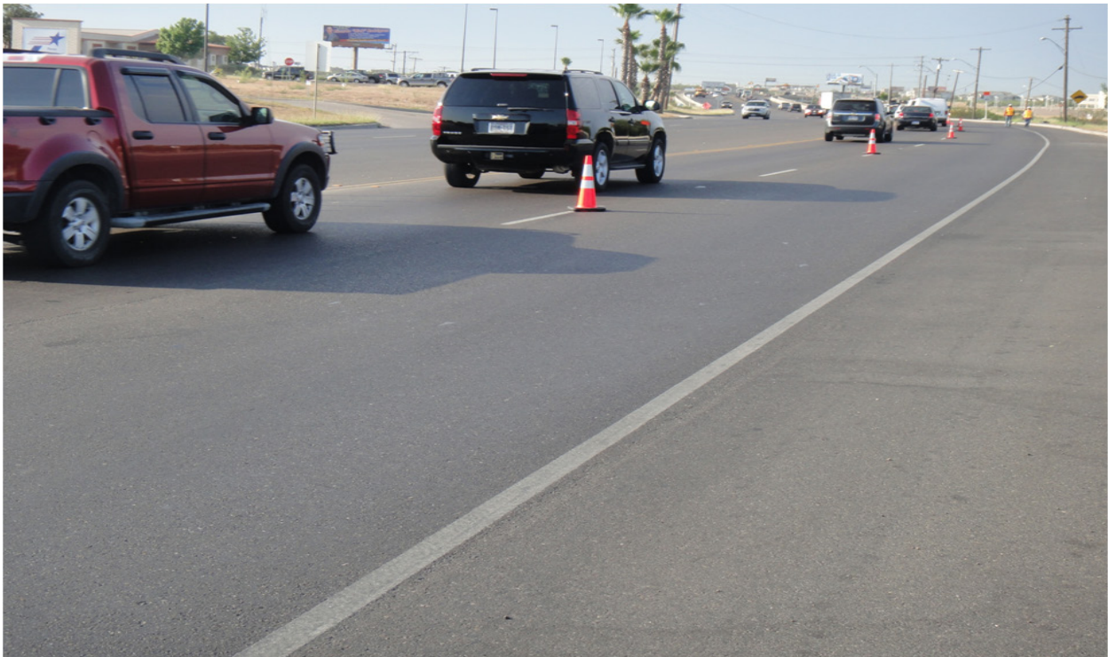
Figure G-4. Loop 20 SB Direction – No Cracking or Rutting Observed - LRD.
