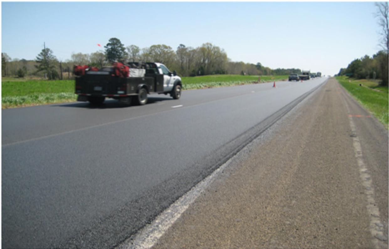
Figure 6-7. Example of Finished HMA Mat on Control Section 01 (ATL).
