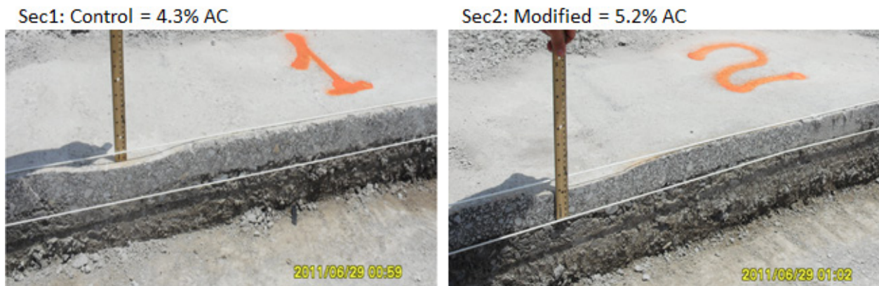
Figure 5-4. Trenching and Pictorial Comparison of Rutting on Test Sections 1 and 2.
