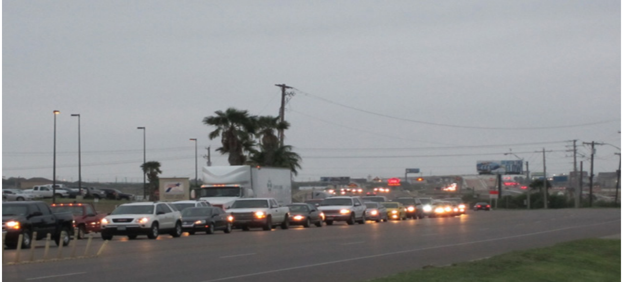
Figure 6-17. Field Performance – Loop 20 (Oct 2012) – No Distresses (LRD).
