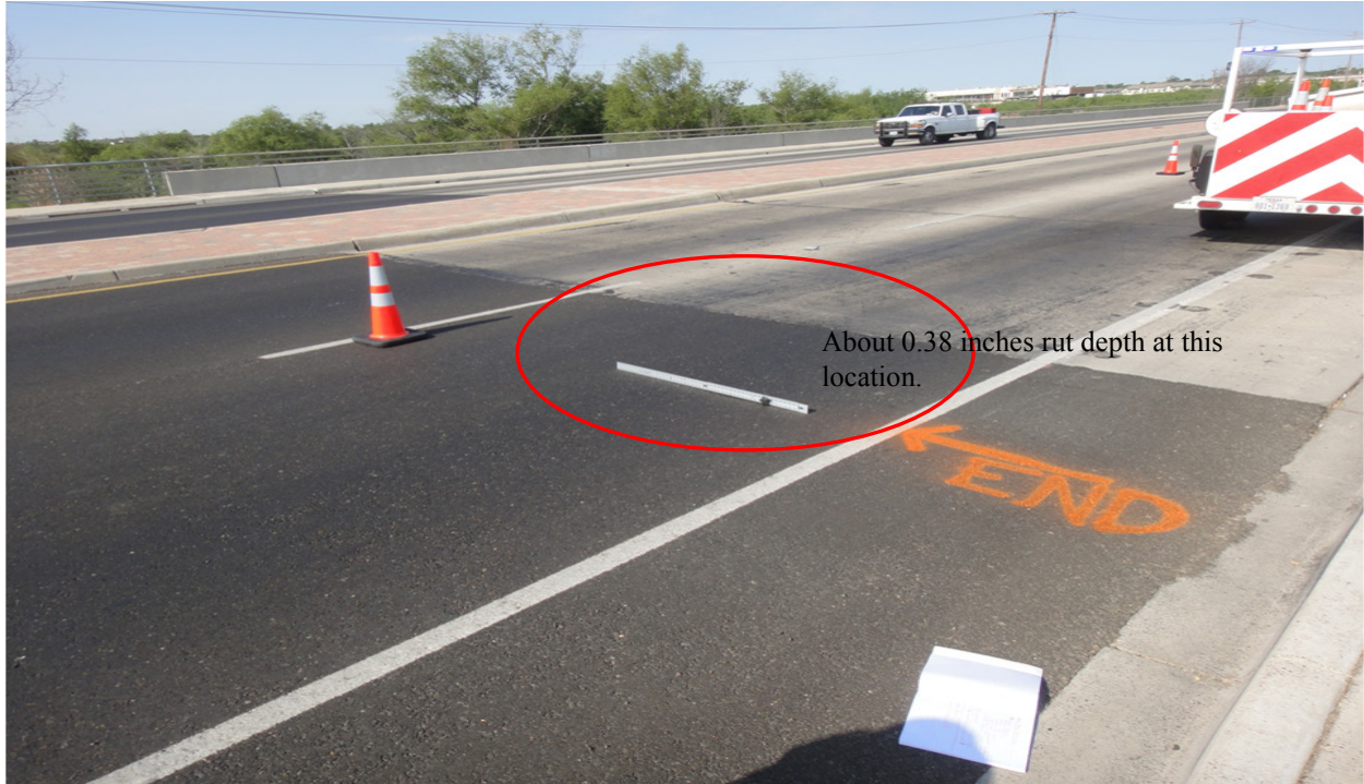
Figure G-9. HMA to Bridge Concrete Deck Transition \cong 0.38 Inches Rut Depth (Spur 400) - LRD.
