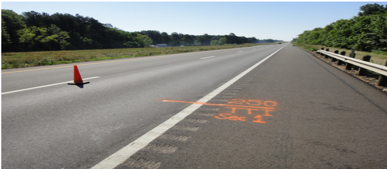
Figure 6-8. Field Performance – Control Test Section 1 (Oct 2012) – No Distresses (ATL).
