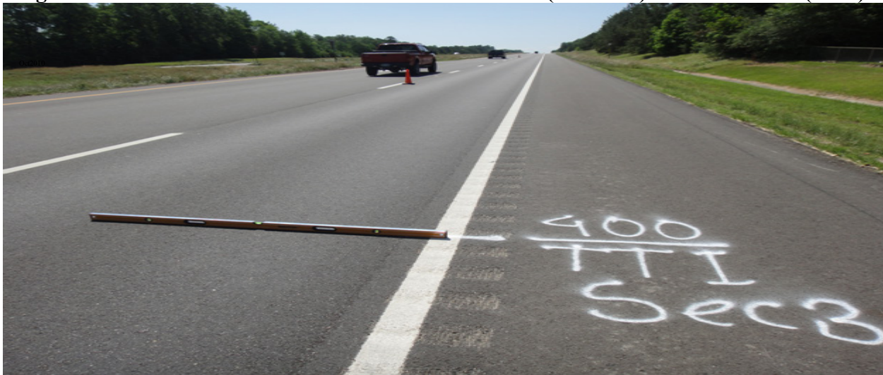
Figure 6-10. Field Performance – Control Test Section 2 (Oct 2012) – No Distresses (ATL).
