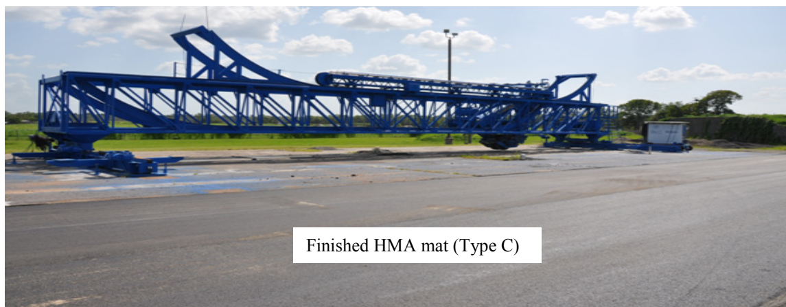
Figure 3-6. Finished HMA Mat at the LTRC-APT Test Site (August 2009).
