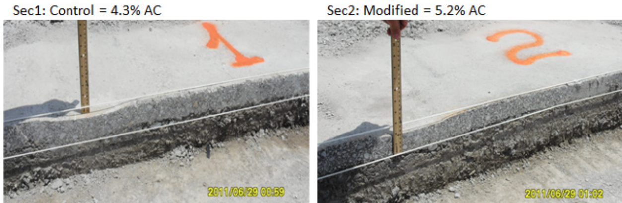
Figure 5-3. Trenching and Pictorial Comparison of Rutting on Sections 1 and 2.
