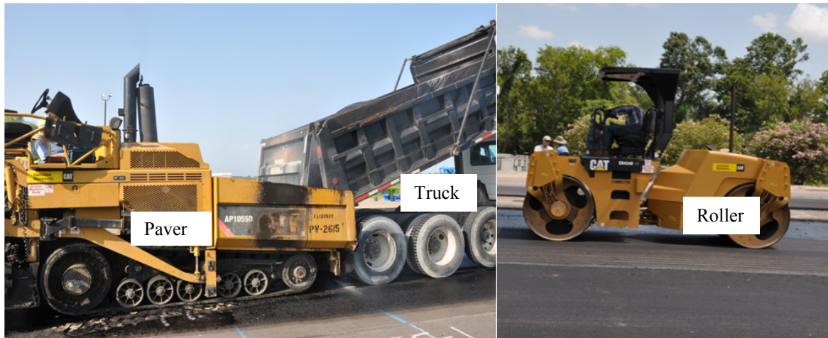
Figure 3-5. HMA Placement and Compaction Operations.
