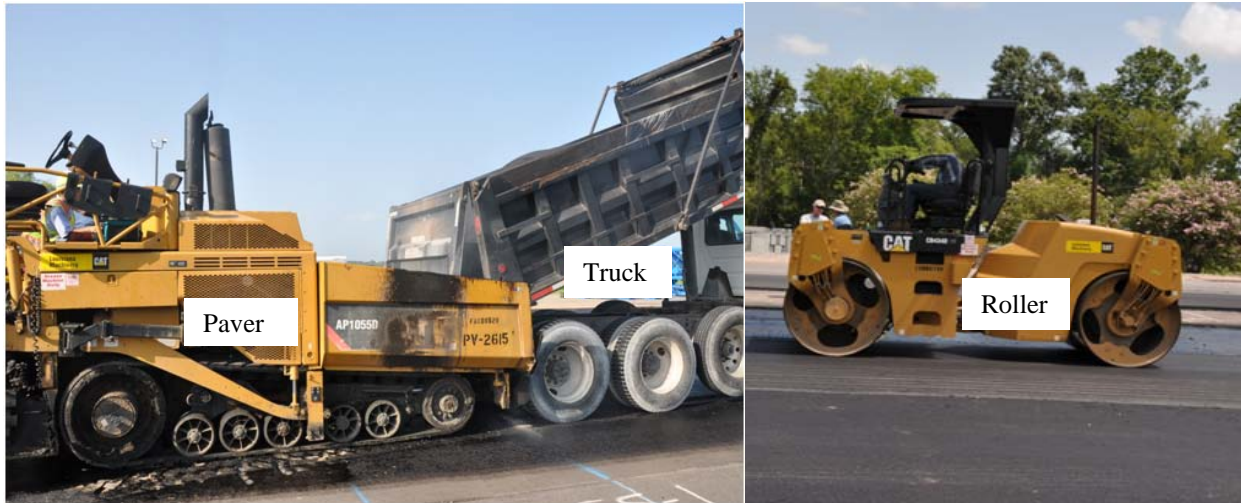
Figure 8-6. HMA Placement and Compaction Operations.
