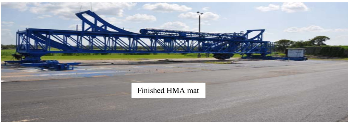
Figure 8-7. Finished HMA Mat at the LTRC-APT Test Site (August 2009).
