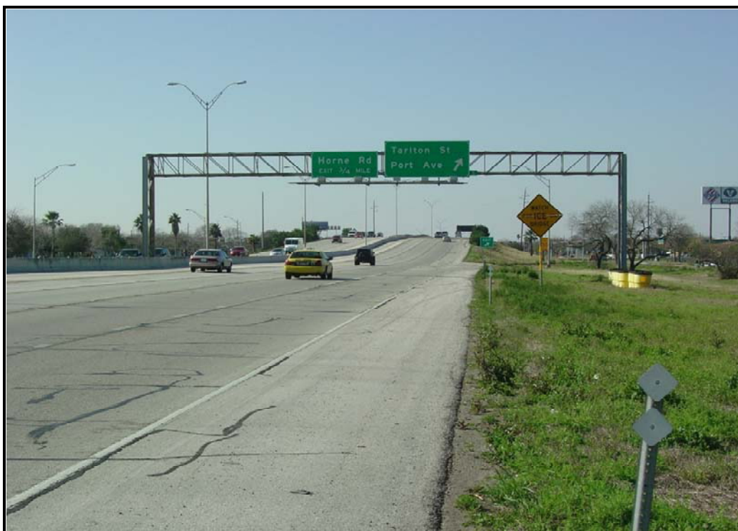
Figure 25. Southbound SH 286 Exit to Port Avenue, Corpus Christi, Texas.
