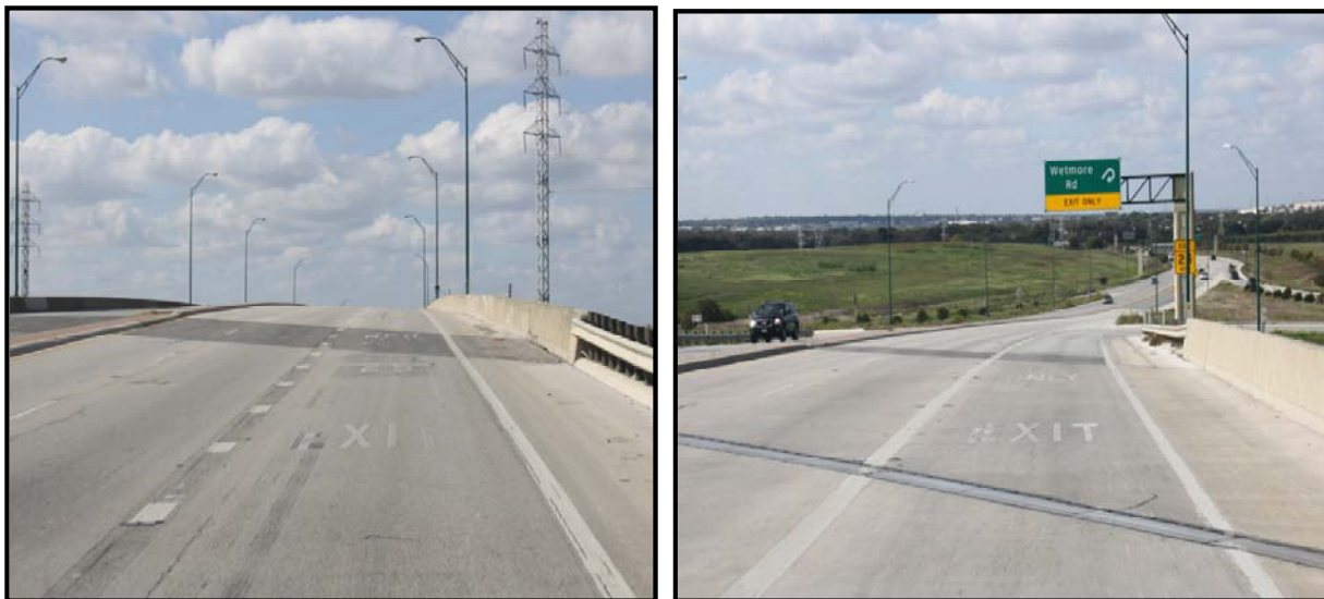
Figure 18. Example of a Potential Hazard—Steep Grade before an Exit.
