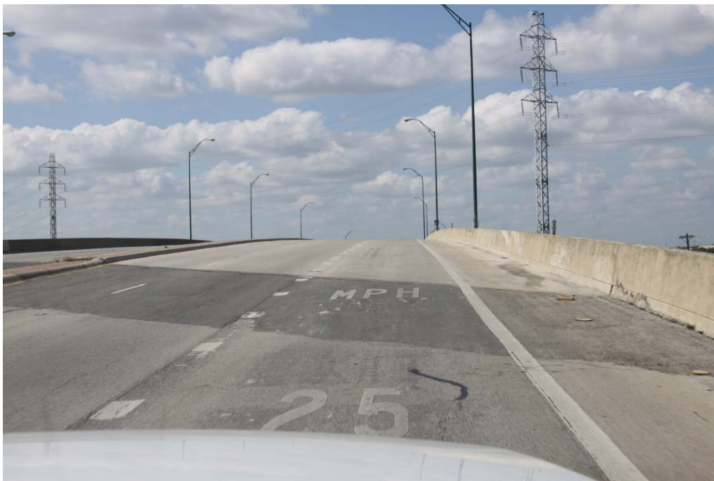
Figure 44. Example of Painted Ramp Speed on Approach to Exit on Wurzbach Parkway.
