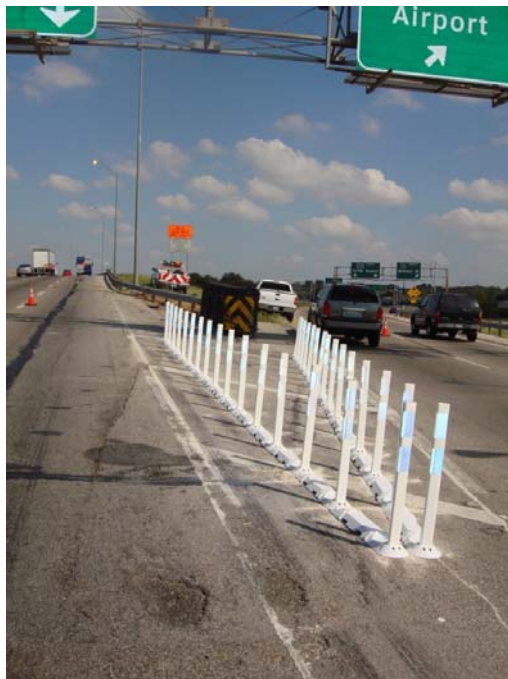
Figure 5. Curb Attenuator.
