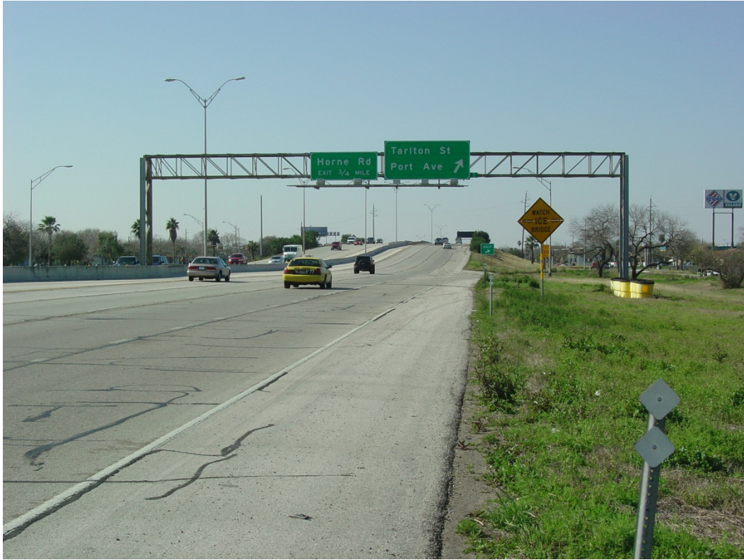
Figure 41. Southbound SH 286 Exit to Port Avenue.
