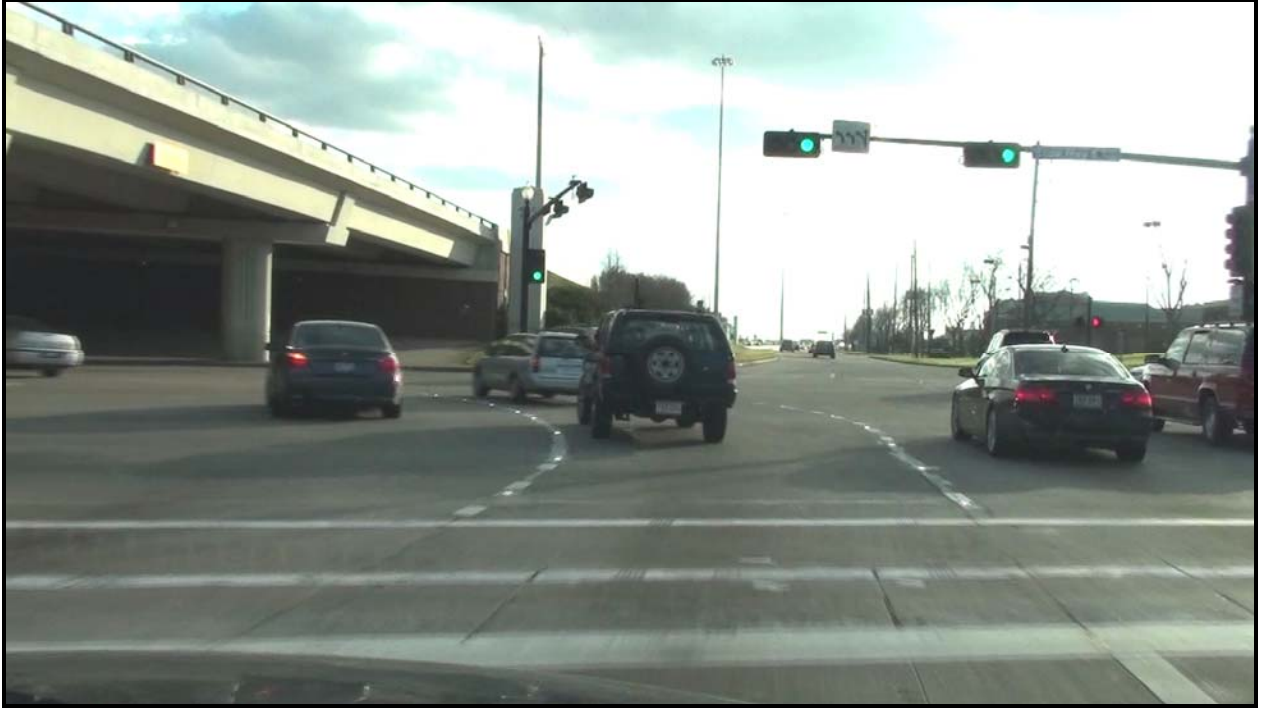
Figure 4-9. Triple Left-Turn LPM System in Sugar Land, Texas (Daytime).
