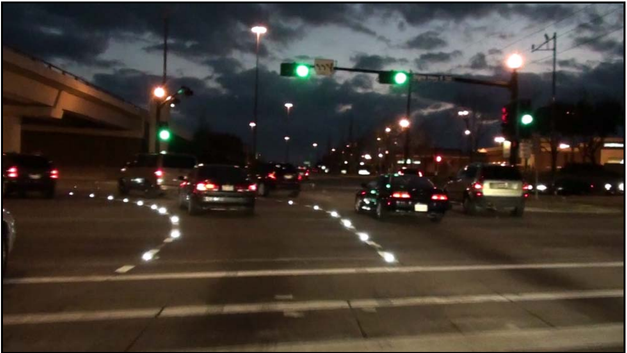
Figure 4-10. Triple Left-Turn LPM System in Sugar Land, Texas (Nighttime).
