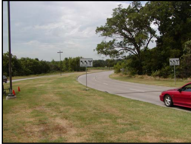
Figure 4-3. Advanced Traffic Sign – Southbound Gerault Road Approach.
