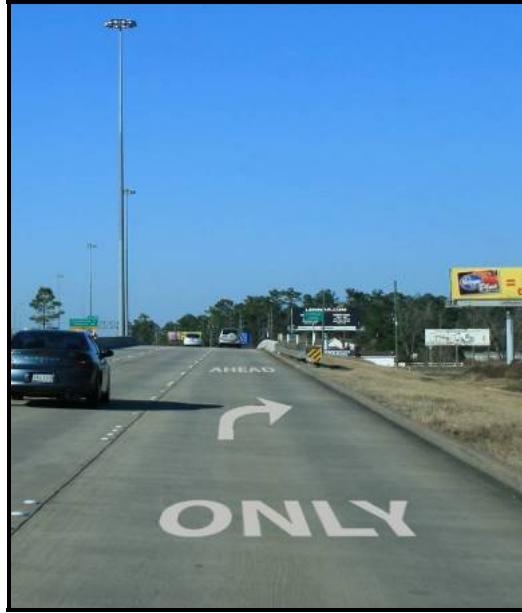
Figure 110. Example of Advanced Pavement Markings for a Turn-Only Lane with the Text “AHEAD.”
