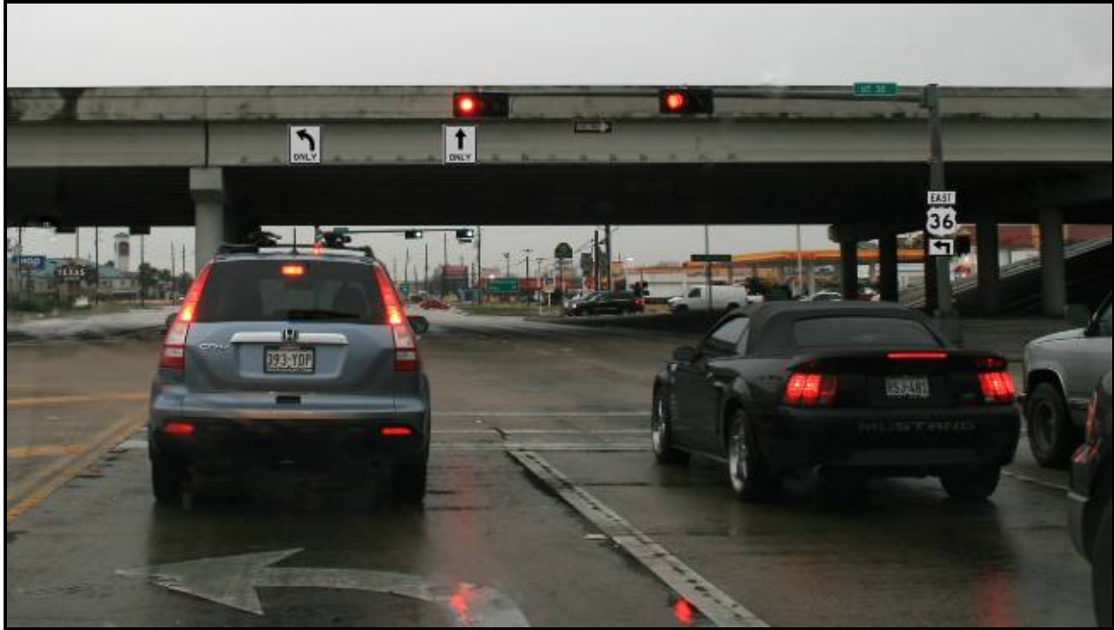
Figure 107. Example of Overhead Signing Used on a Cross-Street Approach to a Freeway. Guideline 4. Avoid using right-angled arrows on guide signs for lane assignment.
