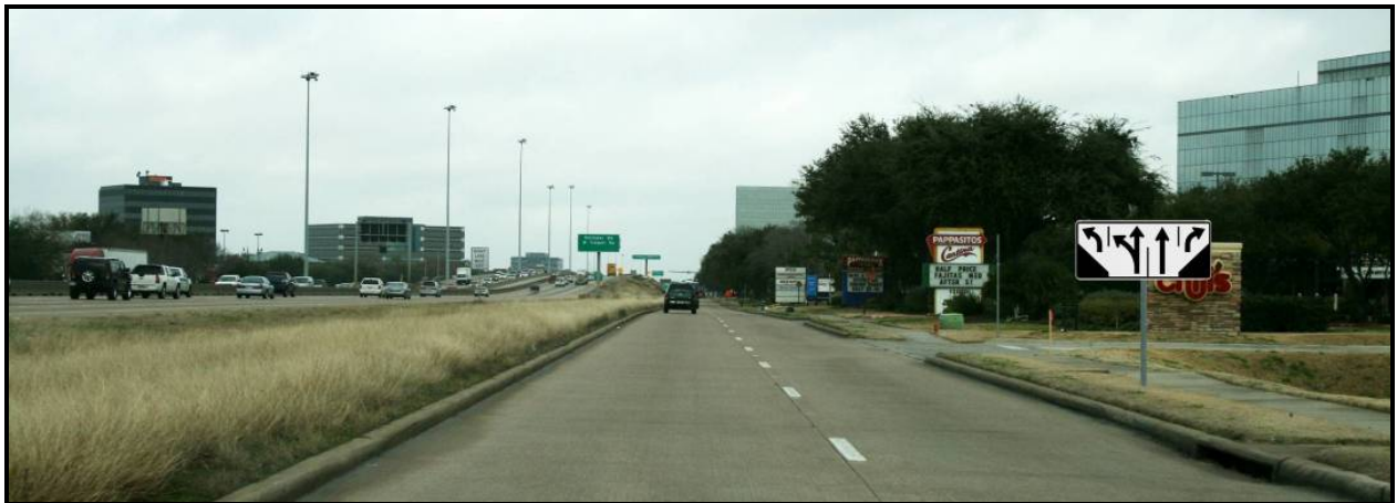
Figure 111. Example of a Lane Assignment Sign with Lane Tapers Placed before the Flare of the Roadway.
