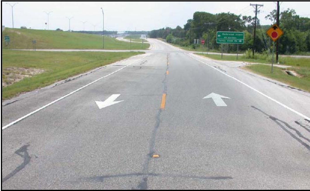
Figure 113. View of Frontage Road Lane Use Guidance after Arrow Pavement Marking Installation. (3)
