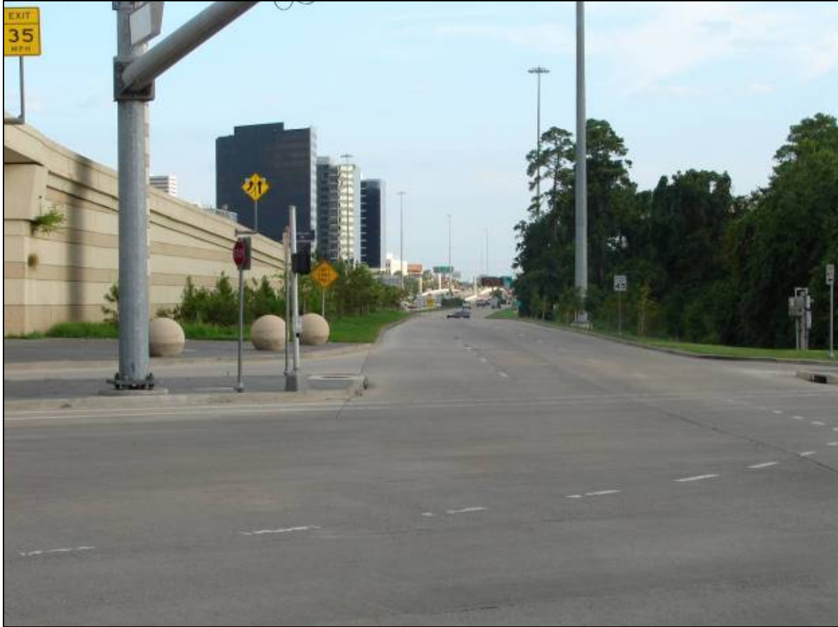
Figure 56. Focus Group Visual: Example of a Lane Drop on Far Side of the Intersection.
