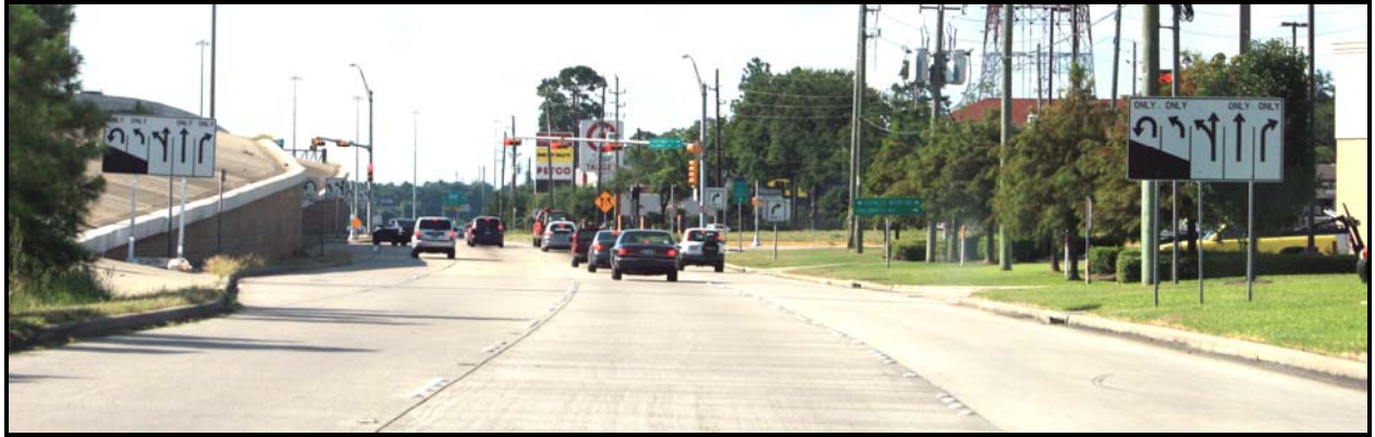
Figure 103. After #1 Signs (IH 45 Southbound at Cypresswood Drive).
