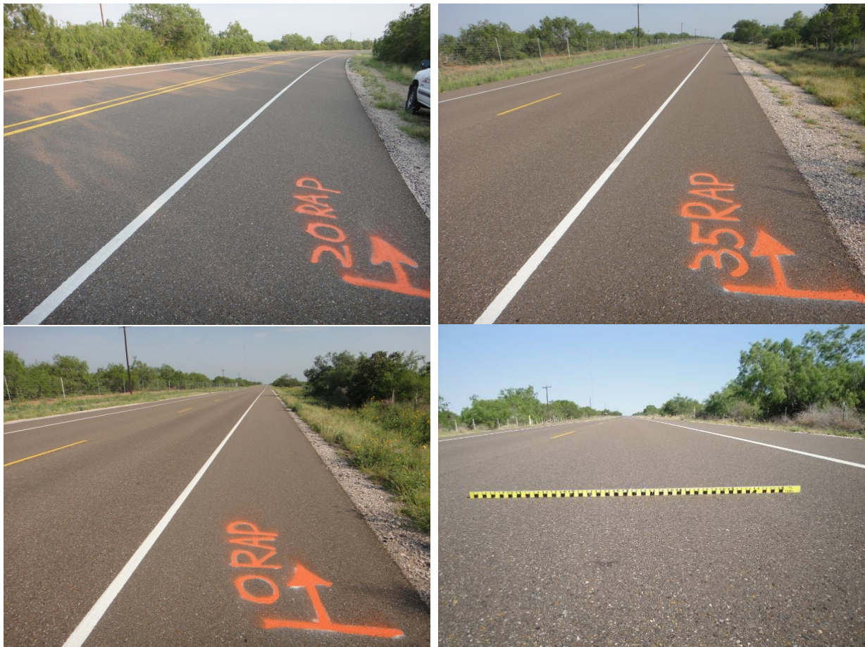
Figure 4. RAP Test Sections on FM1017 on May 25, 2012.
