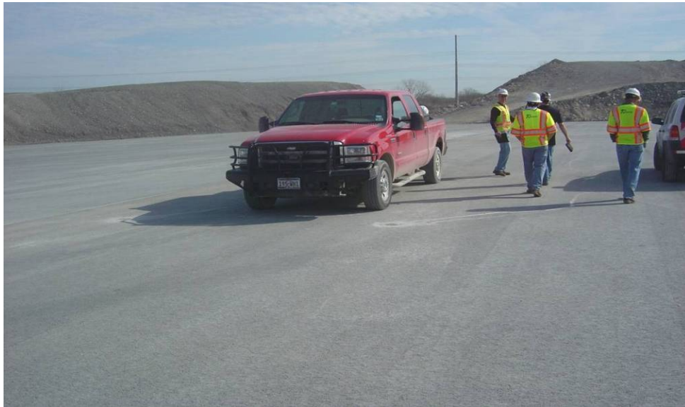
Figure 2-8. Paved, Sloped Stockpiles Surface.
