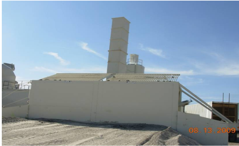
Figure 2-10. Two RAP Bins.
