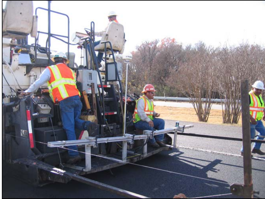
Figure 11. Pave-IR Collecting Thermal Profile on US 75.
