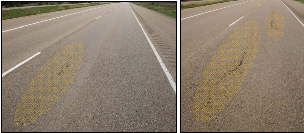
Figure 108. Examples of Cyclical Distress on SH 21.
