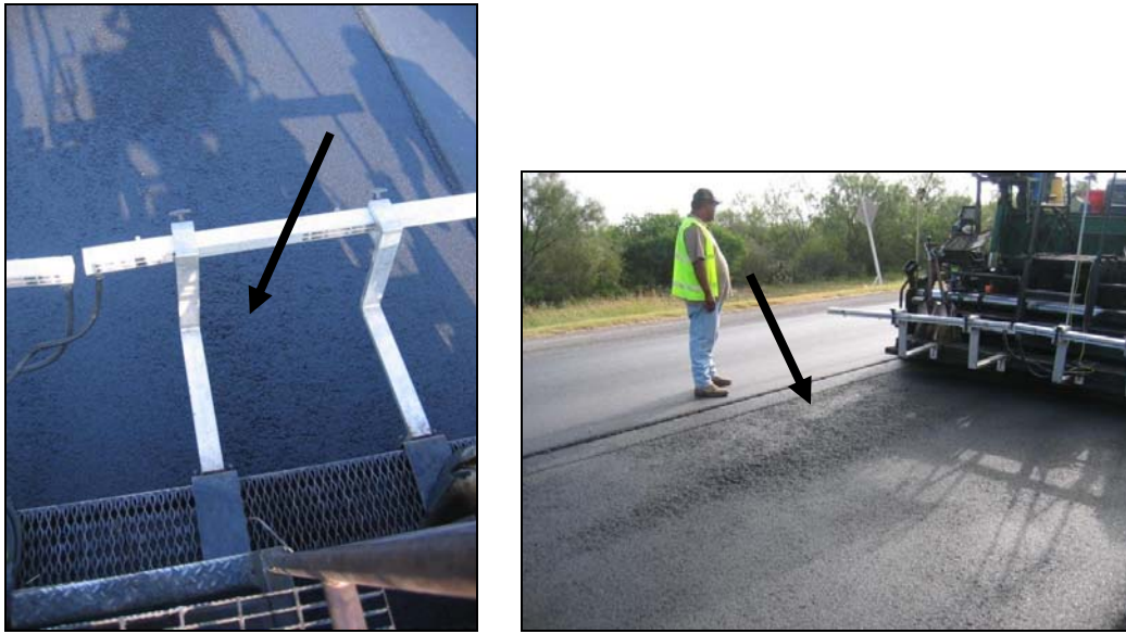
Figure 72. View of Cold Spot on US 90 CAM. Note: corresponds with 520 ft in Figure 57.
