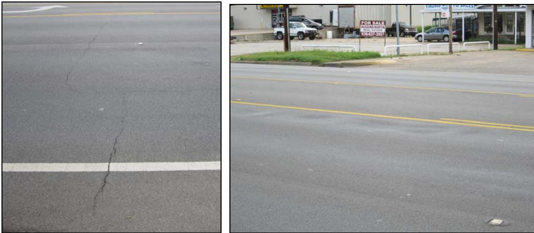
Figure 67. Distresses Observed on BU 59 after Five Years of Service.
