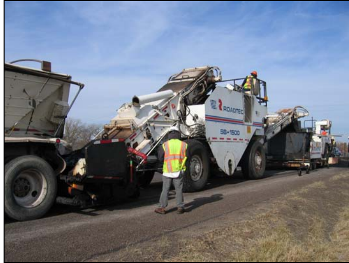
Figure 10. Paving Operation on US 75.
