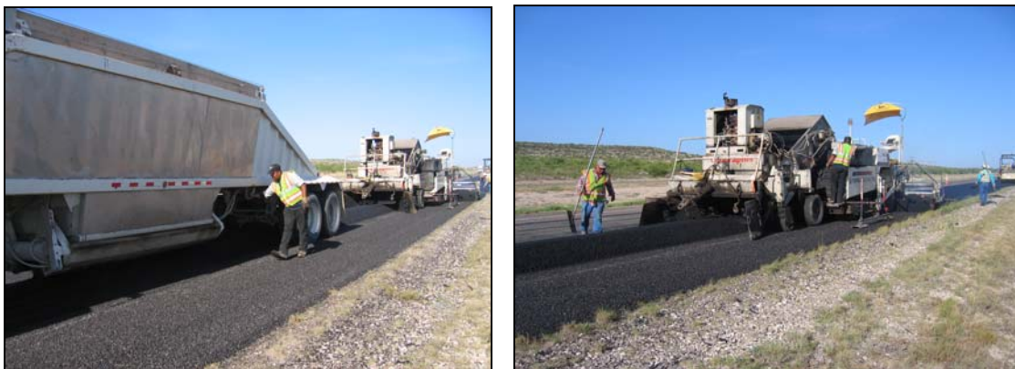
Figure 56. Belly Dump and Windrow Operation on IH 10 CRM.
