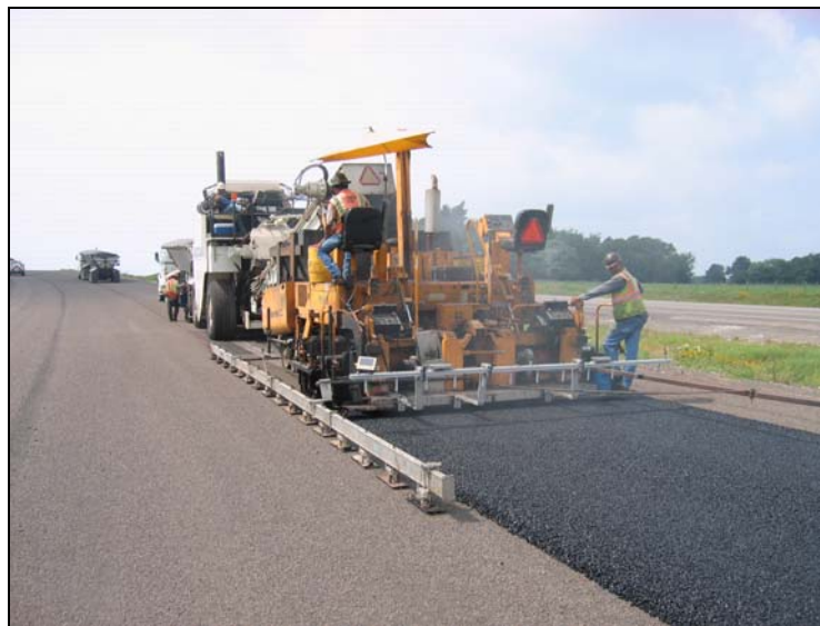
Figure 92. Paving Train on SH 6 PFC.
