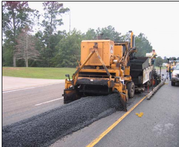
Figure 99. Paving Operation on US 190.
