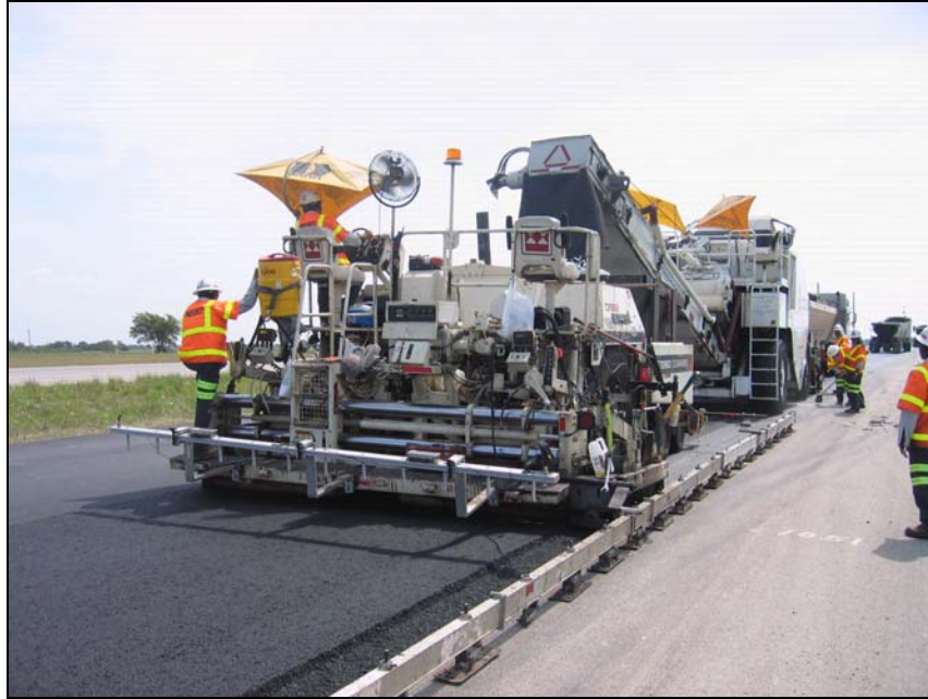
Figure 31. Paving Operation on US 81.
