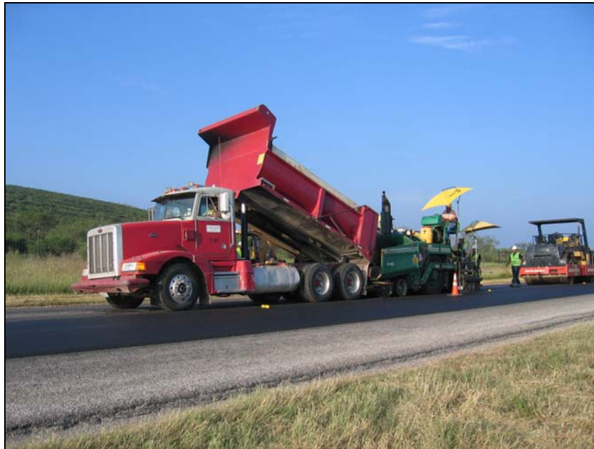
Figure 69. Paving Operation on US 90 CAM Mix.
