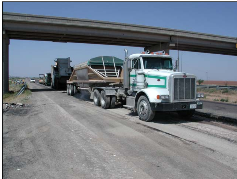
Figure 1. IH 20 1 In. Superpave Site.
