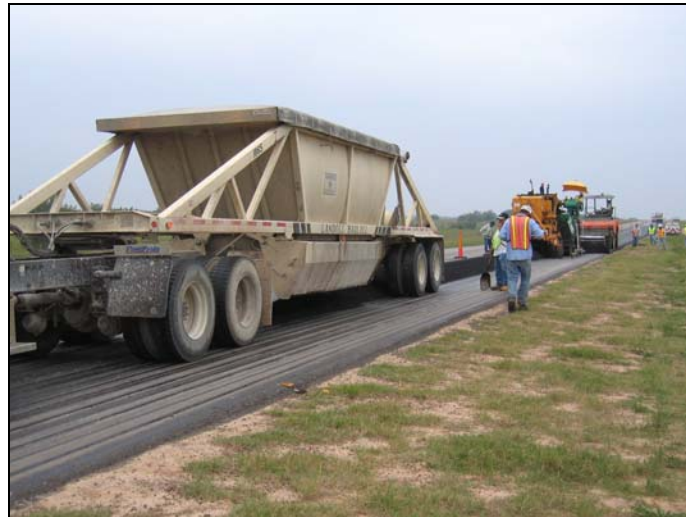
Figure 46. Paving Operation on US 77 Northbound, May 10, 2006.
