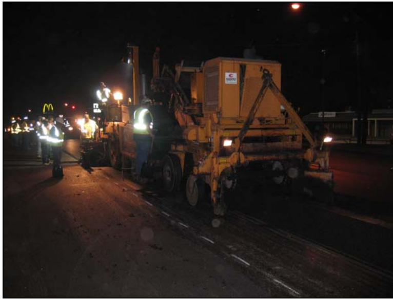
Figure 65. CAM Paving Operation on Business 59.
