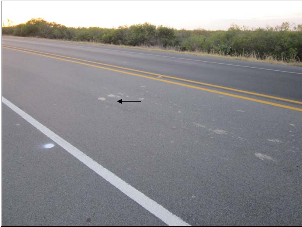
Figure 74. US 90 Thermally Segregated Locations. Note: corresponds to ~450 ft in Figure 70 .
