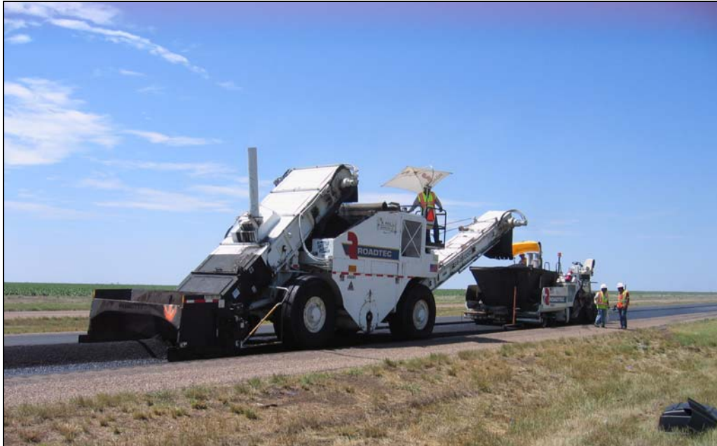
Figure 22. Paving Operation on IH 40.
