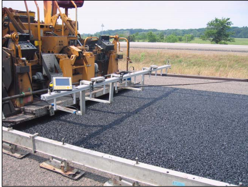
Figure 93. Pave-IR Collecting Thermal Profile on SH 6.
