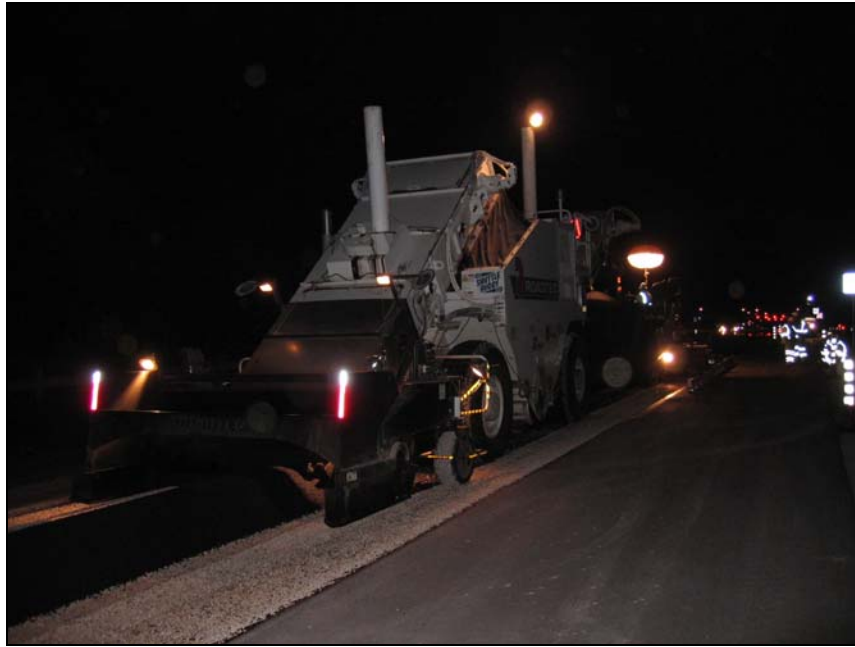
Figure 85. Paving Operation on Parmer Lane.
