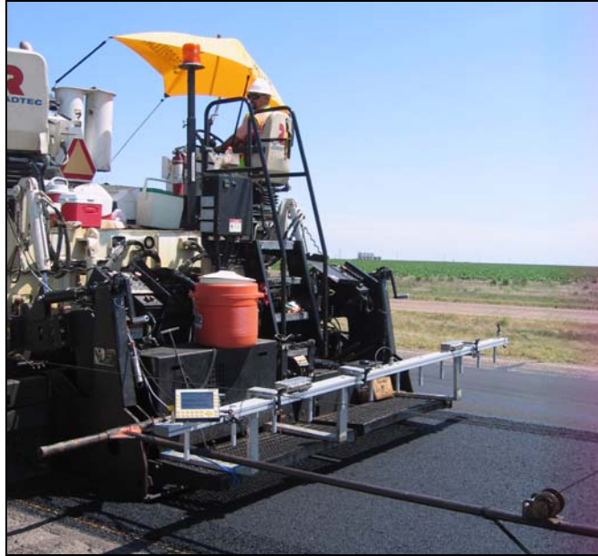
Figure 23. Pave-IR Installed and Collecting Thermal Profile on IH 40.
