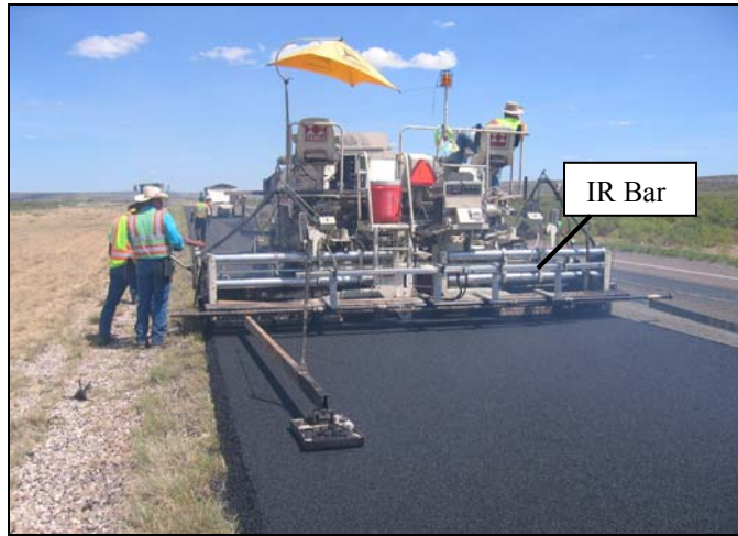
Figure 57. Paver with IR Bar Installed on IH 10 CRM.
