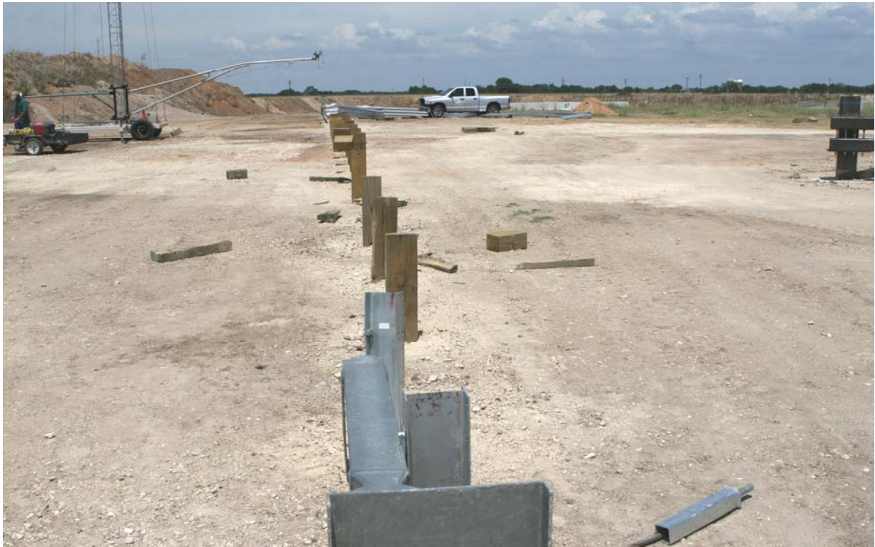
Figure 6.6. Installation after Test No. 460719-3.
