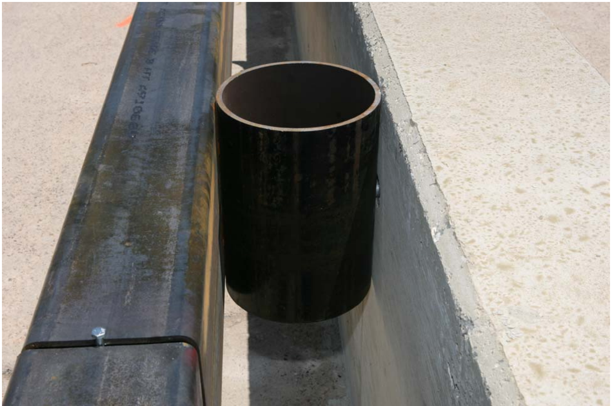
Figure 5.2. Energy-Absorbing Bridge Rail Installation before Test Nos. 470619-1 and 2.
