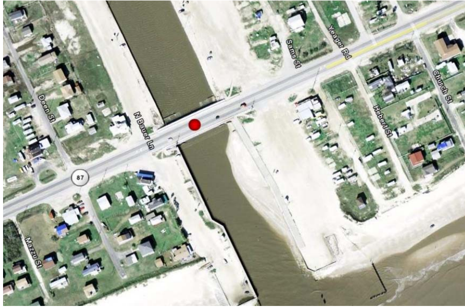
Figure 9. A Bridge (Red Dot) at Rollover Pass in Galveston. (Google Satellite Image, 2009c)
