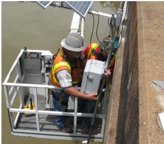
Figure D-4. Mounting the Master Station.
