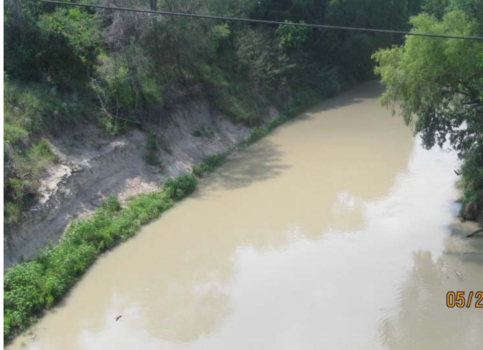
Figure 6-9. Northern Riverbank of San Antonio River (Downstream).
