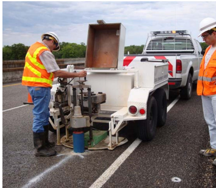
Figure 5-14. Drill the Hole through the Deck.
