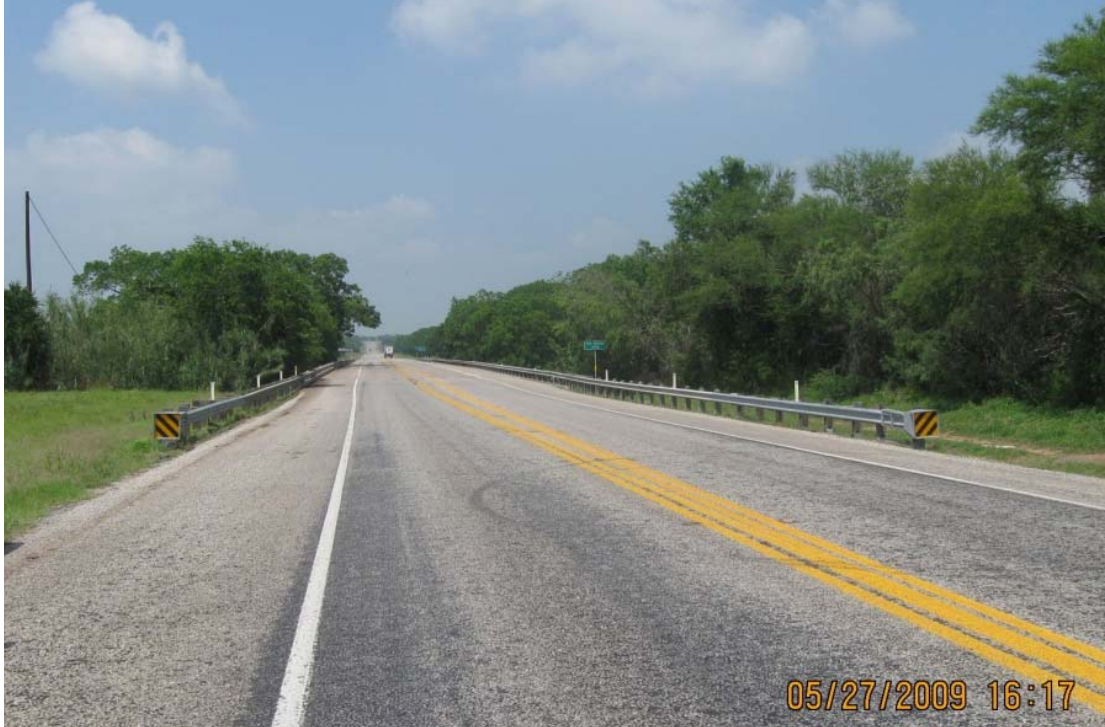
Figure E-3. State Highway 80 over San Antonio River Bridge, Texas.
