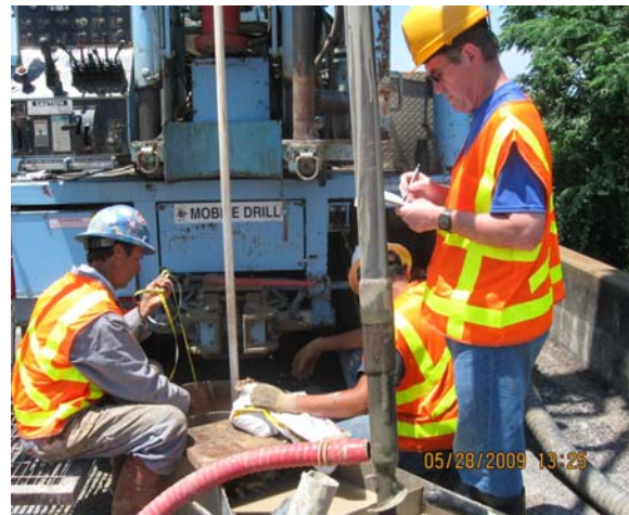
Figure 5-18. Refilling the Drilled Hole.
