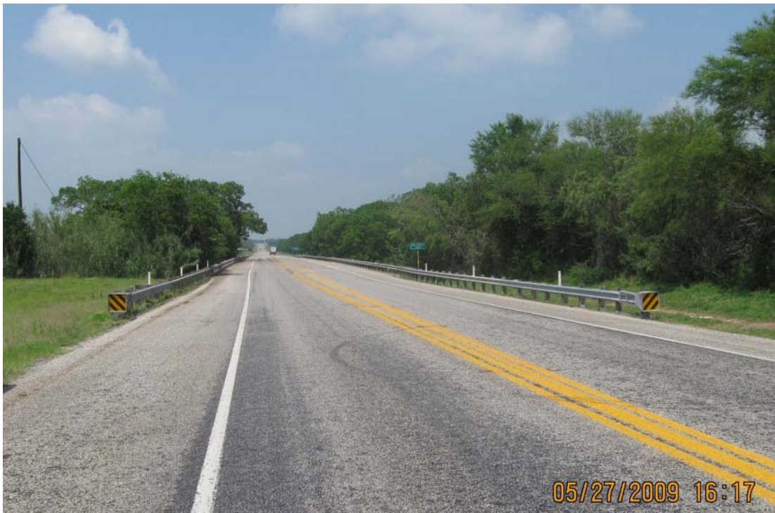
Figure 6-3. State Highway 80 over San Antonio River Bridge, Texas.
