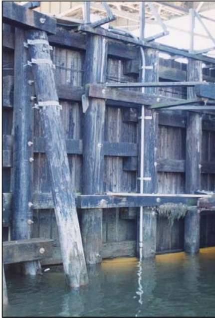
Figure C-14. Velocitymeter Mounted on Bridge Fender (MSHA).
