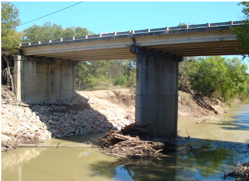
Figure E-4. River Pier with Concrete Web-Wall (P2).
