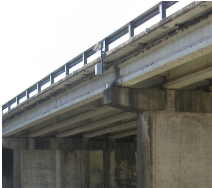
Figure E-16. Bridge Scour Monitoring System.
