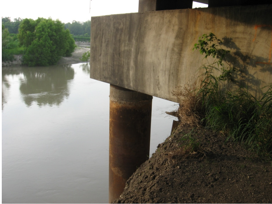
Figure 5-6. Drill Shaft on Northeast Side (SB0) of US59 over Guadalupe River Bridge in 2010.
