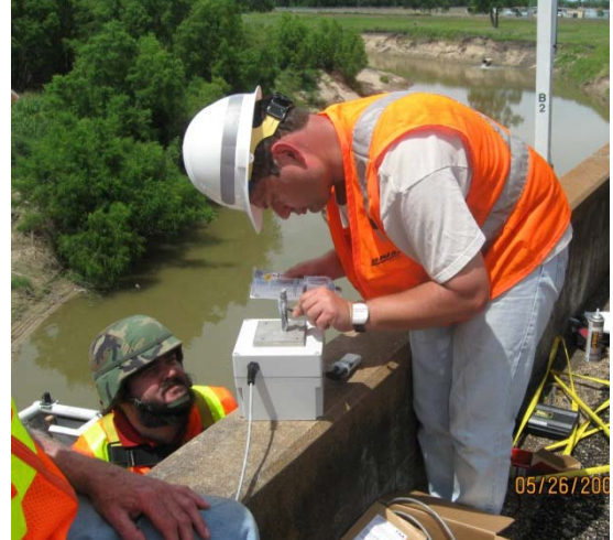
Figure D-10. Applying Glue to the Tiltmeter Enclosure.
