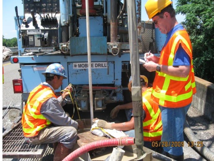
Figure D-26. Refilling the Drilled Hole after the Installation of the Float-Out Devices.
