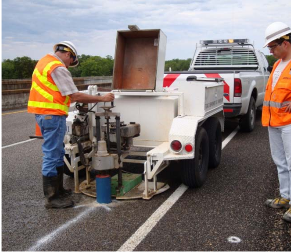
Figure D-19. Drilling the Hole through the Bridge Deck.
