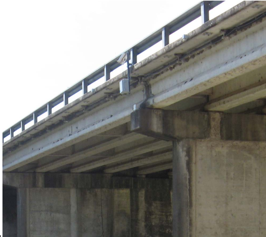
Figure 6-20. Modified Bridge Scour Monitoring System.
