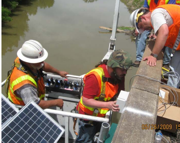
Figure D-9. Positioning the Tiltmeter.
