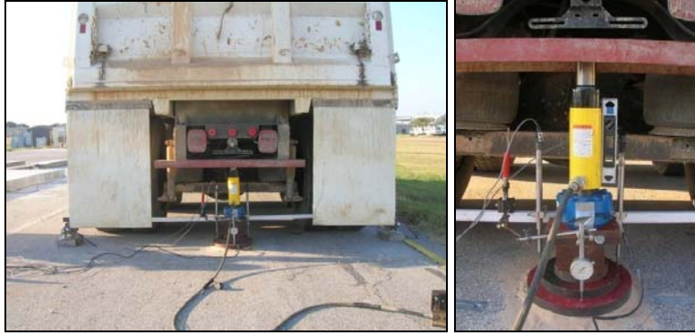
Figure 62. Plate Load Field Test.
