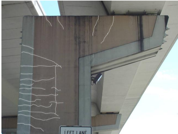
(a) Cantilevered bent
