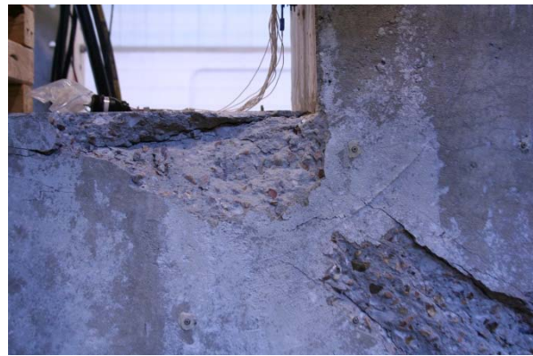
(d) After removal of the spalled concrete
