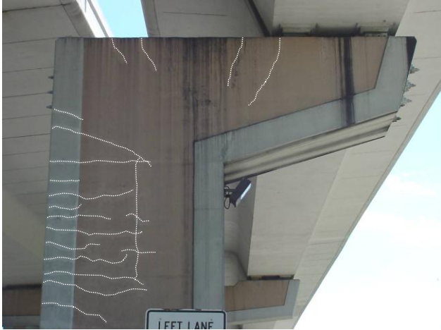
(a) Cantilevered bent
