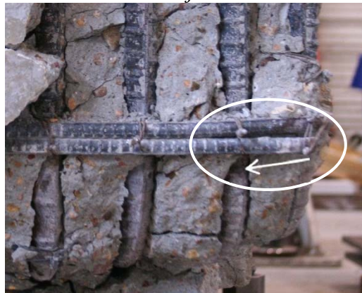
(e) Anchorage debonding of transverse U-bars
