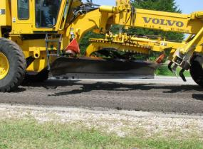
Figure 4. Grader Blade Position in Forward (Left) and Backward (Right) Movements.
