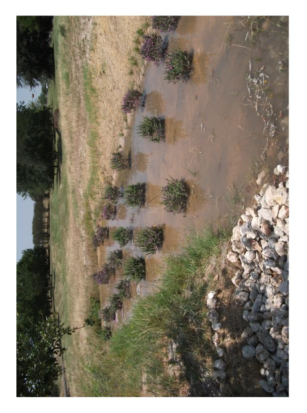
Figure 8. Flood Irrigation of Bioretention Cell (Photo Taken in June 2011).
