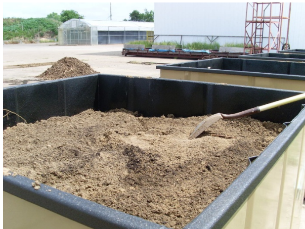
e. soil/compost filter media (2 feet in depth)
