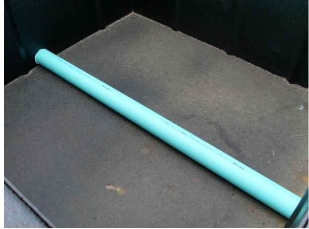
b. coated with liner/4 inches PVC underdrain
