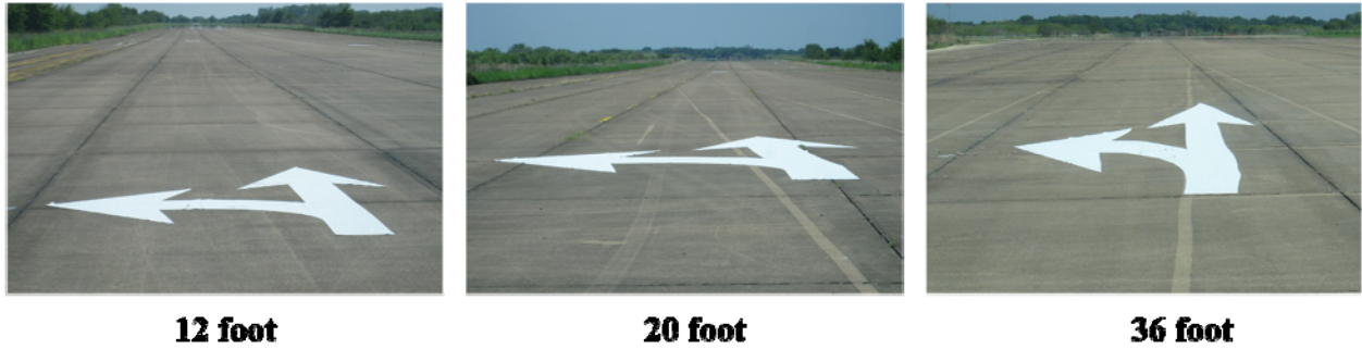
Figure 28. “Left and Through” Pavement Marking Symbols.
