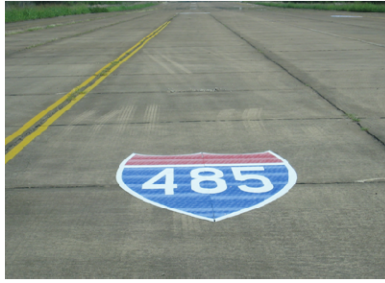
a) 15 foot Interstate Shield
