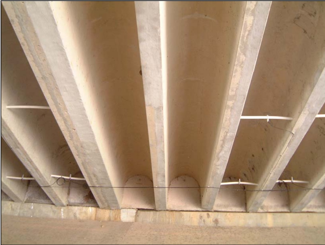
Figure 10. View underneath the F.M. 60 Bridge with GTT Probes in Place.
