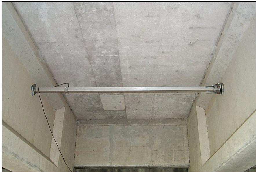
Figure 6. GTT Microloop Probe Support under F.M. 60 Bridge in College Station.
