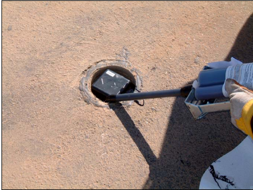
Figure 4. Sensys Networks VSN 240 Flush Mount Magnetometer Installation.
