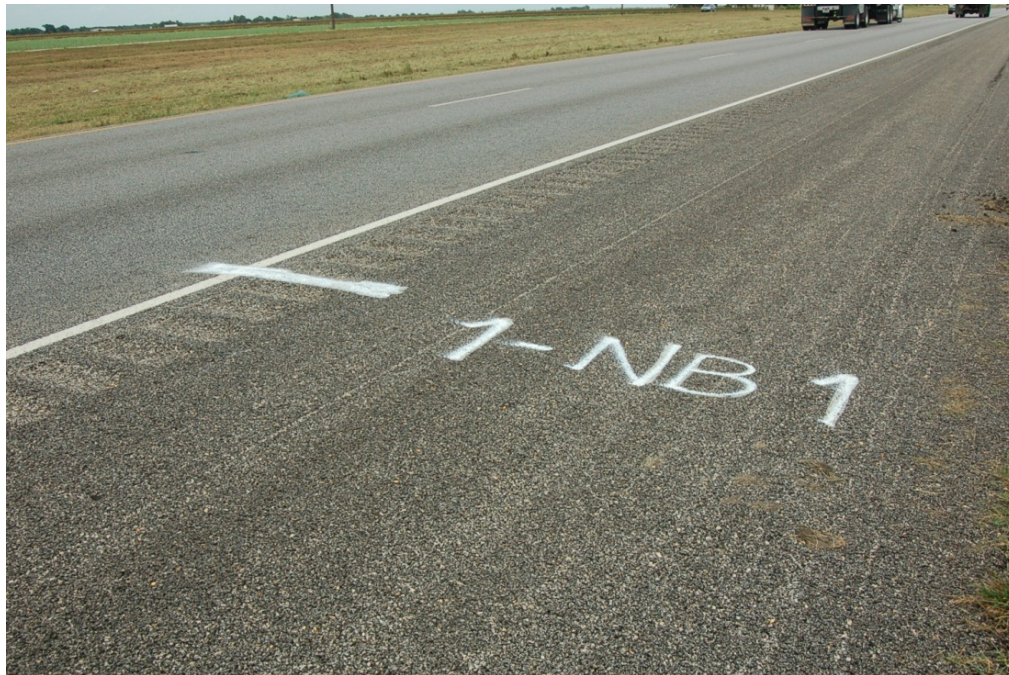
Figure C.2. PFC Pavement Section on US 59 (Section 1).
