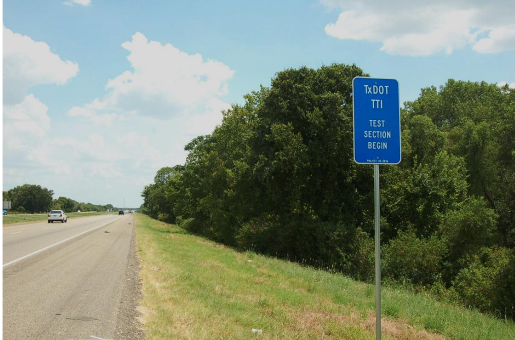
Figure C.30. View of SH6, Section 9 on SH 6, Westbound.
