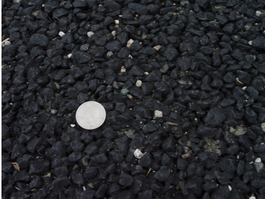
Figure C.35. Detailed View of the PFC Surface on US 281, Section 11, Northbound.
