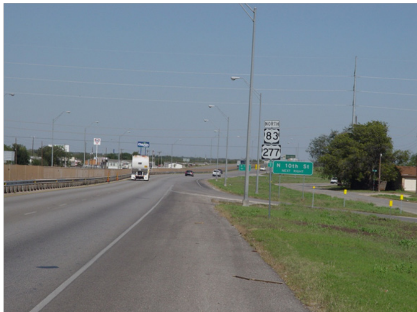
Figure C.26. View of US 83, Section 7, Subsection 7-1, Northbound.
