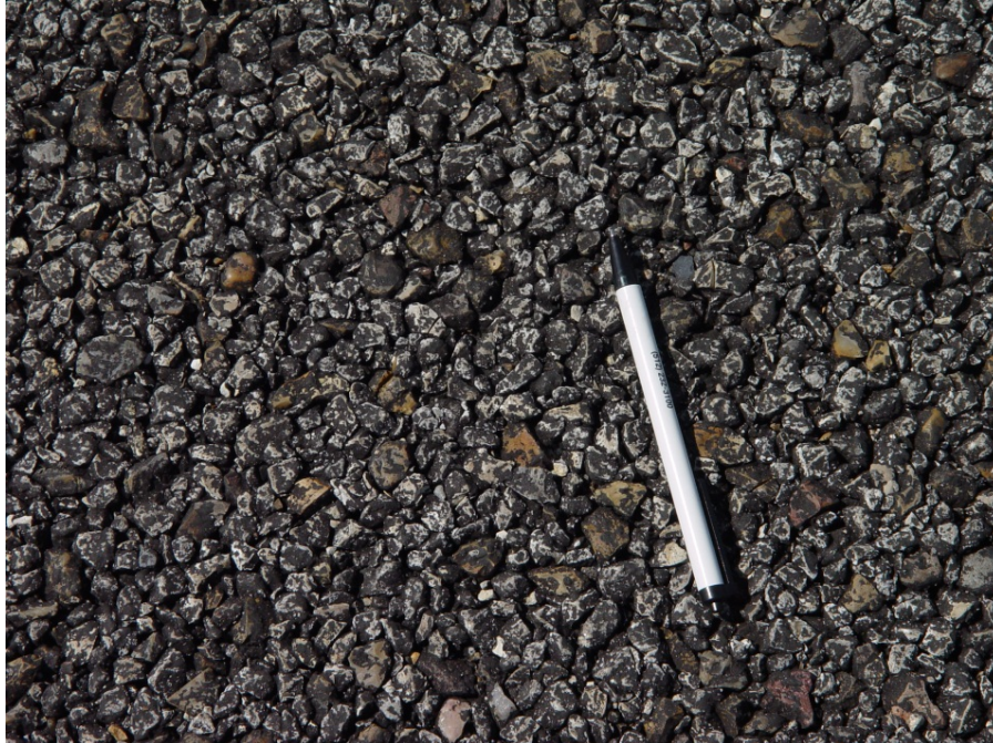
Figure C.45. Detailed View of the PFC Surface on IH-37, Section 14, Corpus Christi.
