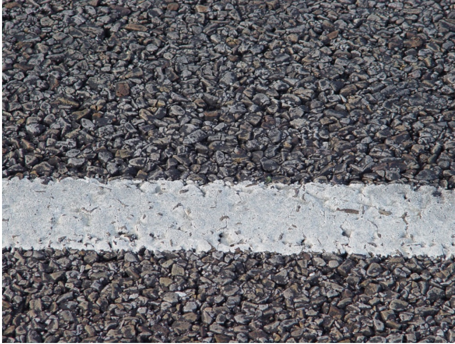
Figure C.17. Detailed View of the PFC Surface on IH-30, Section 4, Subsection 4-6, EB.
