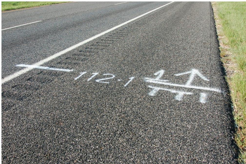
Figure C.40. View of SH 6, Section 112, Northbound.
