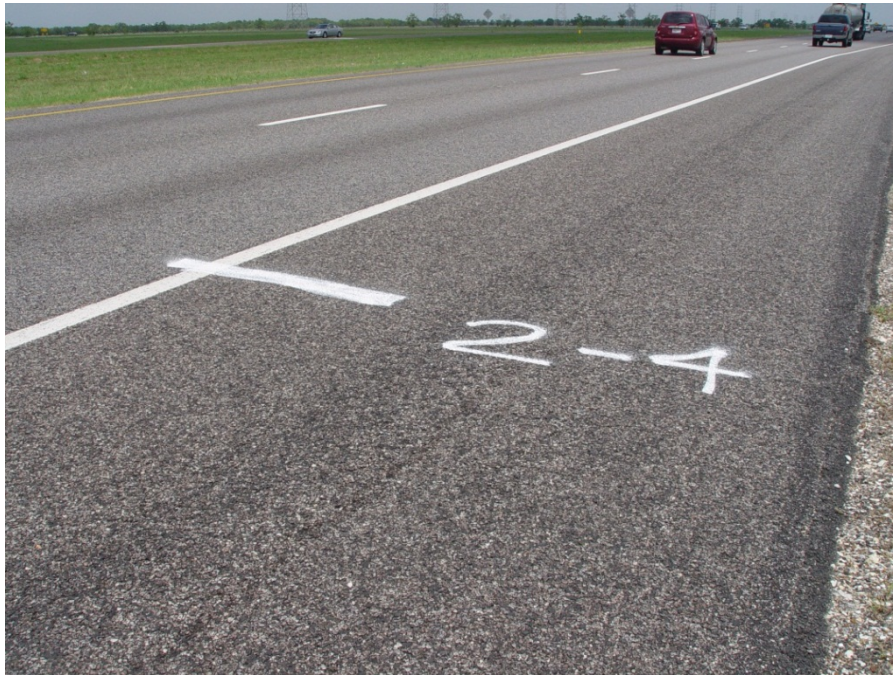
Figure C.7. View of SH 288, Section 2, Subsection 2-4, Northbound.
