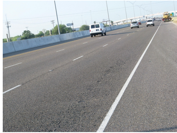
b) Area with Raveling Distress
