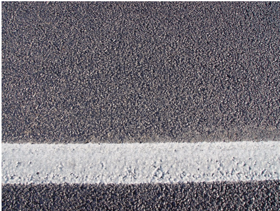
Figure C.24. Detailed View of the PFC Surface on IH 20, Section 6, Subsection 6-1, WB.
