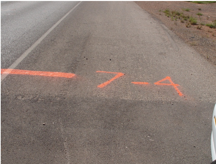
Figure C.28. View of US 83, Section 7, Subsection 7-4, Southbound.
