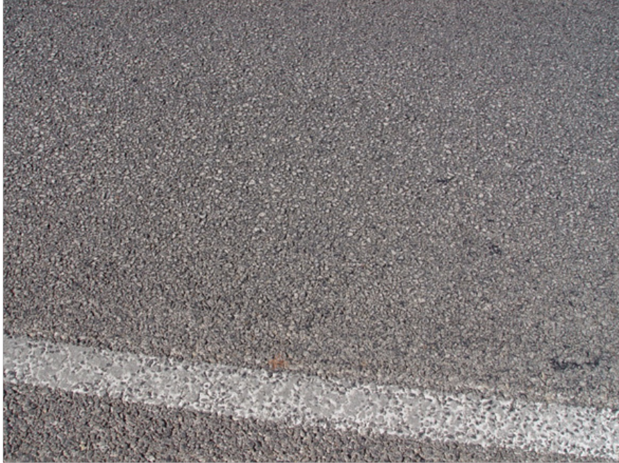
Figure C.27. Detailed View of the PFC Surface on US 83, Section 7, Subsection 7-2, NB.
