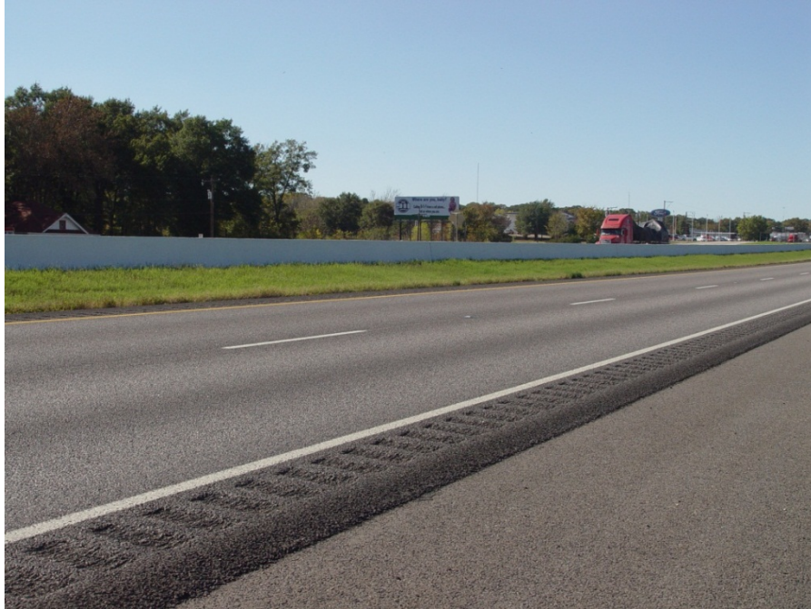
Figure C.53. View of IH 20, Section 19, Subsection 19-4, Westbound.
