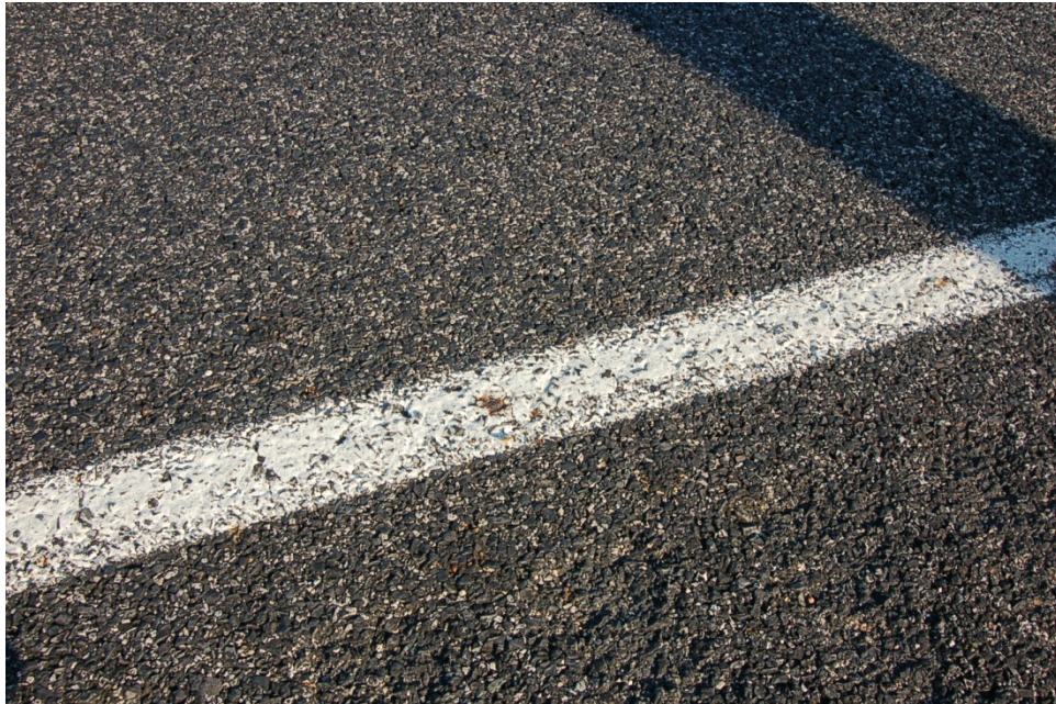
Figure C.42. Detailed View of the PFC Surface on SH 6, Section 112, Southbound.
