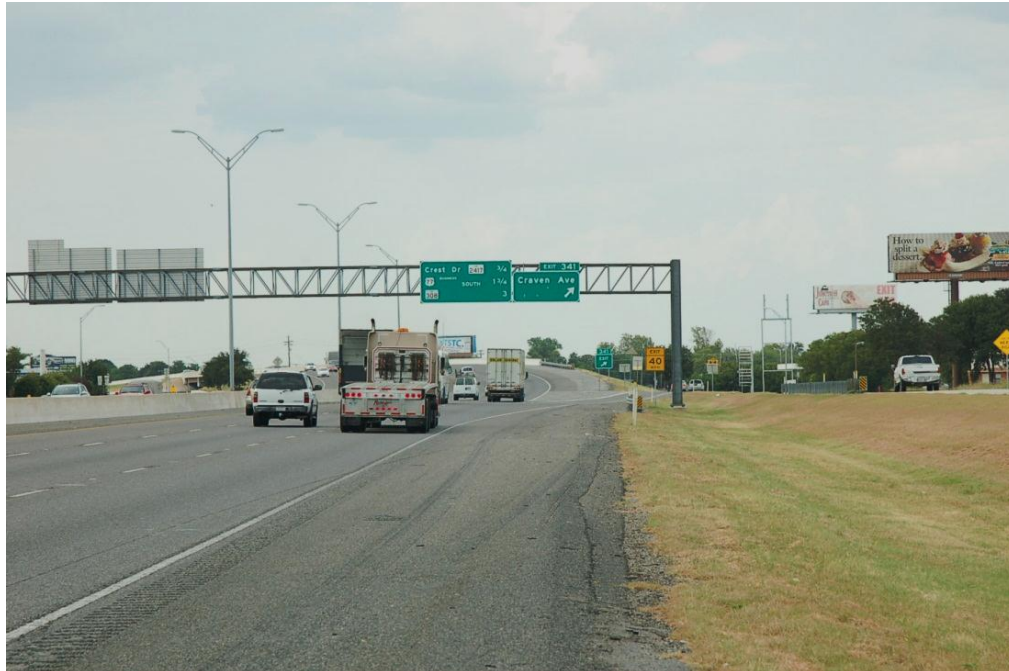
Figure C.50. View of IH 35, Section 17, Northbound (Old PFC).
