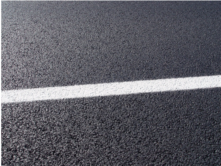
Figure C.57. Detailed View of the PFC Surface on IH 20, Section 20, Subsection 20-3, WB.
