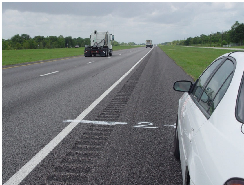
Figure C.6. View of SH 288, Section 2, Southbound.
