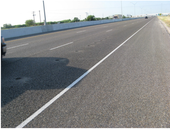
a) Area in Good Condition
