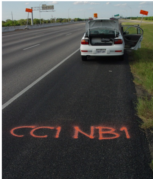
Figure C.46. Views of IH-37, Section 15 (CC1), Northbound.
