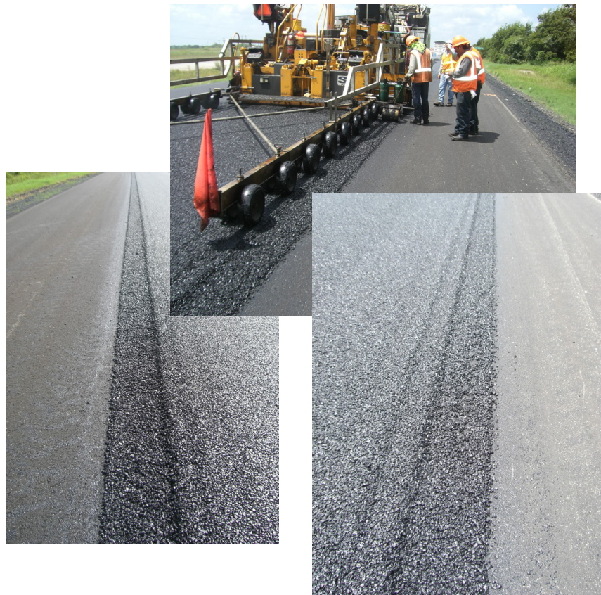
Figure 94. Notched Wedge Joint Construction in PFC.
