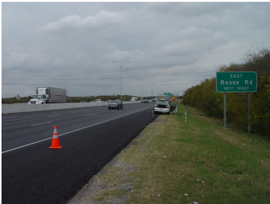
Figure C.34. View of US 281, Section 11, Subsection 12T, Northbound.
