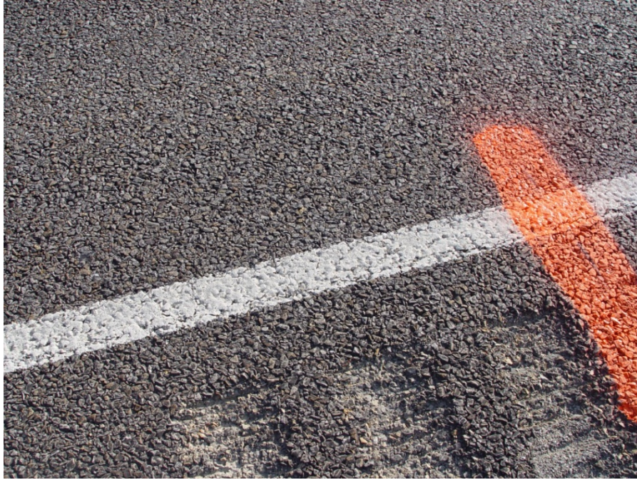
Figure C.15. Detailed View of the PFC Surface on IH-30, Section 4, Subsection 4-1, WB.
