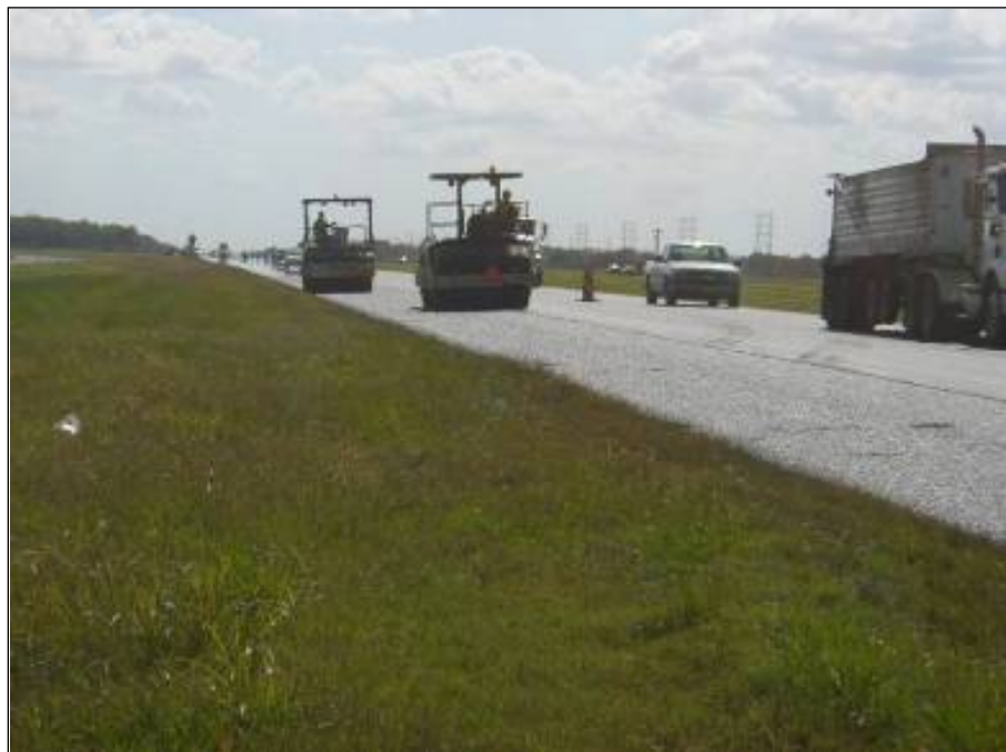
Figure 96. A Single Roller Pass as Allowed in the Houston District (No Roller Back Up Allowed).
