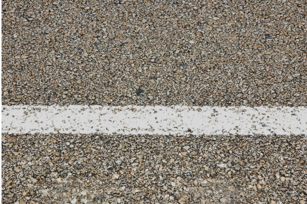
Figure C.32. Detailed View of the PFC Surface on SH 6, Waco.
