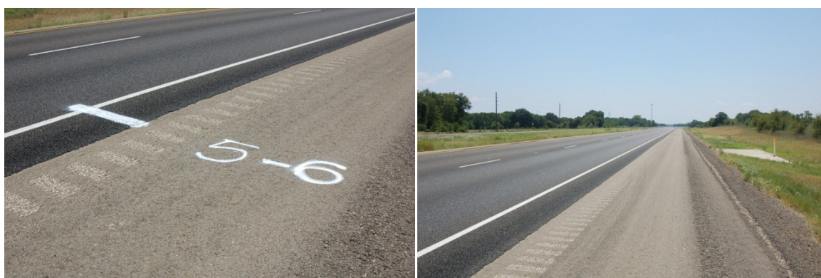
Figure C.21. Views of SH 6, Section 5, Southbound.
