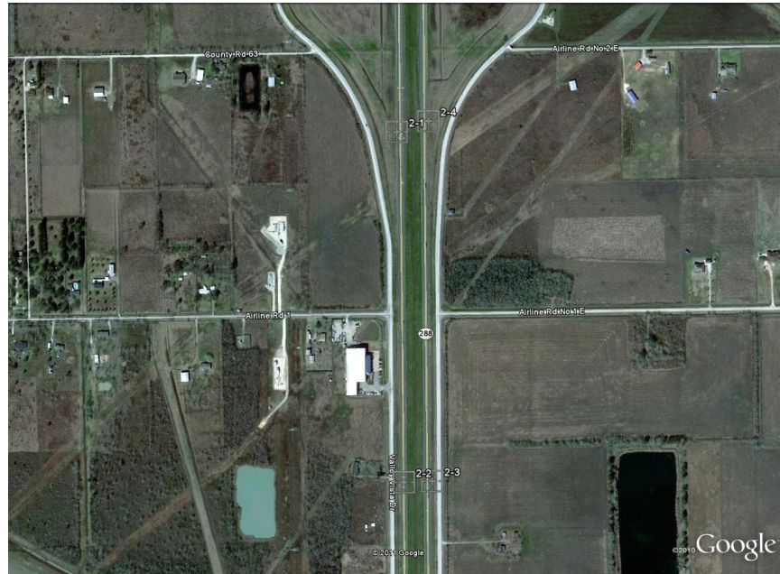
Figure C.5. Section 2 on SH 288, Houston.
