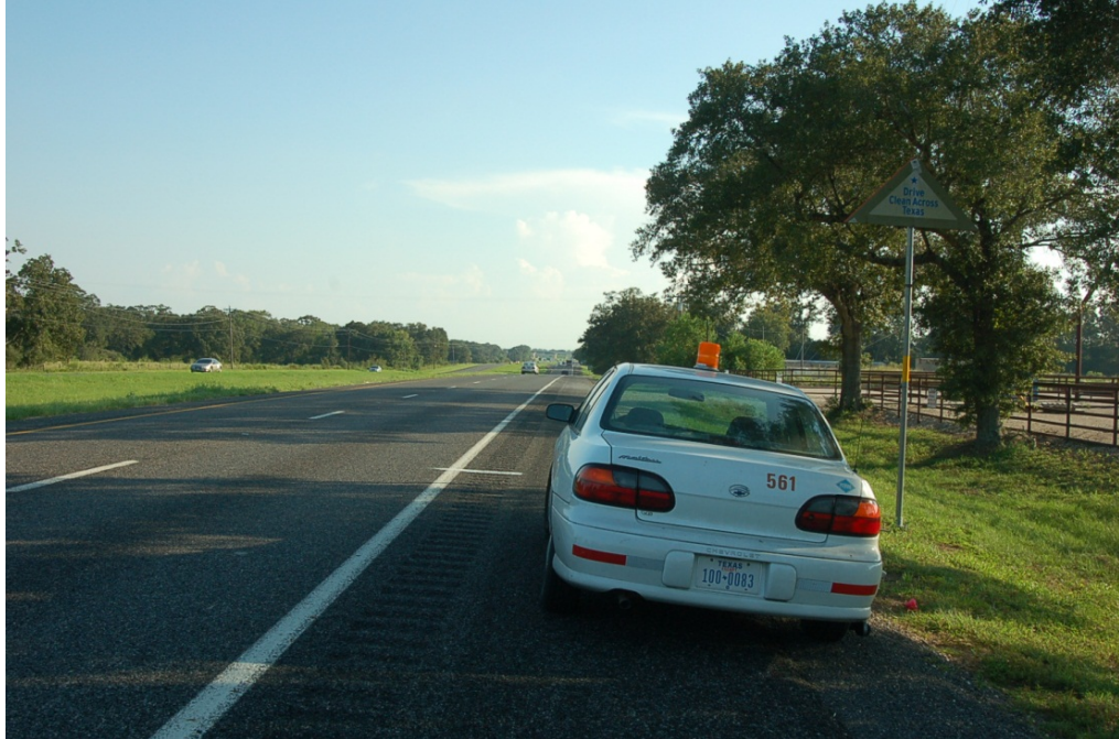
Figure C.41. View of SH 6, Section 112, Southbound.
