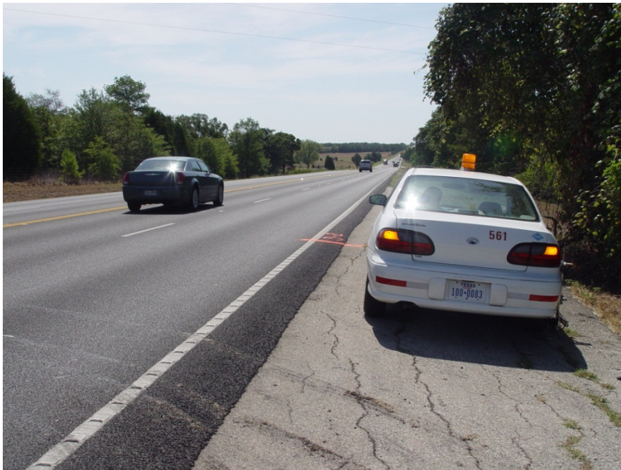
Figure C.11. View of US 290, Section 3, Subsection 3-3, Eastbound.
