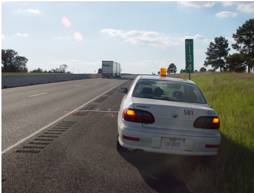
Figure C.14. View of IH-30, Section 4, Subsection 4-1, Westbound.
