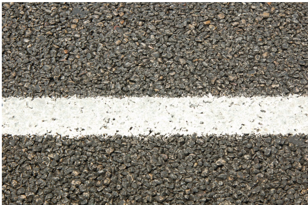
Figure C.20. Detailed View of the PFC Surface on SH 6, Section 5, Subsection 5-1, NB.
