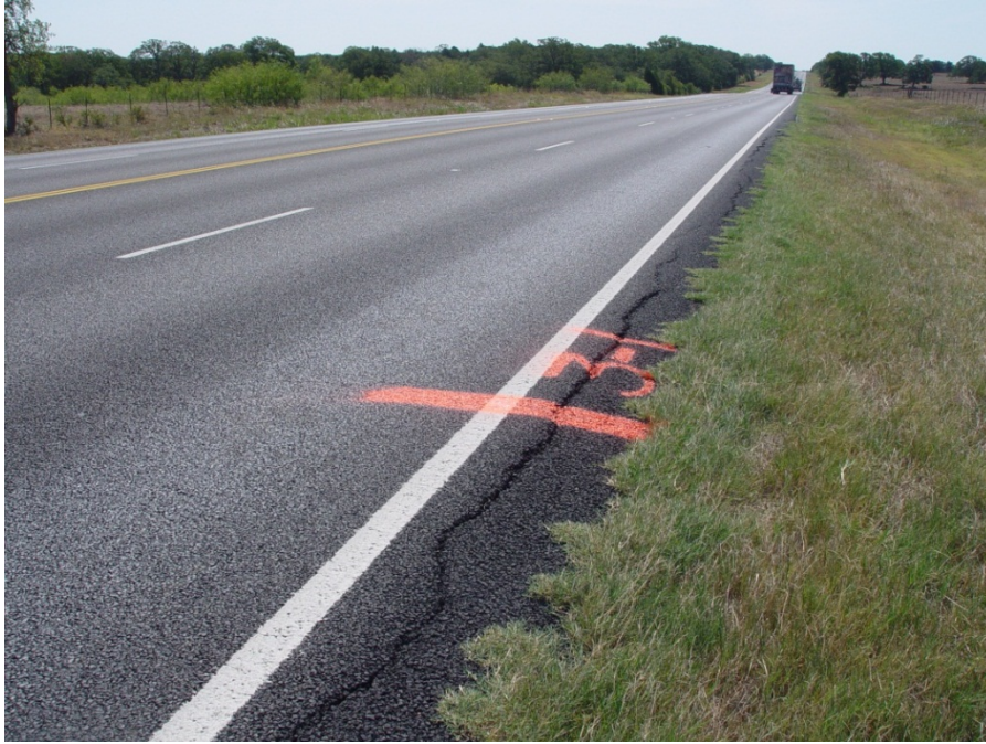
Figure C.10. View of US 290, Section 3, Subsection 3-1, Eastbound.
