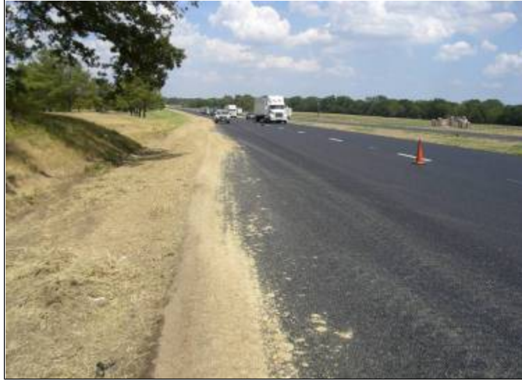
Figure 91. Edge Clearing that Can Cause Clogging of PFC Restricting Lateral Water Flow.
