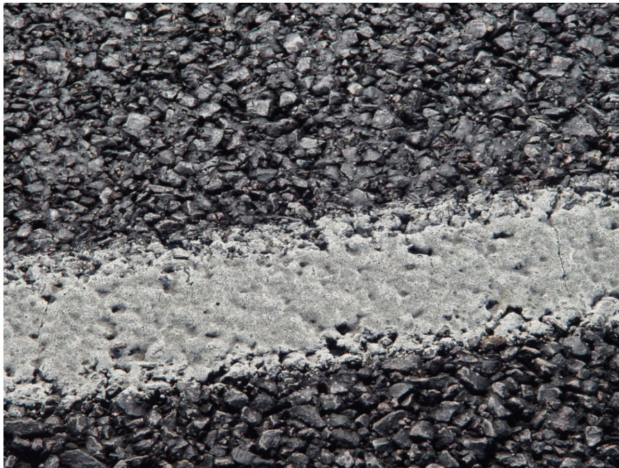
Figure C.54. Detailed View of the PFC Surface on IH 20, Section 19, Subsection 19-5, WB.
