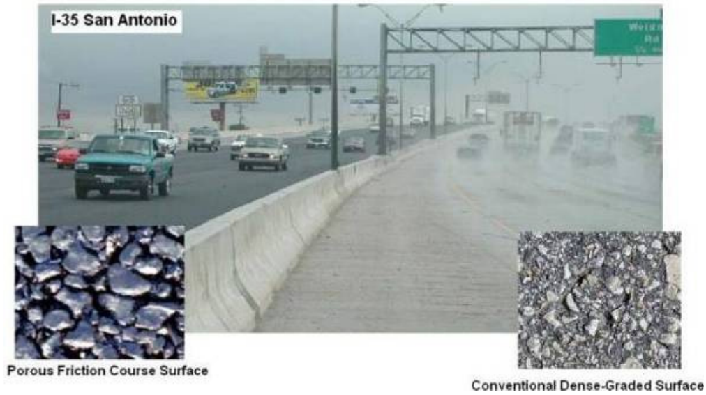
Figure 83. PFCs in Urban Areas to Reduce Splash and Spray (San Antonio IH 35).
