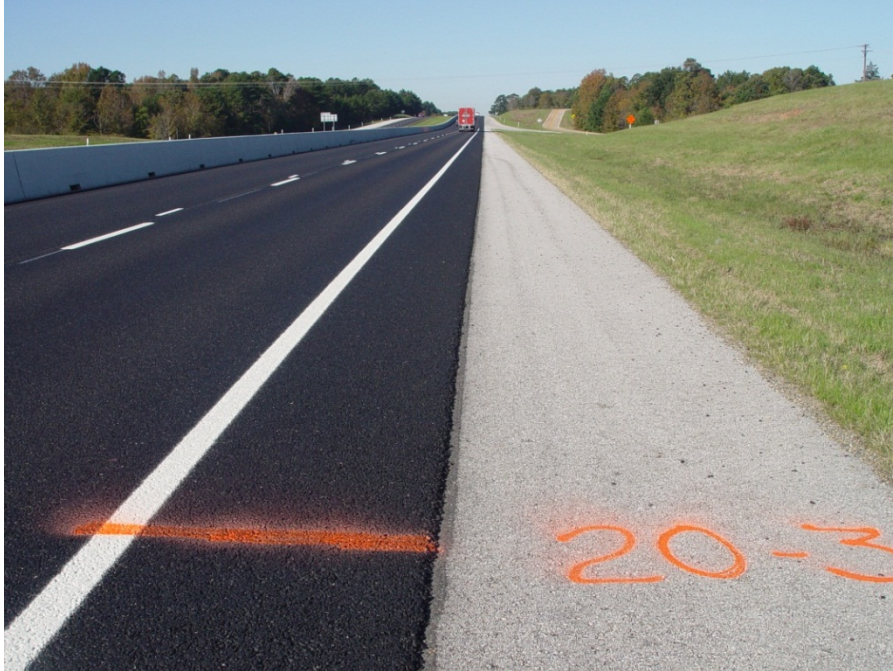
Figure C.58. View of IH 20, Section 20, Subsection 20-3, Westbound.
