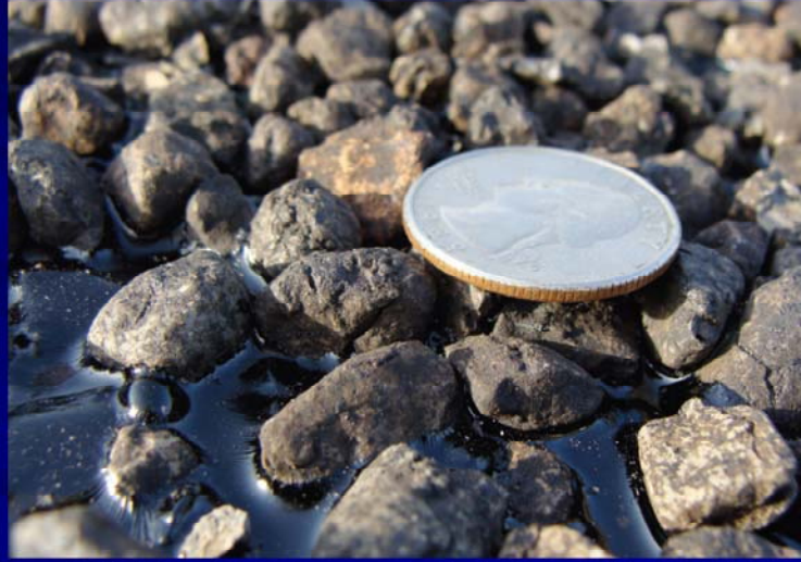
Figure 4-12. Wheel Path Aggregate Embedment Slightly Higher than Usually Desired after a Day or Two of Traffic.
