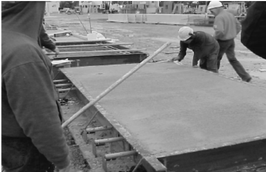
(a) Precast PCC panel
