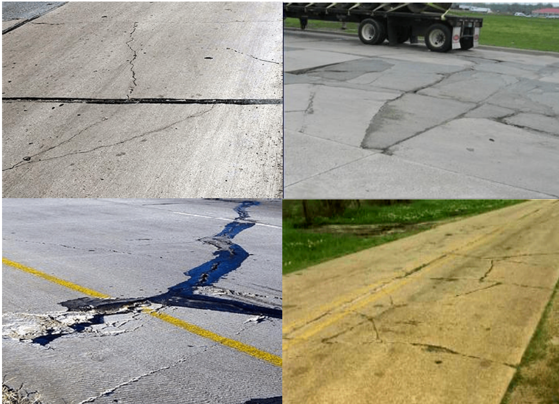
Figure 17 Shattered Slabs.
