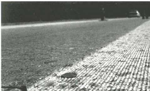
Figure 62 Diamond Grinding (21).
