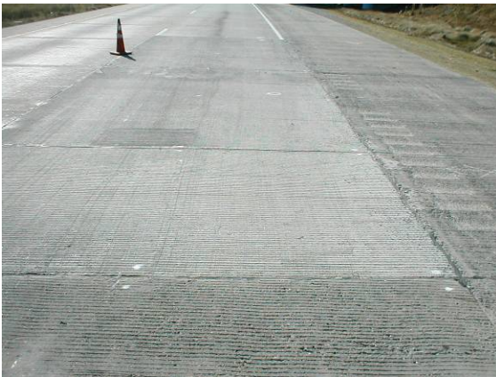
Newly Patched Section
