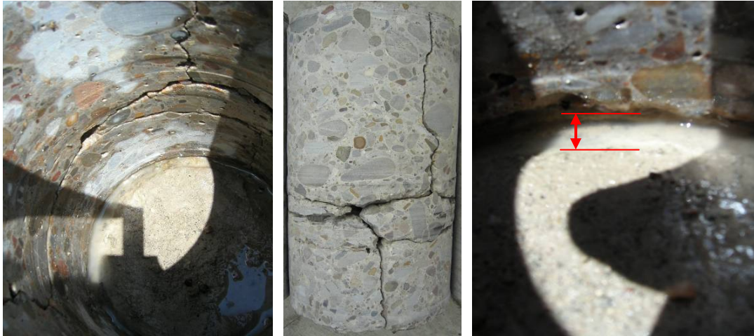
Figure 49 Coring in Poor Condition Section.
