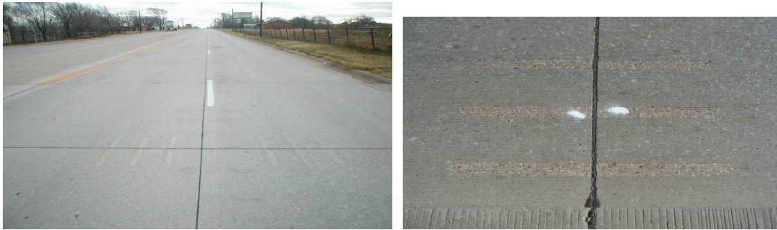
Figure 44 Repaired Section Using DBR and DG in Quanah.
