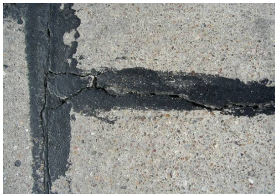
Crack and Deteriorated Joint Sealing in Poor Condition Section
