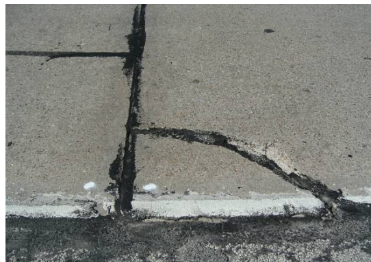
Crack and Deteriorated Joint Sealing in Poor Condition Section
