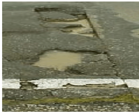
Figure 19 Reflection Failure.
