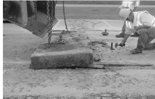
(b) Slab removal
