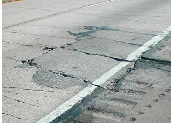
Figure 13 Patch Deterioration.
