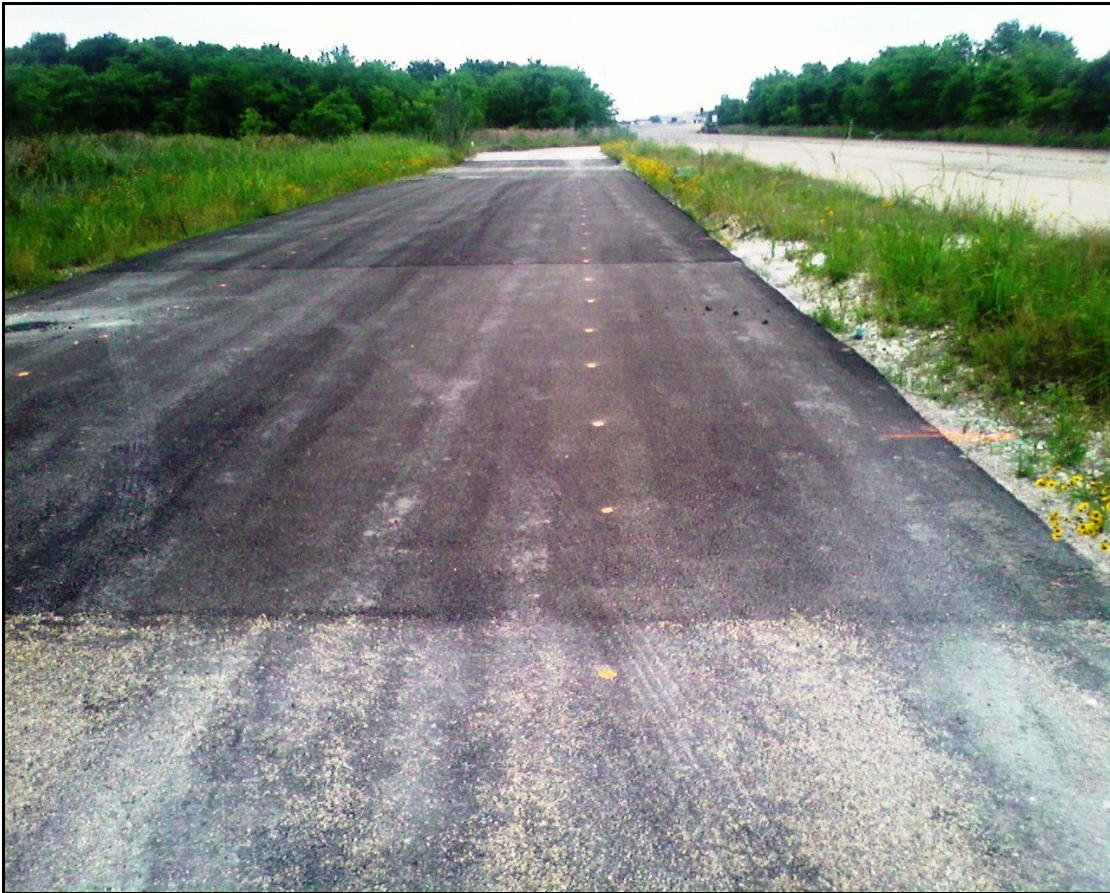
Figure 6-3. Picture of Test Track after Construction.
