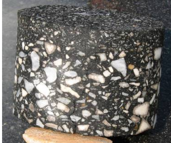
Figure 4-29. Evidence of Bottom-Up Fatigue Cracking.
