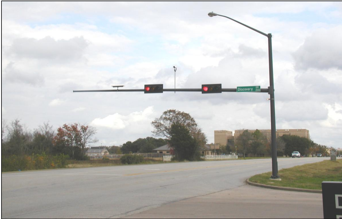
Figure 8. F.M. 60/Discovery Drive Intersection in College Station.
