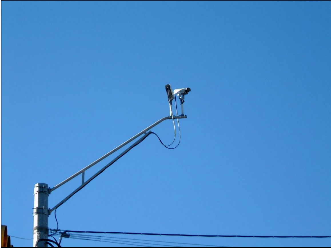
Figure 5. S.H. 105/Walden Intersection near Conroe in the Houston District.
