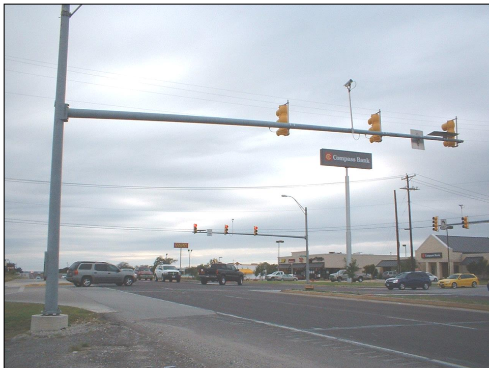
Figure 4. Ft. Worth District VIVDS High-Speed Intersection Installation.
