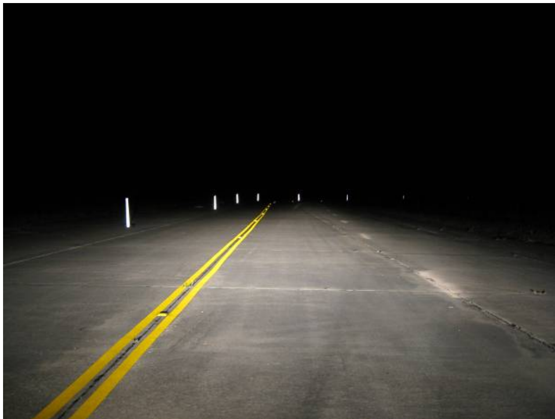
Figure 6. Photo of Curve 1 with Fully-ReflectORIZED Post-Mounted Delineators.
