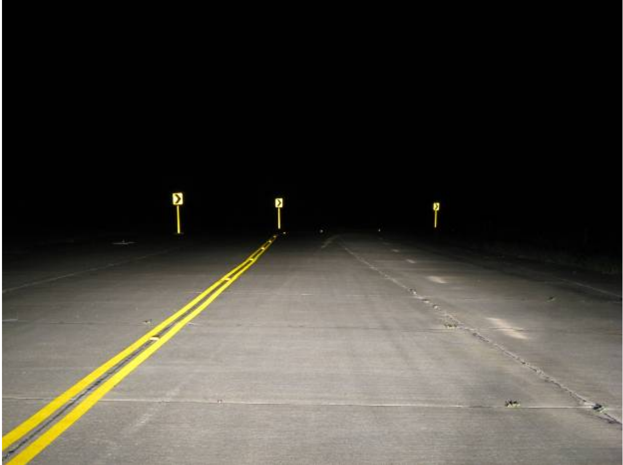
Figure 9. Chevron Signs with Fully-Reflectorized Posts on Curve 1.
