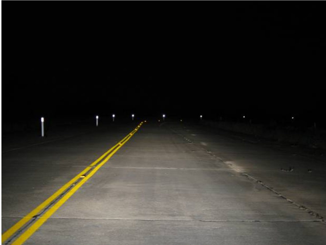
Figure 7. Photo of Curve 2 with Dot-ReflectORIZED Post-Mounted Delineators.
