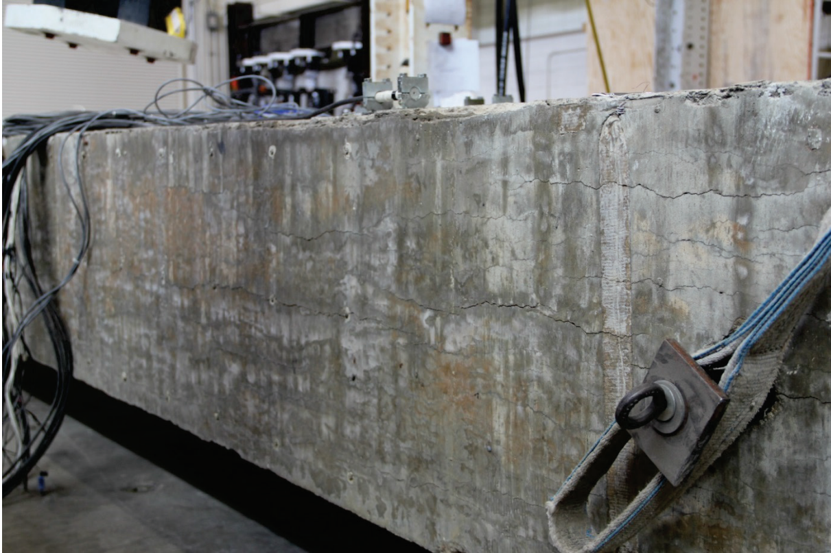
Figure 4-3. Cracking of Specimen #12 prior to Structural Load Testing.
