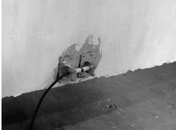
Figure 4-11. KM Gage Installation prior to Testing.
