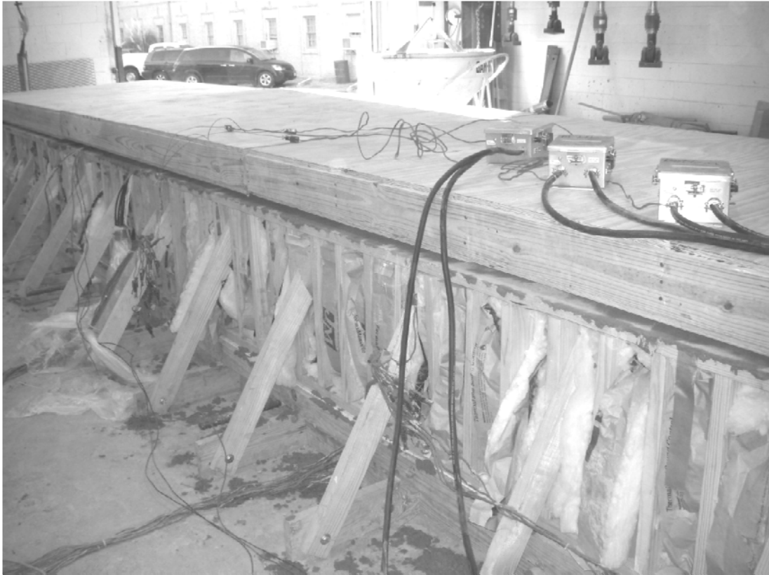
Figure 2-22. Insulated Form with ERW Power Supplies on Top.
