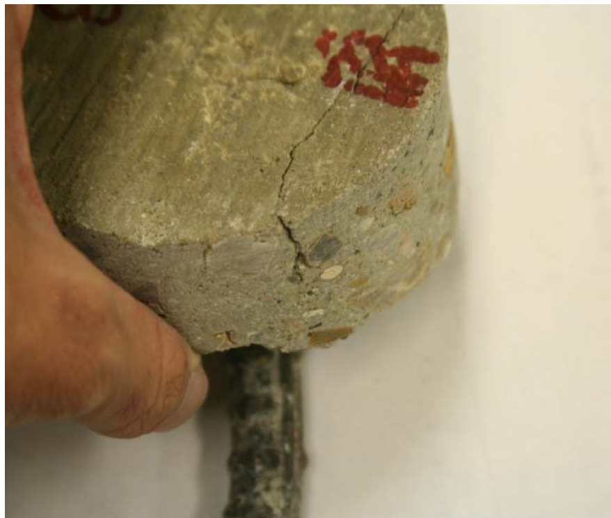
Figure 3-30. Core Extracted above Hoop with Surface Cracking.
