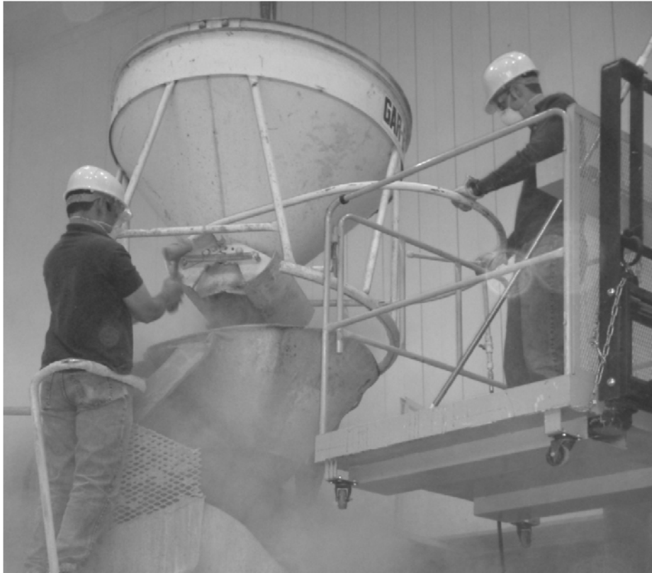
Figure 2-19. Dumping Cement into the Mixer.
