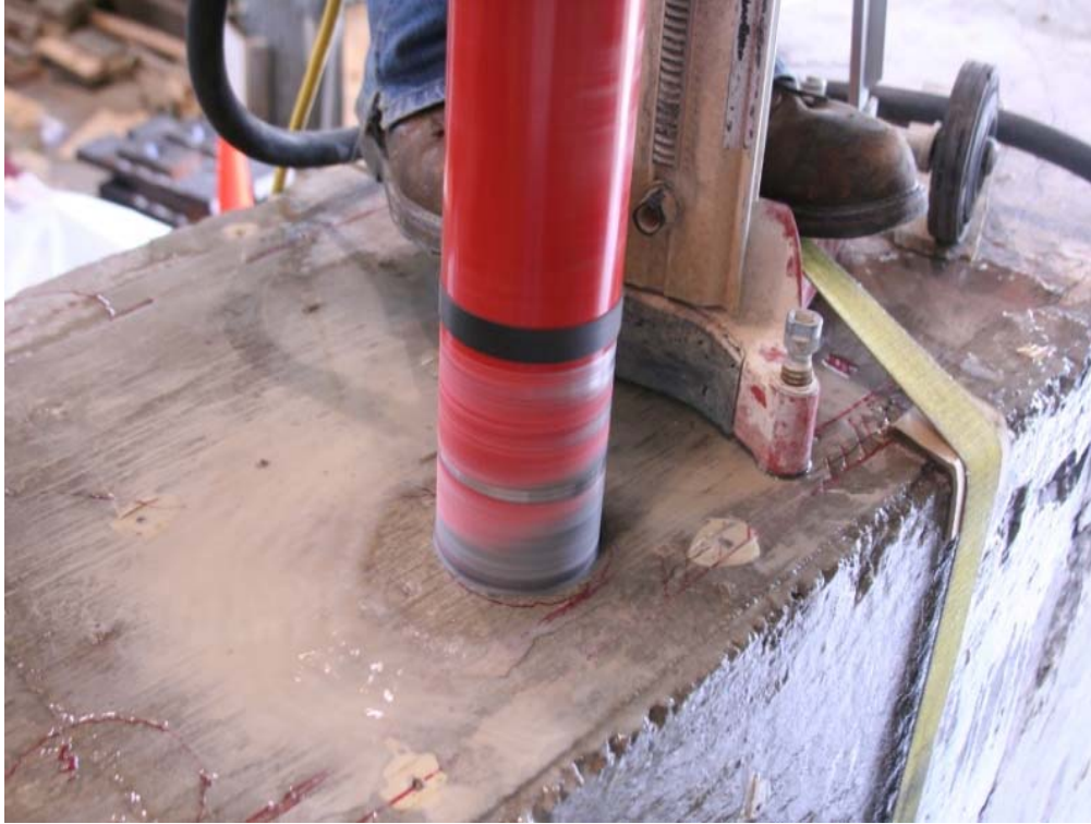
Figure 3-27. Coring Machine Attached to Beam.
