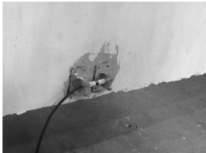
Figure 5-8. KM Gage Installation prior to Testing.
