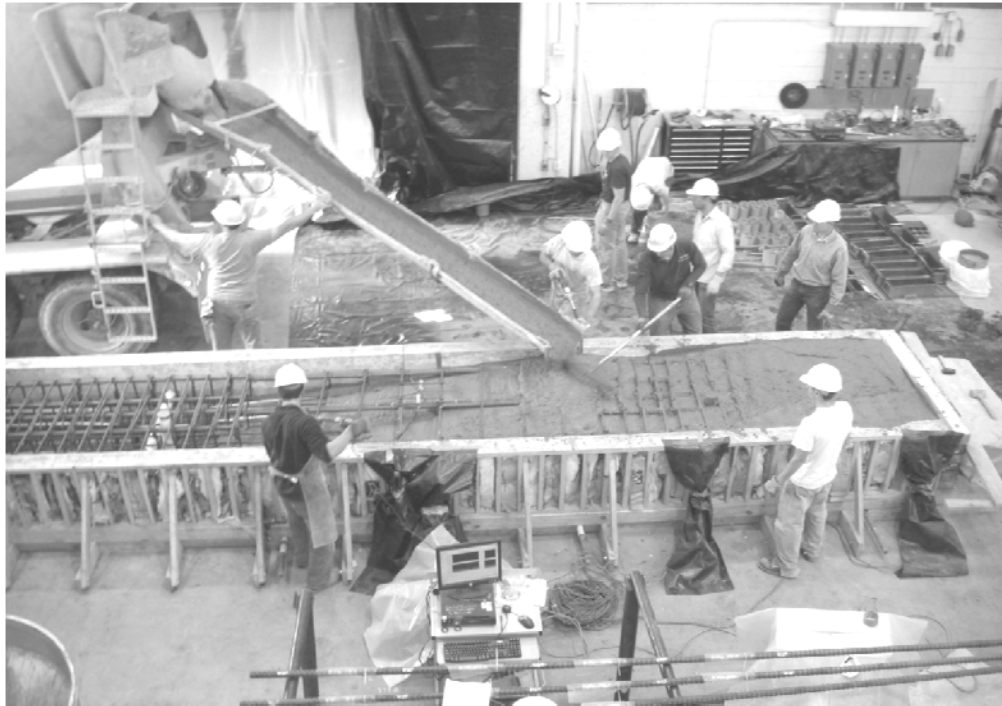
Figure 2-21. Pouring Concrete in the Form.
