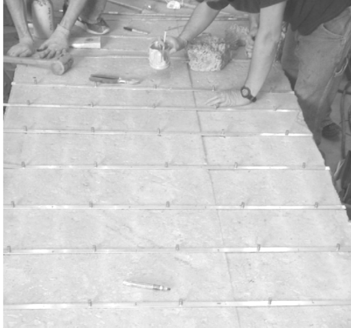
Figure 2-26. DEMEC Installation on the LSC Specimen's Large Face 1.
