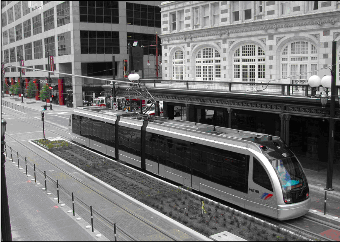
Figure 2. Houston METRORail, Houston, Texas.
