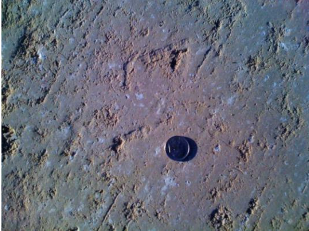
Figure 18. Waco, US 84, Eco-Prime. Relatively Impermeable.
