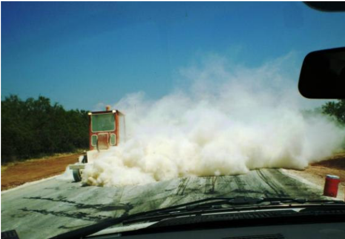
Figure 23. Abilene, FM 1235, AEP. Aggressive Brooming.
