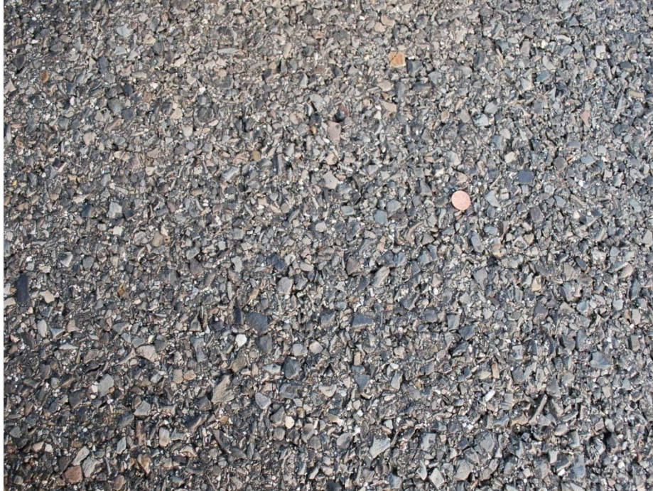
Figure B5. SMA-C Mixture on Wheelpath of IH 20 in Atlanta District.
