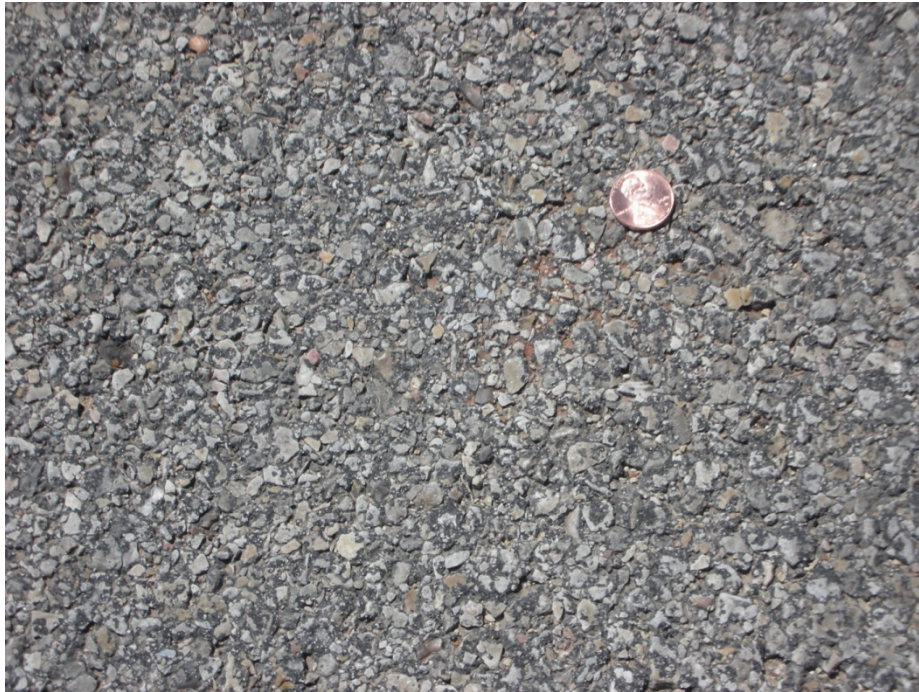
Figure B12. Superpave Mixture on Shoulder of IH 20 in Abilene.
