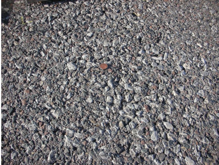
Figure B3. CMHB Mixture on Wheelpath of US 87 in Lubbock.
