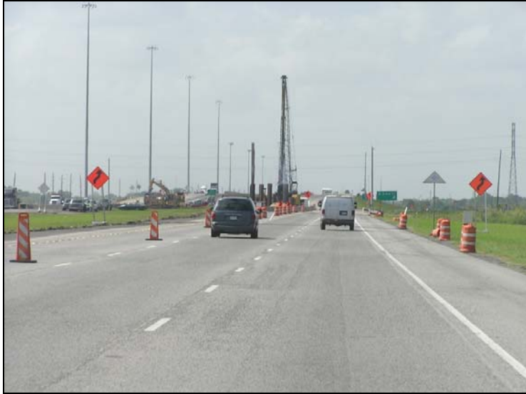
Figure A-13. Street View of SH 288 Northbound Lane Closure.
