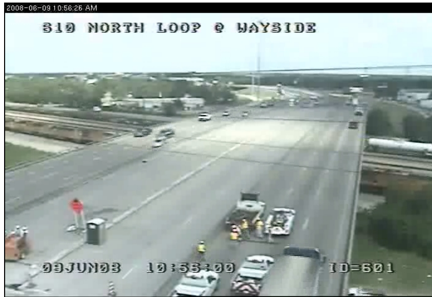
Figure A-2. Site 1 Work Activity.
