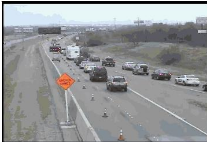
Figure A-9. Left Lane Closure for Site 4.
