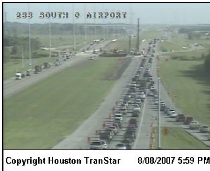
Figure A-12. SH 288 Construction in Final Stages.
